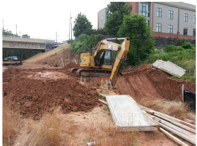
Gunby Street drainage and ramp installation activity adjacent and away from soil cap.
