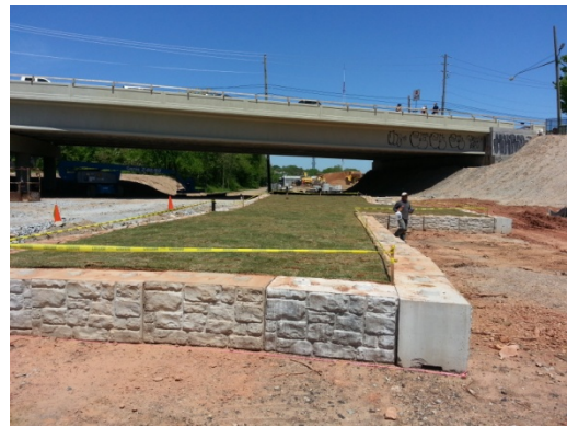
View looking north of final soil-vegetative cap on the NW corner of 670 DeKalb Avenue
