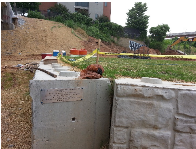
View east from Beltline property. Corners are holding soil well and vegetation is healthy.
