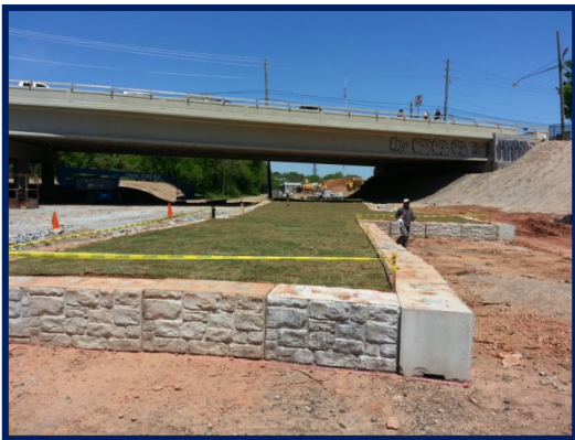
View looking north of final soil-vegetative cap on the NW corner of 670 DeKalb Avenue.
