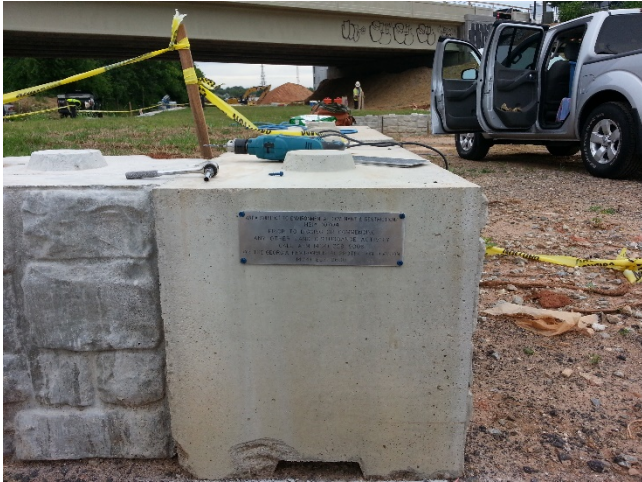
View north from SE Corner, vegetation cover is intact. Surface is used by contractors
