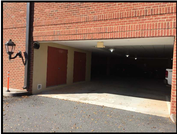
3. View of parking deck entrance at south wall of building.
