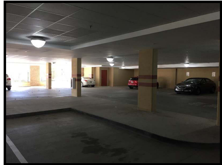
4. View of parking deck interior facing south to deck exit
