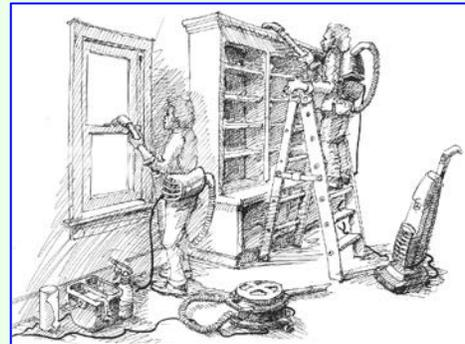
☀ Wash the windowsills and window troughs in the work area with general purpose cleaner and damp cloths. Use a wet cleaning method that keeps the wastewater separate from the rinse water. Georgia requires that window troughs be cleaned and reach cleaning verification requirements.
