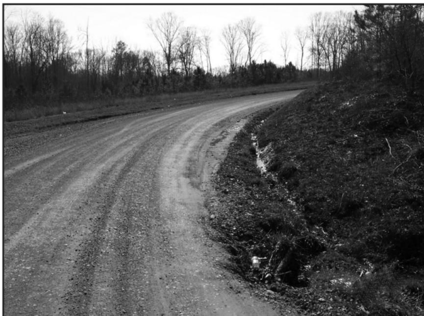
Problem: culvert is blocked with debris; ditch grade too steep.
