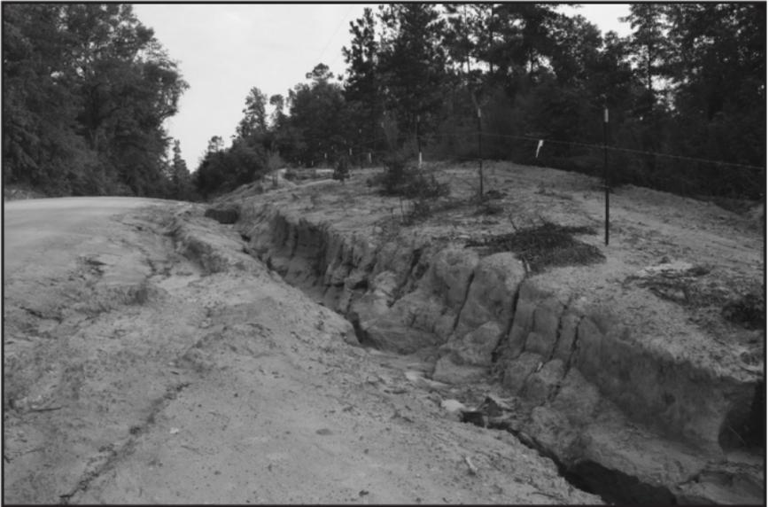
Eroded ditch in need of maintenance; tremendous source of sediment to state waters.
