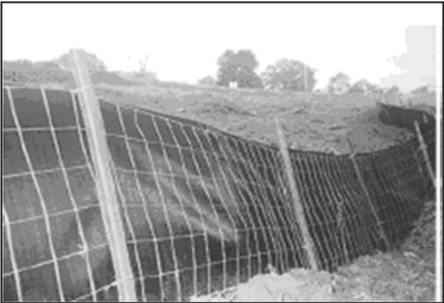
Example of type "C" sediment barrier silt fence (Sd1-C). Note that the fence is slightly angled into the direction of runoff.
