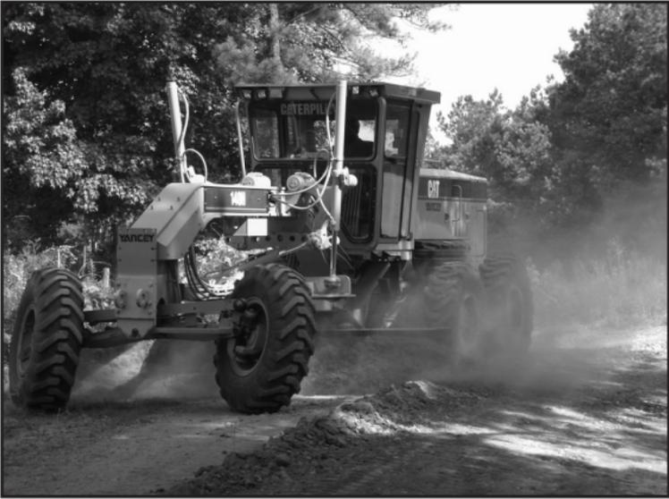
Re-shaping crown step 1: cutting road surface.
