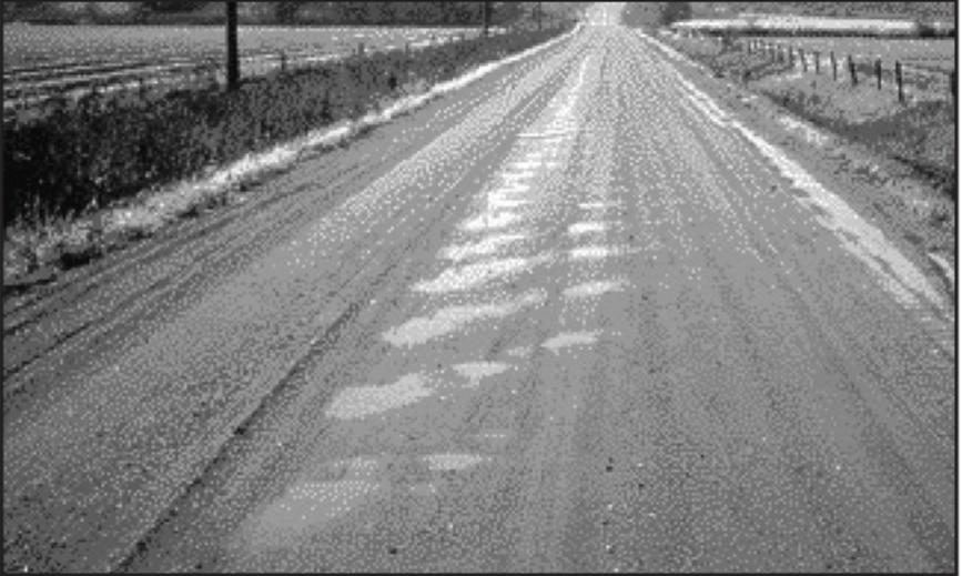
This distortion was cut into the road surface by operating motor grader too fast. The angle of depressions matches the angle of the moldboard.
