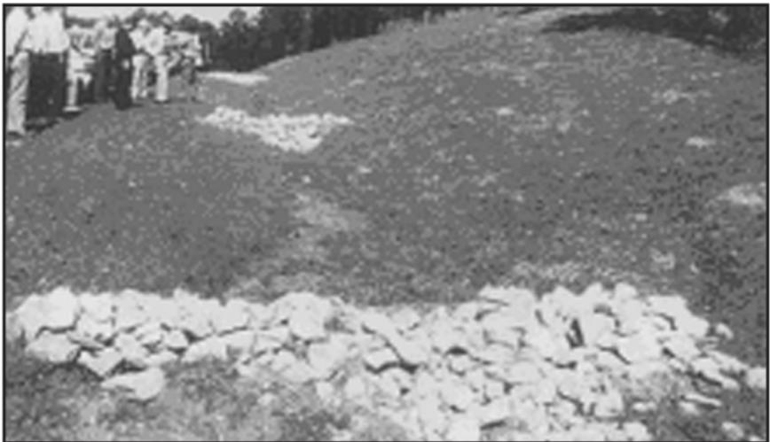
Example of check dams (Cd) in concentrated ditch flow.
