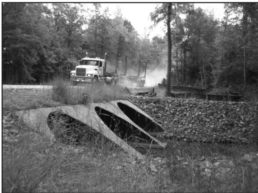
Example of rock filter dam (Rd) installed at drainage ditch outlet to live stream.
