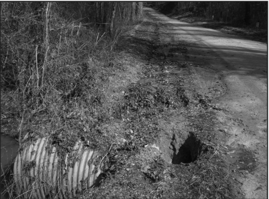
**Problem:** water erosion around pipe; poor installation with fill.
