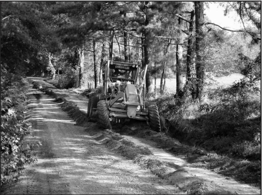
Example of “pulling” ditch and re-establishing crown.
