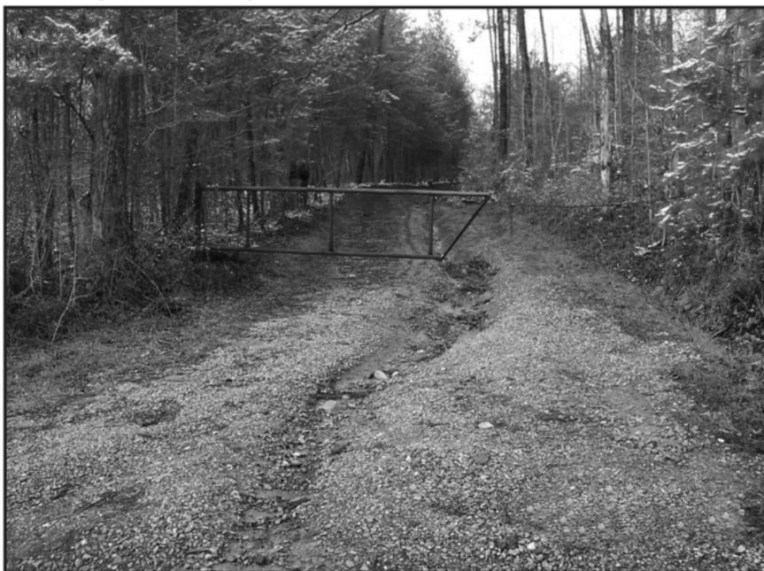
Inadequate surface water control and crowning contributed to this forest road rut.
