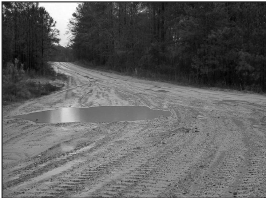
Poor drainage causing weak sub-grade and road surface from vehicle weights during “dry” periods.
