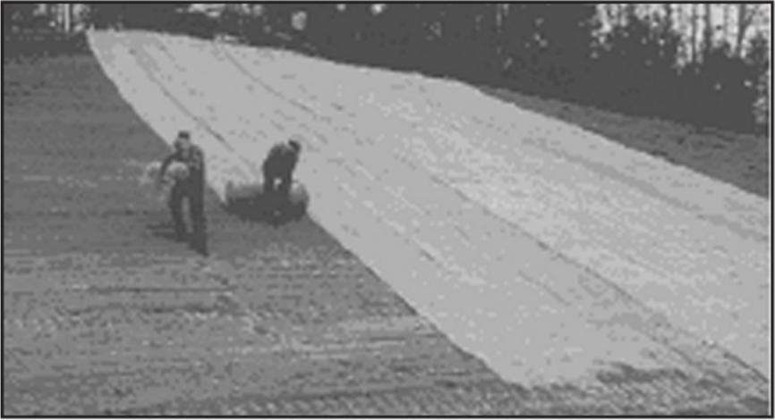
Example of installation of jute (wood fiber) matting, erosion control blanket/matting (Mb).
