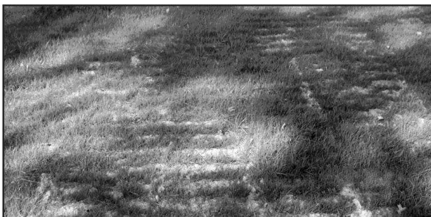
Example of 1-month old tracking with grass cover establishment for slope stabilization.
