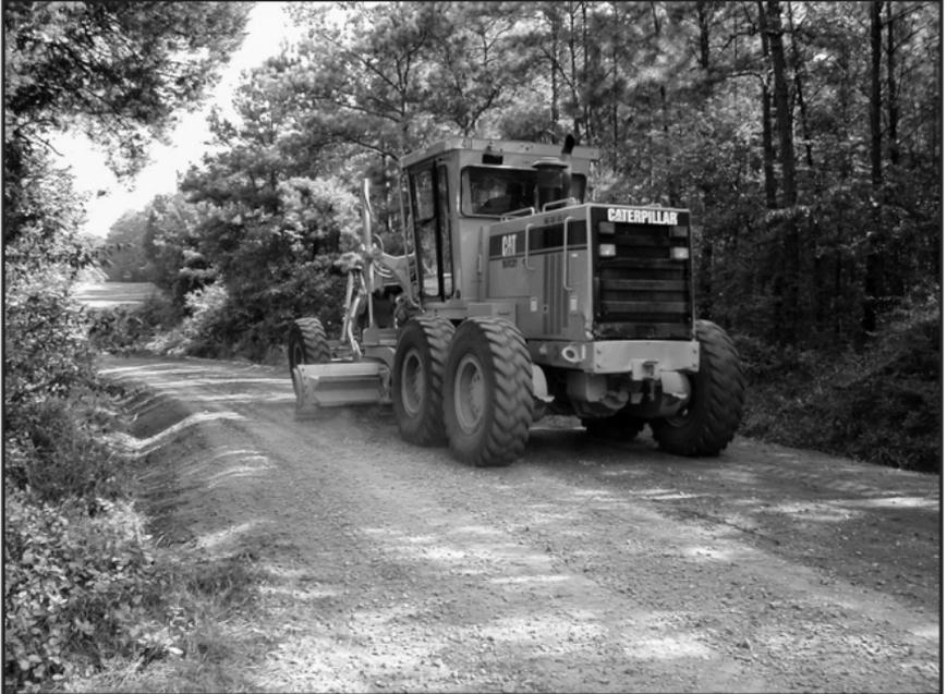
Blading to move surface materials; note slight tilt of front wheels.
