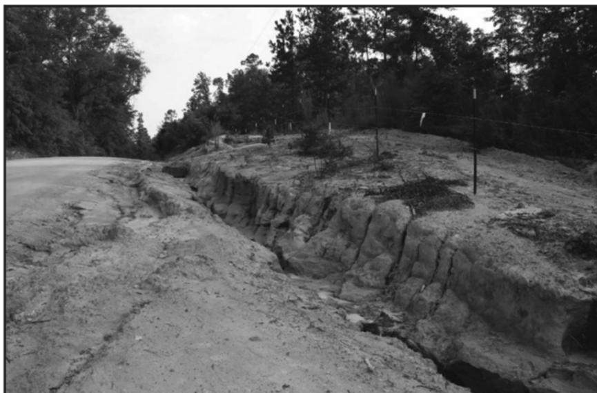
Before Implementation: Eroding road surface, road banks, and ditches
