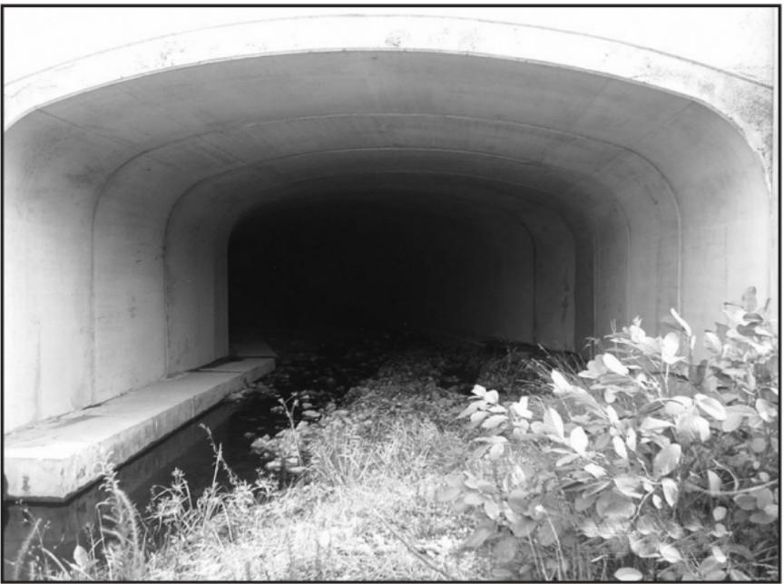
Example of bottomless culvert; note natural bottom material remains exposed.
