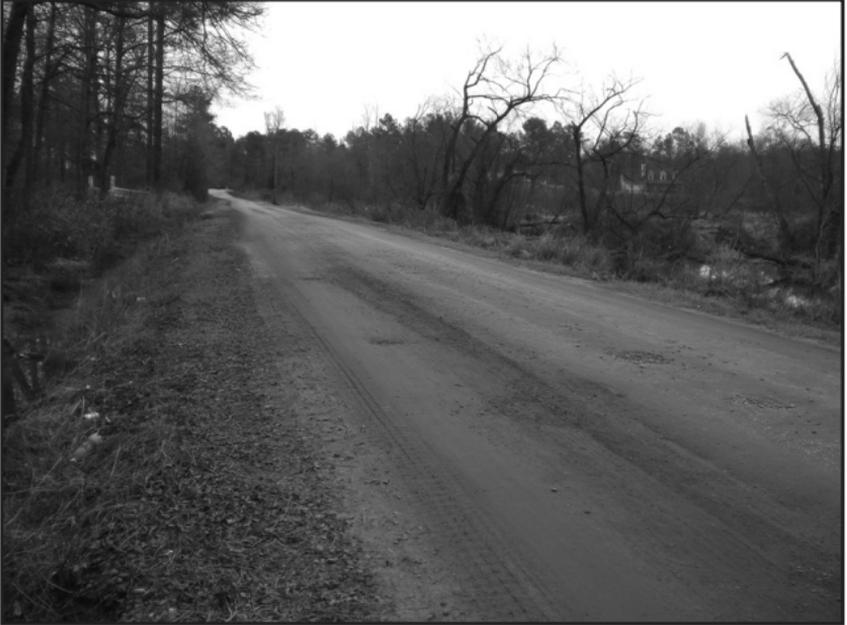
Unpaved road adjacent to wetland (right shoulder); note vegetated shoulder, banks and ditch to trap sediment.
