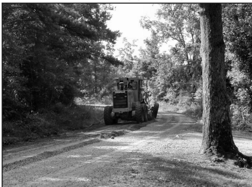
Blading against traffic flow can reduce surface distortions.
