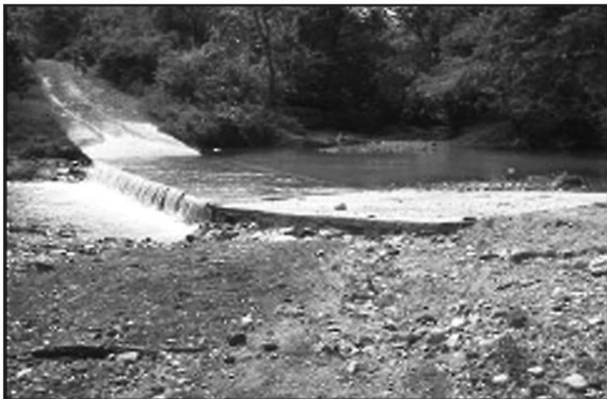
Example of concrete low-water crossing; note downstream edge is protected from scouring with riprap or gabions.
