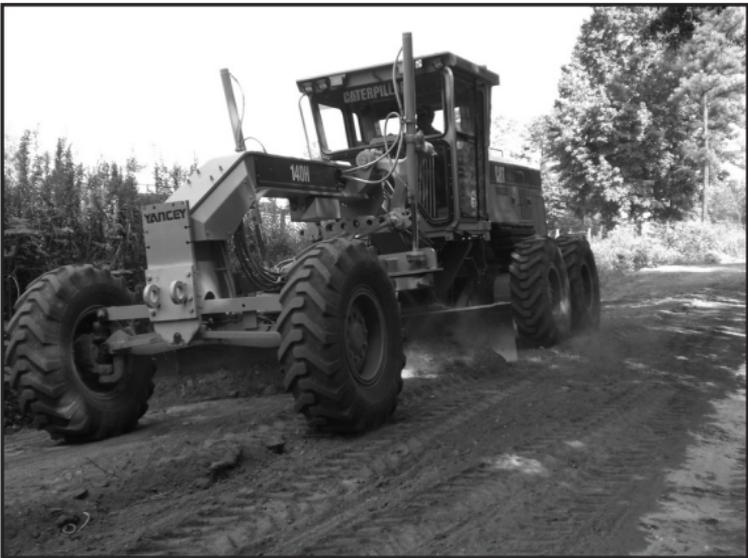
Re-shaping crown step 2: re-distributing road surface.
