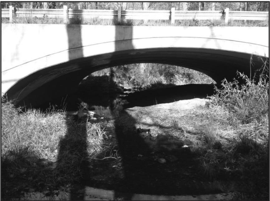
Example of low arch bridge; note span is outside of stream channel.
