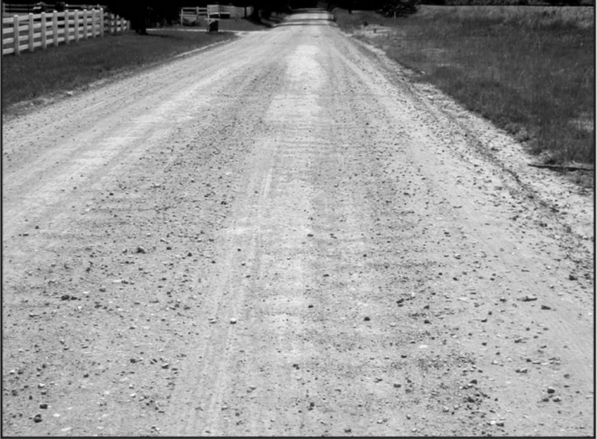
Road surface ravelling; coarse aggregates worn away by traffic.
