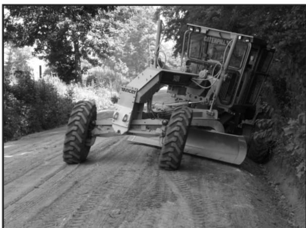
Using wheel for “shaping and tamping” ditch; creates a “roll” or “rounded U” shape ditch.
