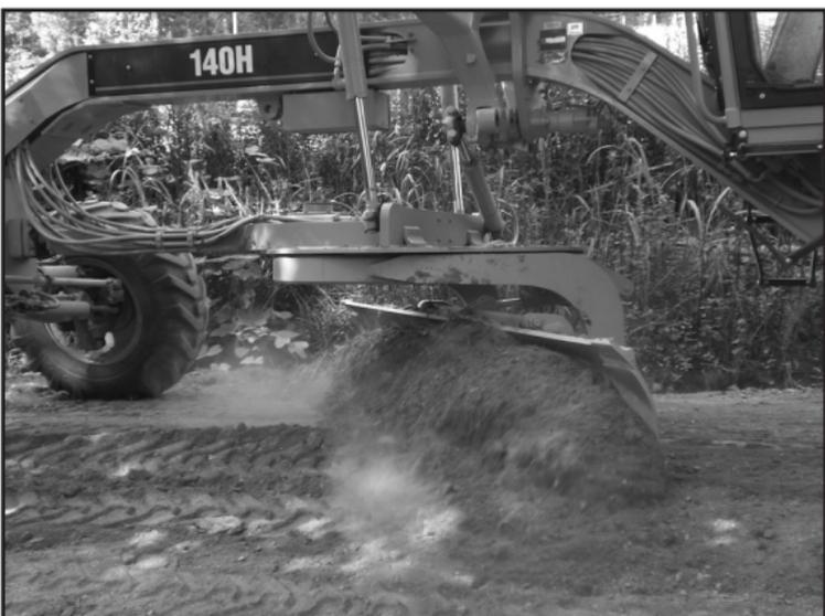
Re-shaping crown step 3: re-mixing road surface.
