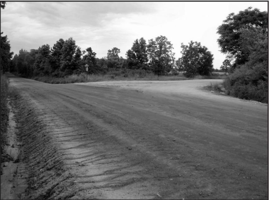
Lignin sulfate application; treated area “darker” than side road.
