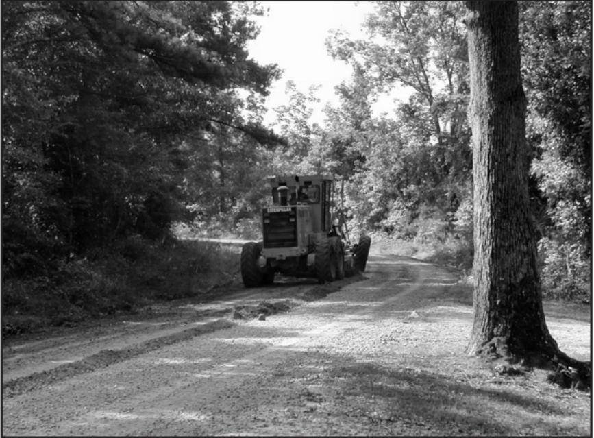
Note tilt of front wheels and grading against traffic flow.
