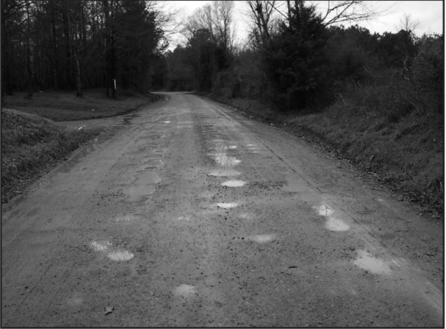
This road section suggests poor road drainage.
