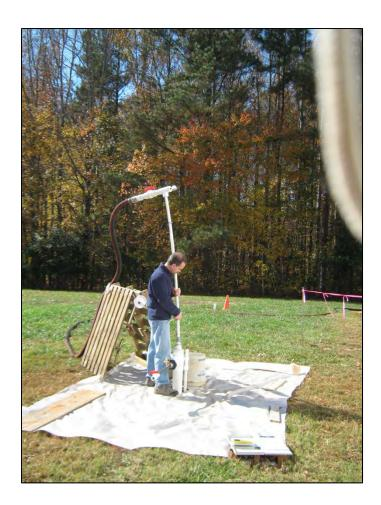
An operator inserts the slurp tube through the top port of the MP-2 wellhead. The flexible hose runs back to the manifold at the MPE trailer.
