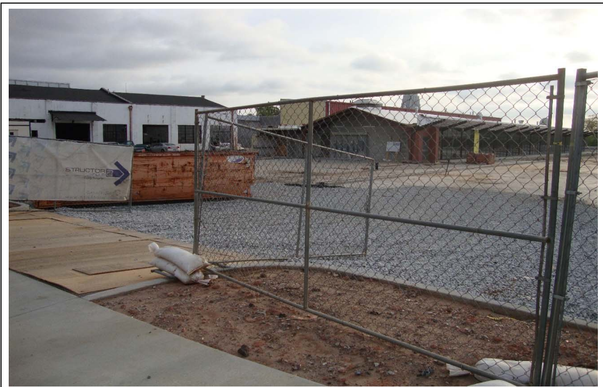
Photo 2. View northeast across underground detention vault area from Howell Mill Road. Note proposed restaurant concrete pad and remnant original building in background.
