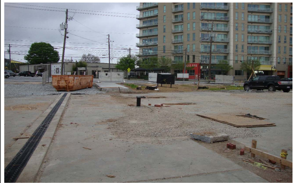
Photo 1. View west across property from northeast corner of existing building. Note footing excavations and trench drain in foreground with gravel cover over underground detention vault and soil cover over future landscaped area in background.
