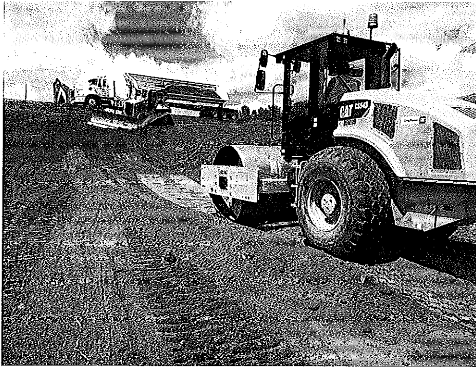
Compaction of the ash material was achieved using a vibratory smooth drum roller.
