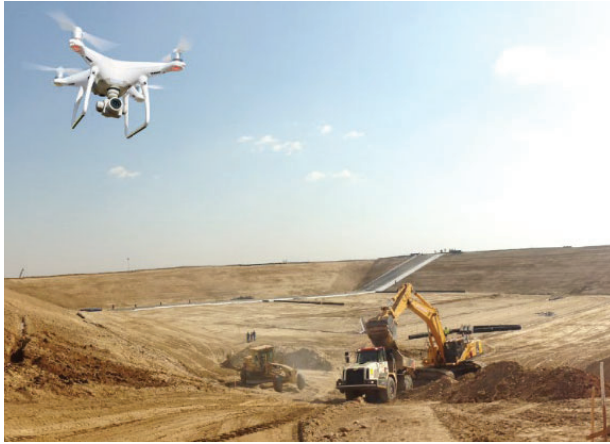
Exhibit 2. UAV Survey and Portable Ground Control Tile
