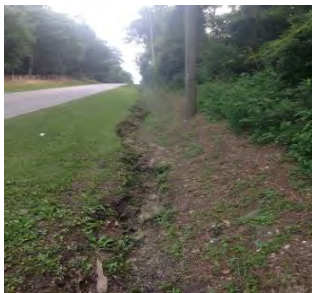
Ditches downstream of Thomas University- recommended BMP-rocklay infrastructure within ditches to alleviate the erosion and collapse. The City Thomasville Engineers were alerted to this issue and are addressing.
