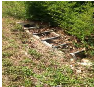
Collapse and blocked storm drain downstream of Thomas University 25 yards past above referenced issue opposite side of street- recommended – address and fix collapse, clear out plugged storm drain. The City Thomasville Engineers were aware of collapse due to working in the area, and send team to clear drain the following day. .
