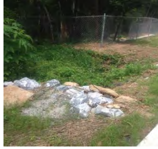
Residential area on Tuxedo drive to alleviate storm water runoff. Installation of this BMP was not at correct slope level and caused more flooding in the home owner's property as well and the street. City of Thomasville Engineers were aware of the issue and were addressing.
