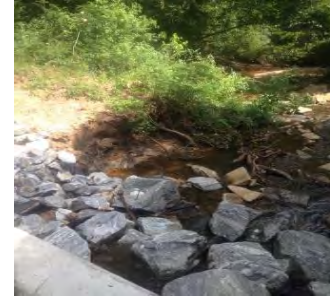
Residential area on Tuxedo drive to alleviate storm water runoff. Installation of this BMP was not at correct slope level and caused more flooding in the home owner's property as well and the street. City of Thomasville Engineers were aware of the issue and were addressing.
