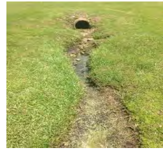
YMCA Park across from the Summer Creek Subdivision –recommended rock lay infrastructure within outlays from ditches
