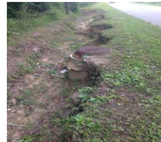
Ditches downstream of Thomas University- recommended BMP-rocklay infrastructure within ditches to alleviate the erosion and collapse. The City Thomasville Engineers were alerted to this issue and are addressing.
