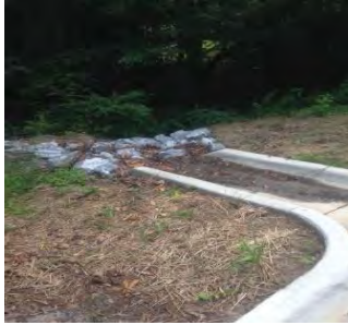
Residential area on Tuxedo drive to alleviate storm water runoff. Installation of this BMP was not at correct slope level and caused more flooding in the home owner's property as well and the street. City of Thomasville Engineers were aware of the issue and were addressing.
