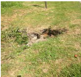
Collapse and blocked storm drain downstream of Thomas University 25 yards past above referenced issue opposite side of street- recommended – address and fix collapse, clear out plugged storm drain. The City Thomasville Engineers were aware of collapse due to working in the area, and send team to clear drain the following day. .
