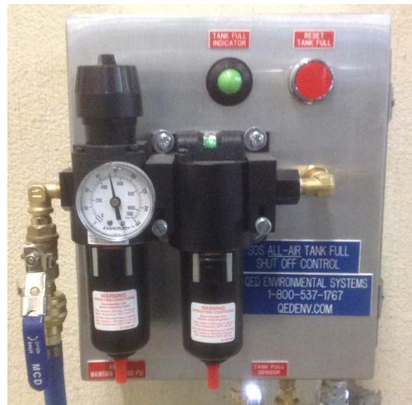
**Photo C-7:** Pneumatic Tank Full Shut Off Control Center
