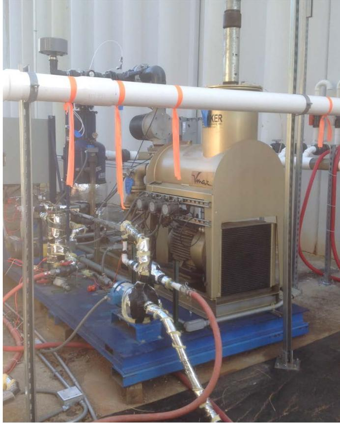
**Photo C-12:** Liquid Ring Pump
