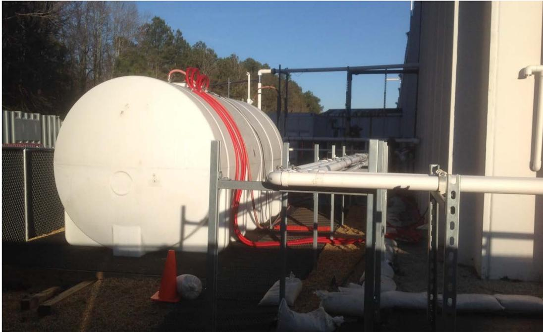
**Photo C-8:** Groundwater Storage Tank and Exterior Piping
