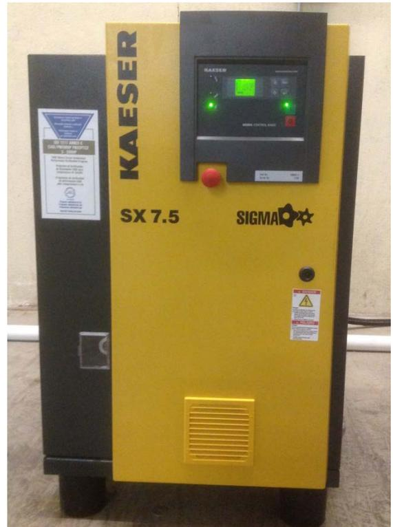
**Photo C-6:** Rotary Screw Air Compressor
