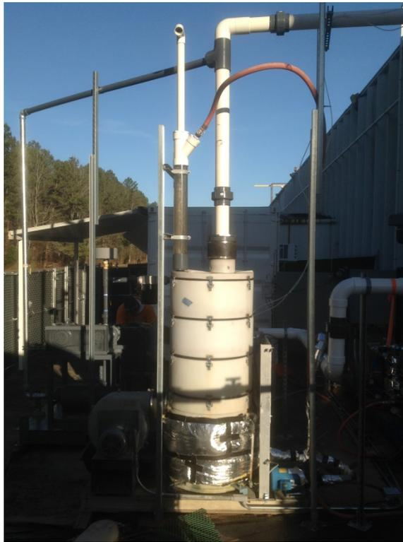
**Photo C-9:** Air Stripper with Advanced Oxidation System (AOS) container in background
