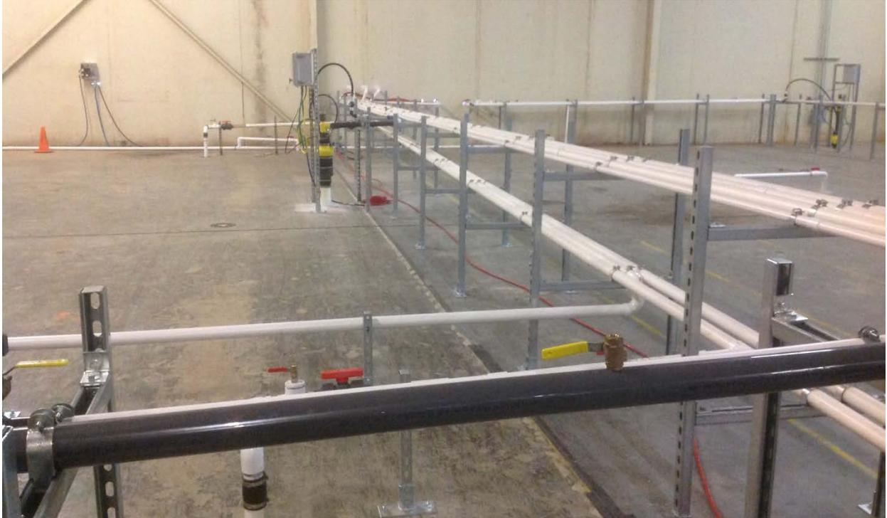
**Photo C-4:** Interior separate-phase extraction well field layout. The MP-1 conveyance piping is depicted in the foreground and the MP-8 and MP-5 installations are shown in the background.
