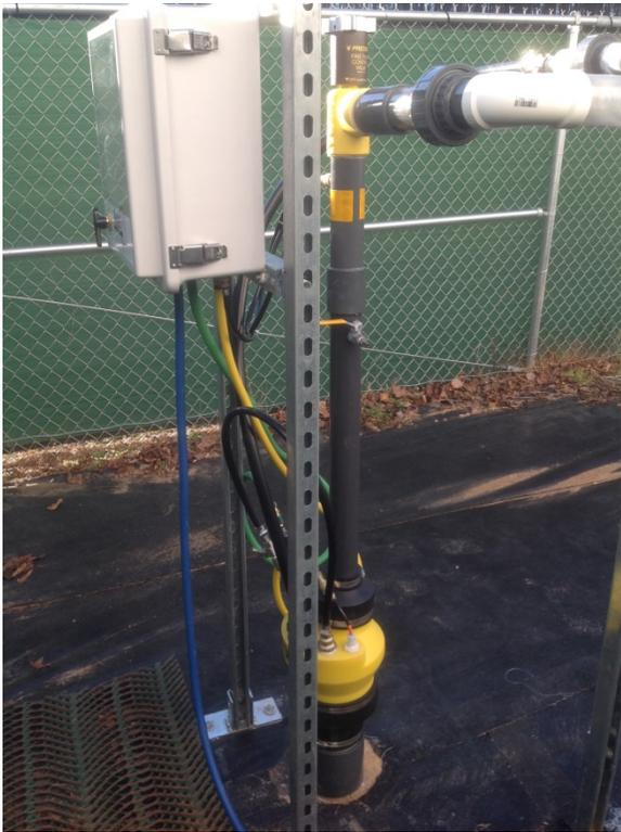
**Photo C-5:** Exterior separate-phase extraction well installation at MP-10.
