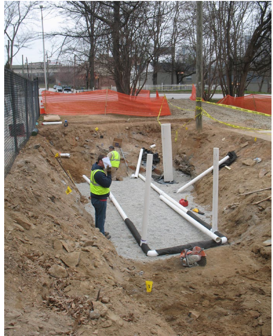
Bioretention under construction in Atlanta, GA.
