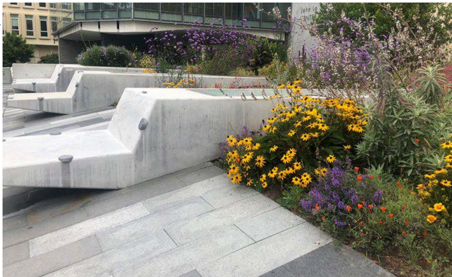
A bioretention practice with beautiful plantings and decorative seating in San Francisco, CA.
