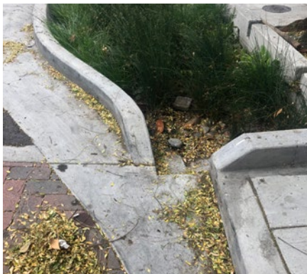
Curb Extension Inlet (Rhea Thompson)
