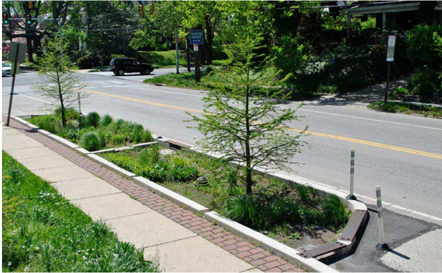
Stormwater curb extension in Philadelphia, PA.
