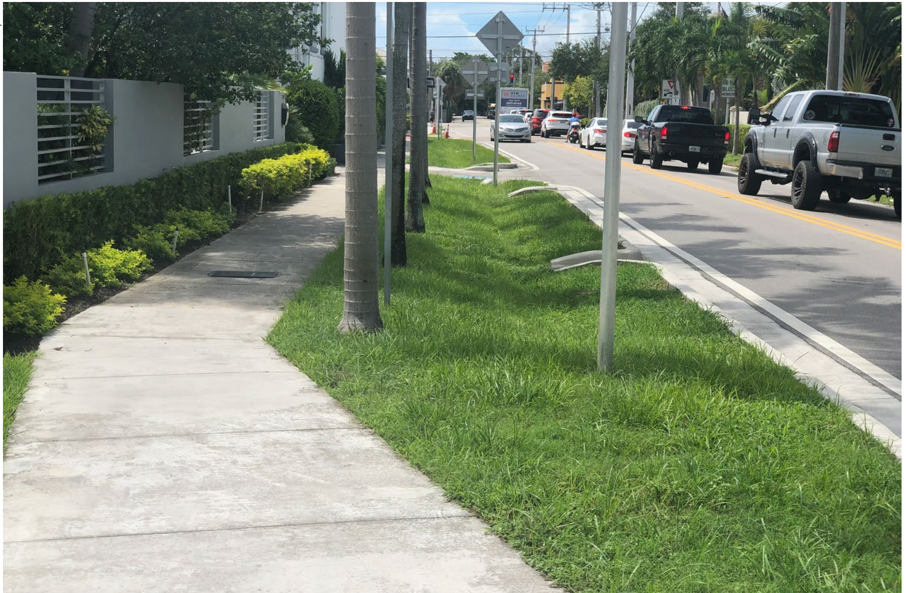
This grassy street-side bioswale is easy to clean and maintain and fits in with the community aesthetic in Fort Lauderdale, FL.
