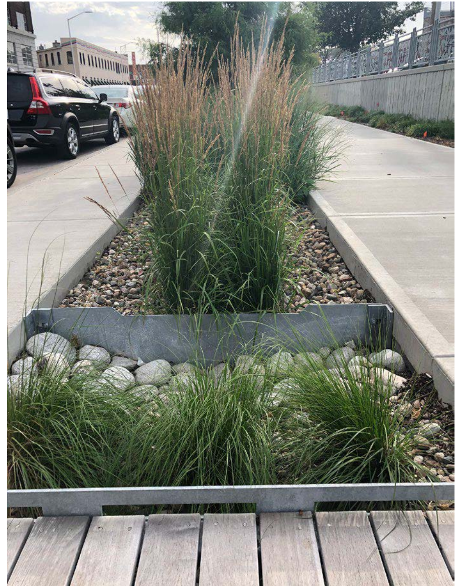
Check dam used for energy dissipation in a bioretention planter box in Kansas City, MO.
