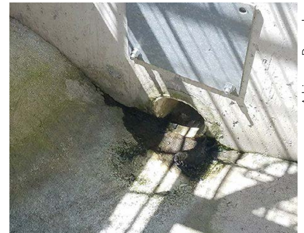
Underdrain outlet in an outlet box.
