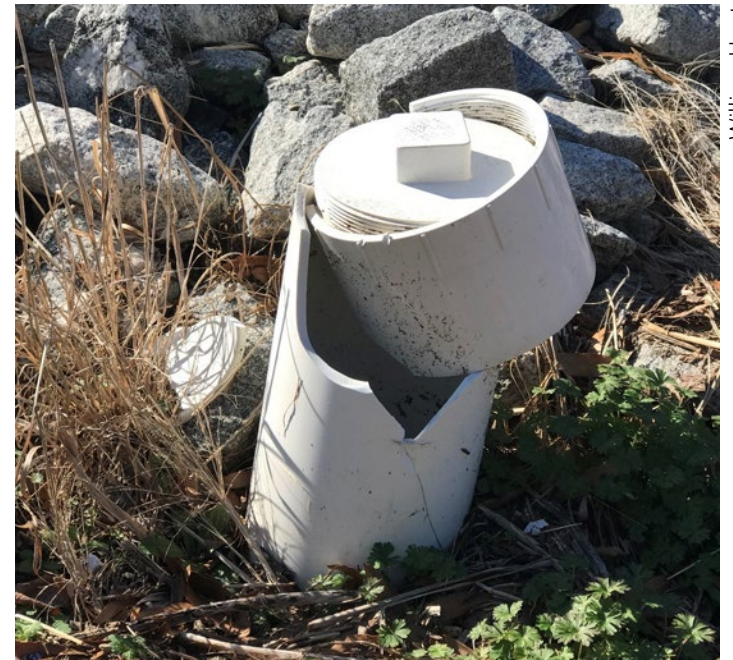
A broken cleanout.
