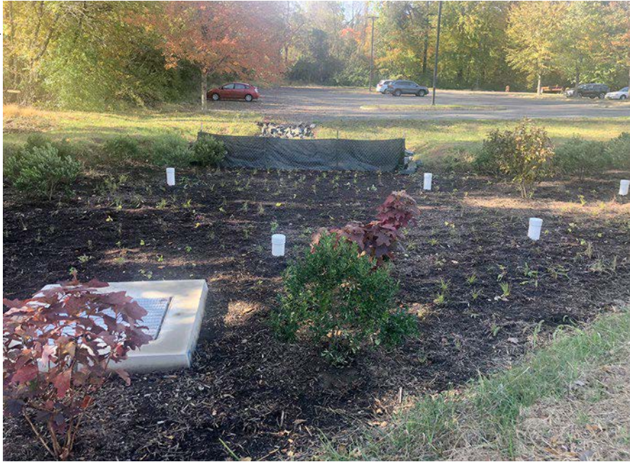
A newly planted bioretention practice in Fairfax, VA.
