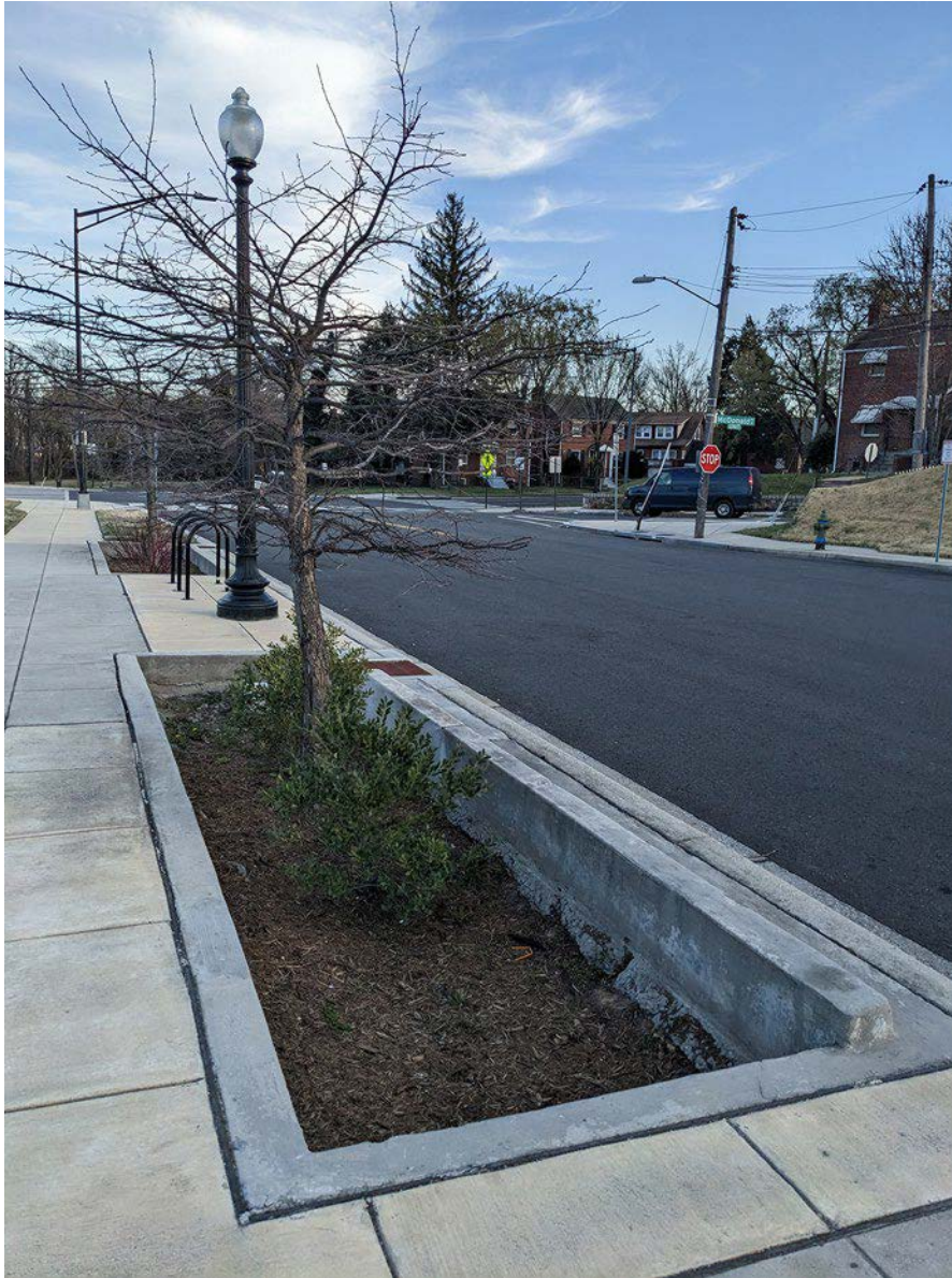
A street-side bioretention planter in Washington, DC.
