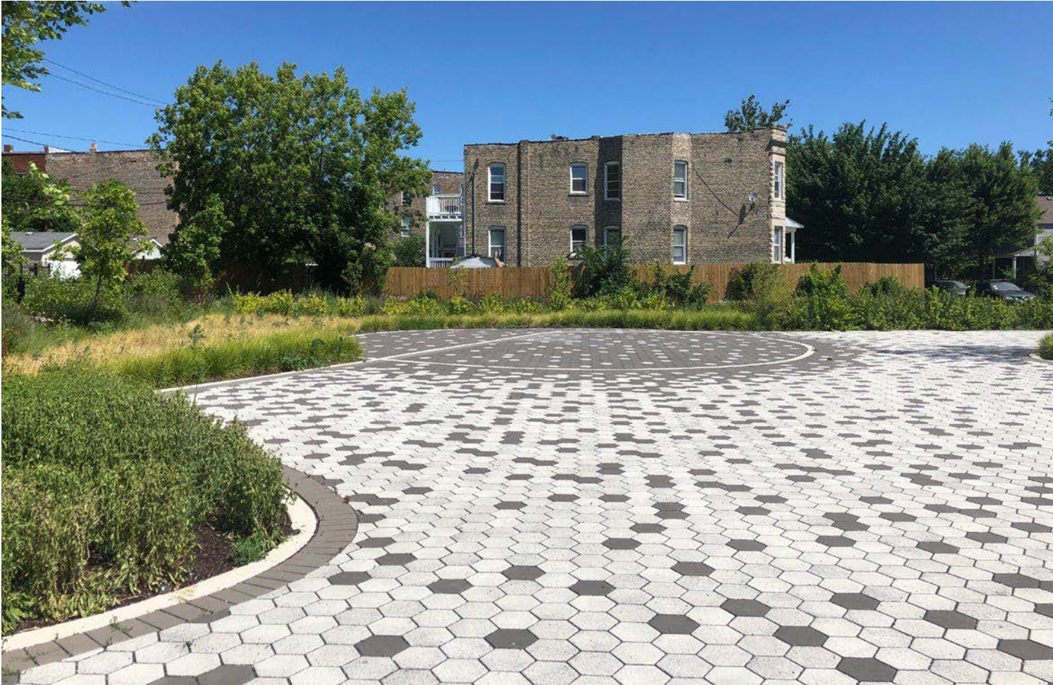
Permeable pavers were installed around this bioretention facility to create a stage and event space for the community in Chicago, IL.
