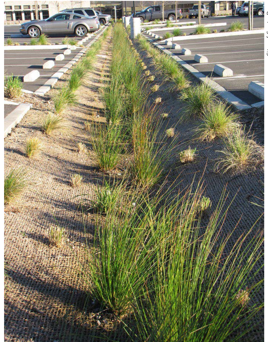
A mesh mat was installed to suppress weed growth in a newly planted bioretention practice in Santa Rosa, CA.
