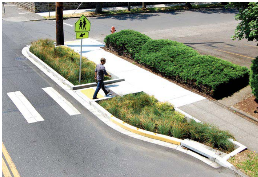
This GSI design treats runoff while guiding pedestrians safely to the crosswalk.
