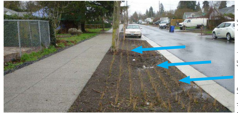
Sheet flow is directed off a residential street by using a gentle slope along the street crown and a curbsless gutter (valley gutter) in Portland, OR.
