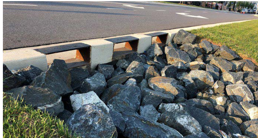
Wheel guards are installed over inlets that are parallel to traffic, such as on this median bioswale in Prince George's County, MD.
