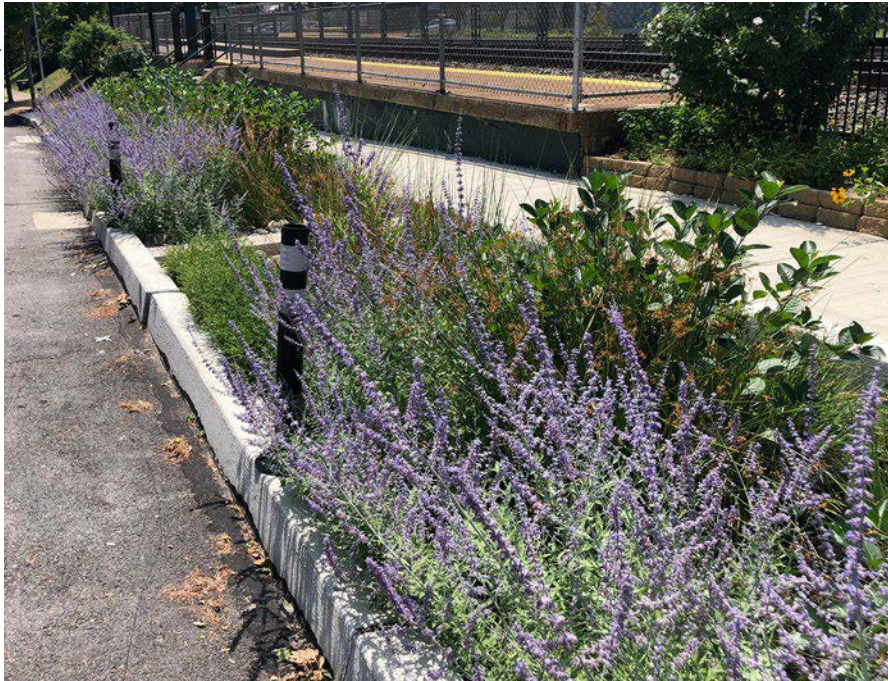
Stormwater curb extension bioretention in Philadelphia, PA.
