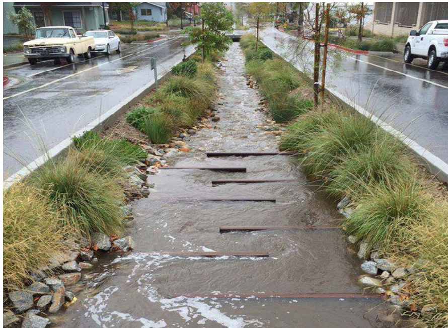
Check dams in a bioretention facility in Paso Robles, CA. These types of in-practice erosion control measures create terraces on the steep grades of sloped streets, prevent erosive flows from entering and damaging bioretention practices, and help control the desired ponding depth. This example also illustrates how check dams can be designed in an artistic manner.
