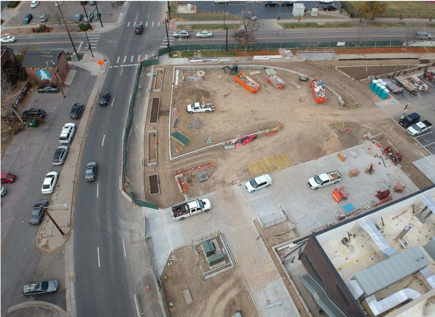
Aerial view of the installation of five bioretention facilities in the ROWs in conjunction with the reconstruction of a city-owned recreation center in Denver, CO. Barriers are being added around the perimeter of the construction staging area for public safety. Note the space reserved for pedestrian pathways to the right of the four bioretention units in the top left.
