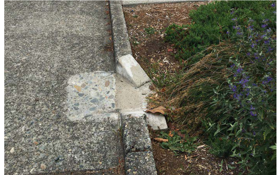
An angled curb cut in Seattle, WA.
