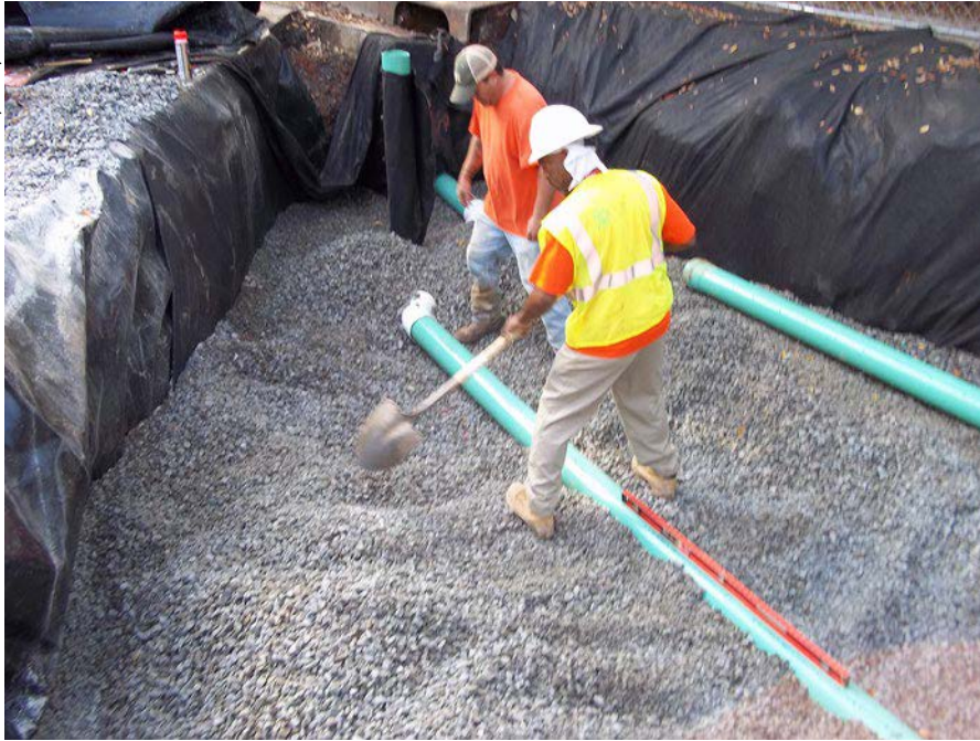
Installing aggregate media in Atlanta, GA.
