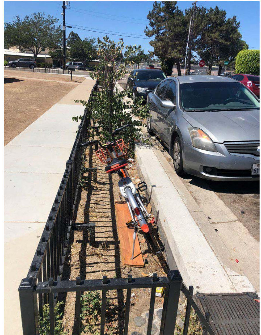
A facility experiencing erosion, unhealthy vegetation, and unwanted bike parking.
