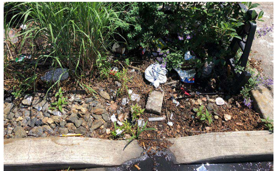
Accumulated sediment and trash needs to be removed from this forebay to ensure proper function.
