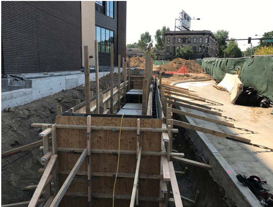
Bioretention under construction in Denver, CO.
