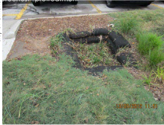
A vegetated bag forebay in Omaha, NE.
