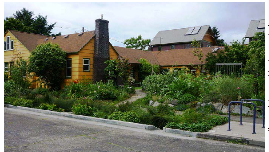
Street-side bioretention in Portland, OR.
