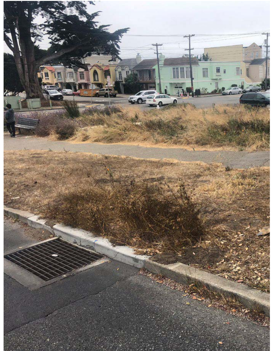
A pipe conveys runoff from a depressed drain to a bioretention facility in San Francisco, CA.
