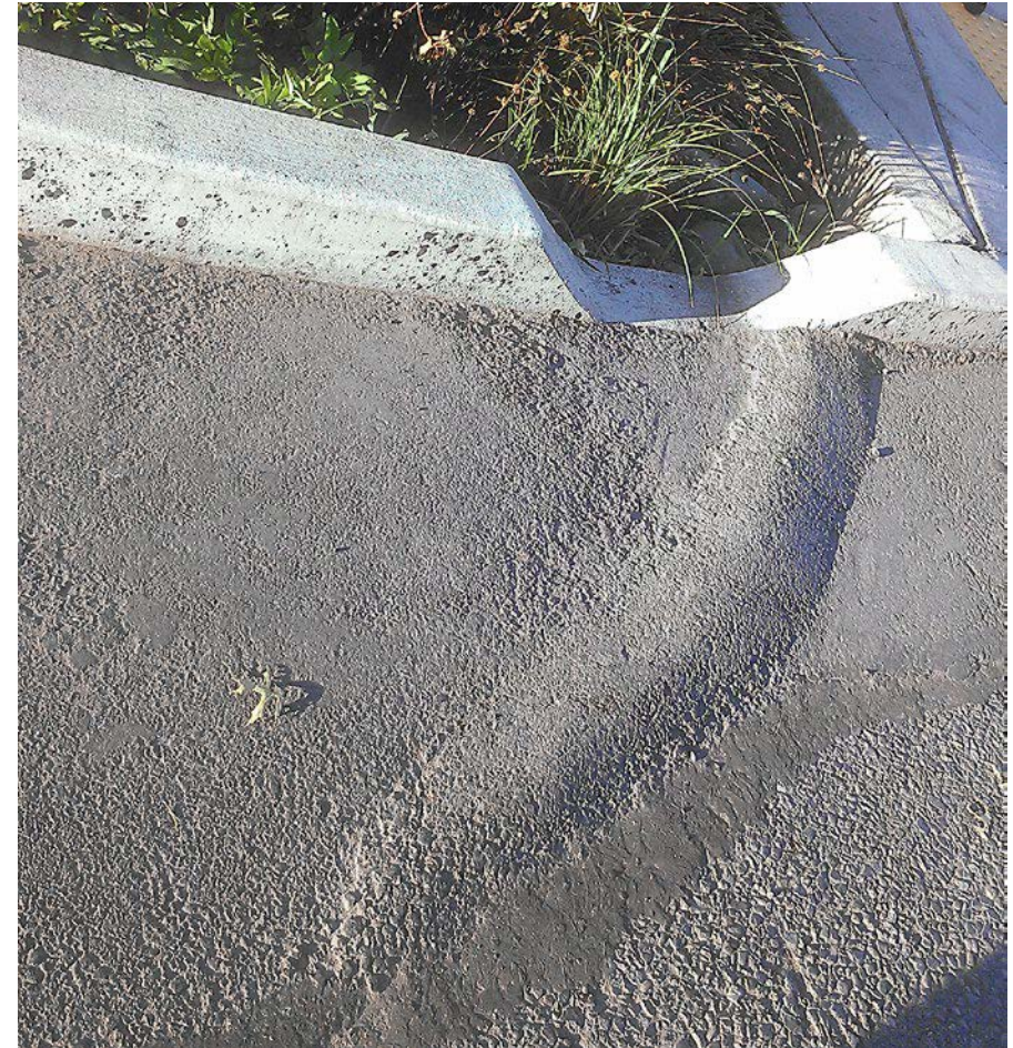
A berm on the downstream side of a curb opening directs runoff.
