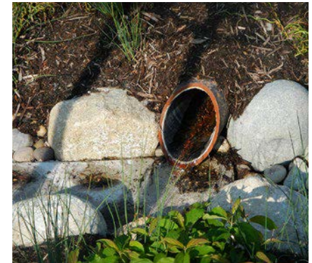
Pipe (City of Seattle and MIG/SvR)
