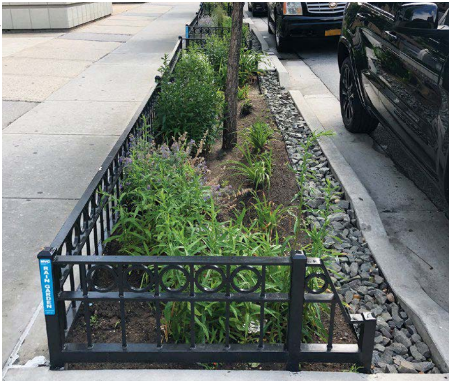
A gravel forebay receives runoff flow and distributes it evenly across this bioretention facility in New York City, NY.
