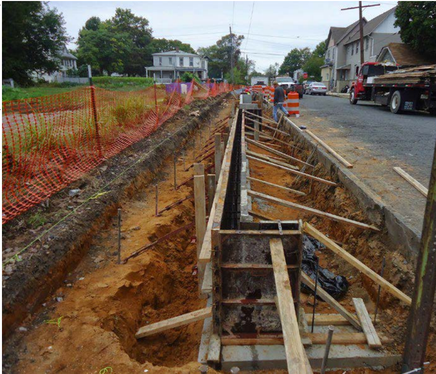
Bioretention under construction in Camden, NJ.
