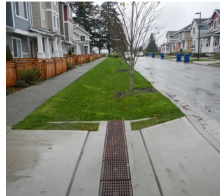
Trench Drain (City of Seattle and MIG/SvR)
