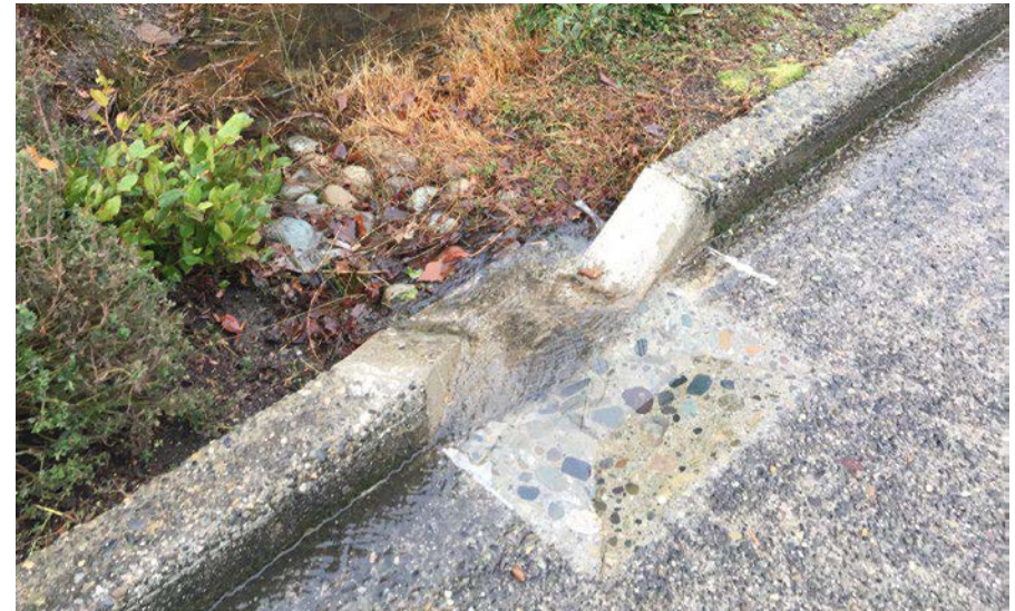
Top: A schematic of a gutter apron. Bottom: A depressed curb cut in Seattle, WA, showing how concrete aprons can be created (retrofitted) by grinding down the existing concrete pavement.
