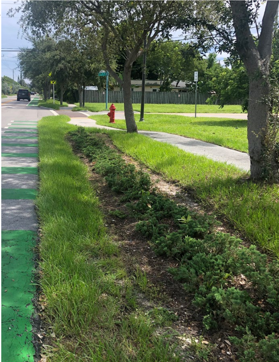
Curbless bioretention with a VFS that treats sheet flow in Fort Lauderdale, FL.
