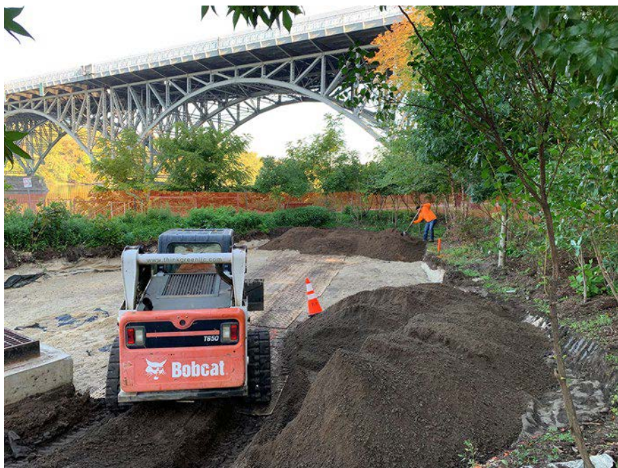
Soilless Soil Initiative project site during construction.
