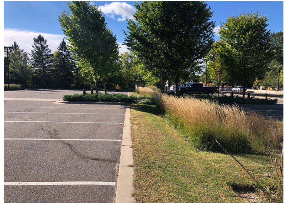
A bioswale includes gentle grades and low-growing vegetation, which fits the parking lot site in Minneapolis, MN.
