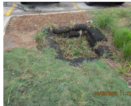
Vegetated Bag Forebay (City of Omaha)
