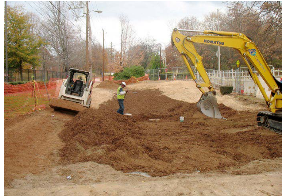
Bioretention facility under construction in Atlanta, GA.
