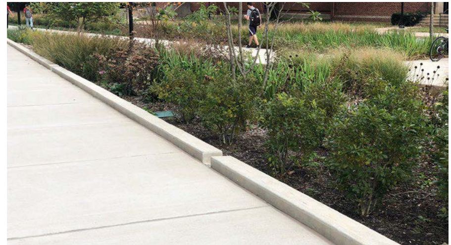
Curbed bioretention with inlets for runoff in College Park, MD.
