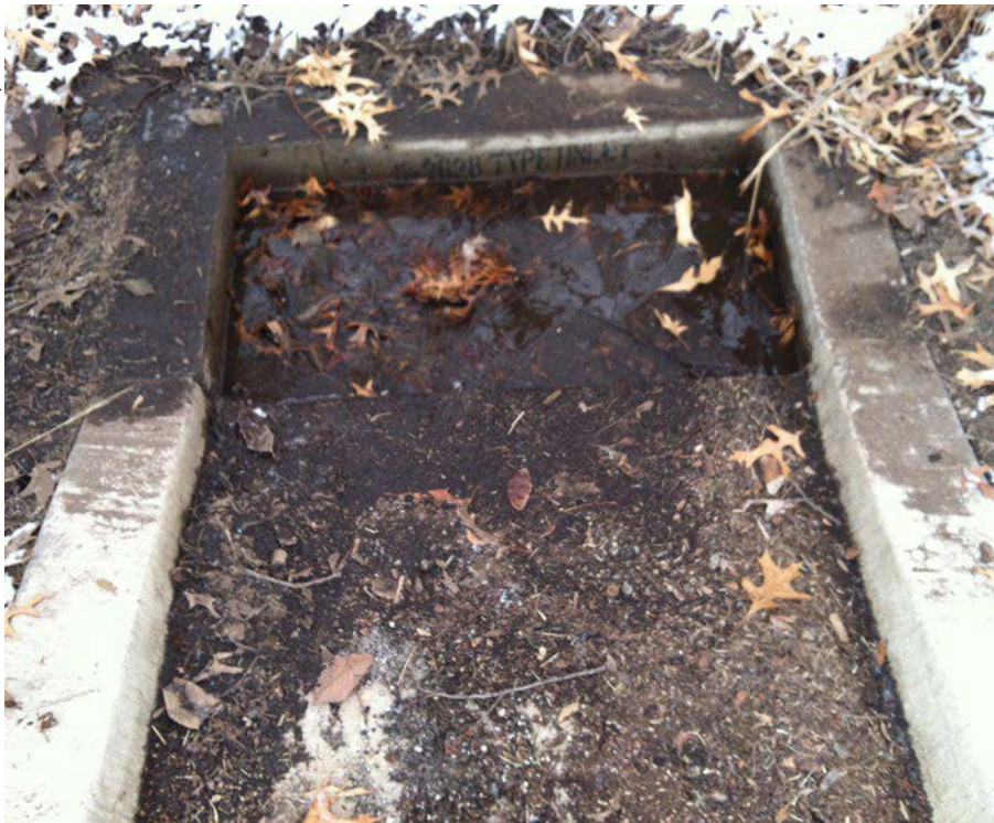
A poorly draining concrete forebay (left) was retrofitted in Kansas City, MO (right).
