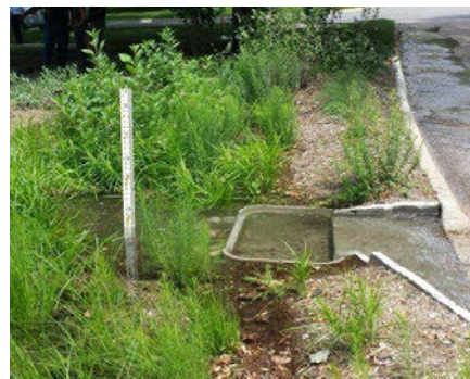
Utility Box Forebay (City of Omaha)
