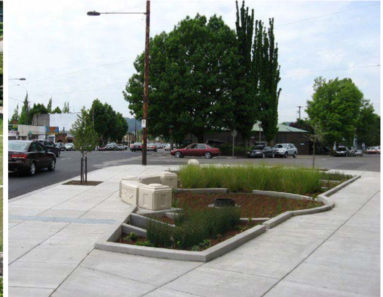
Raised curbs and seating help delineate the edges of the GSI while providing a place for respite in Portland, OR.
