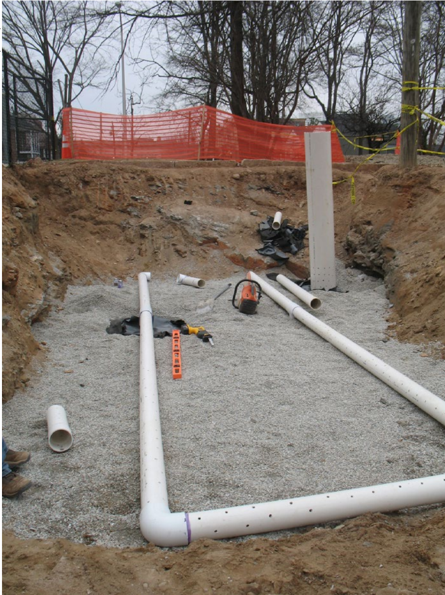
Underdrains being installed in Atlanta, GA.
