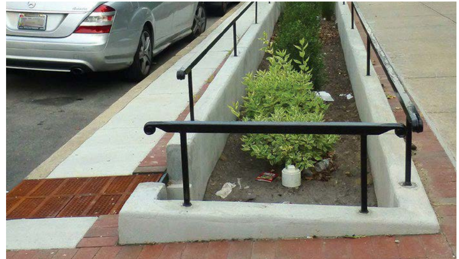
Inadequate pretreatment allowed sediment and debris to accumulate on the surface of a facility in Baltimore, MD.
