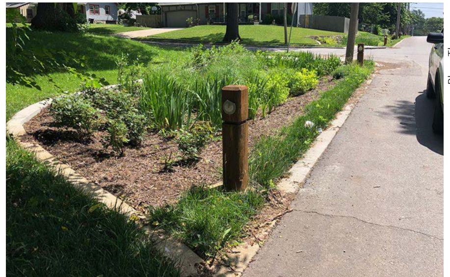
A VFS in a curbside bioretention facility treats incoming sheet flow in Kansas City, MO.
