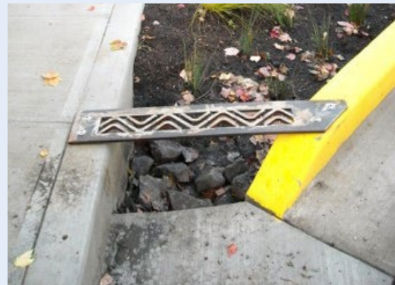
Metal bars added across inlet opening prevents vehicle access.
