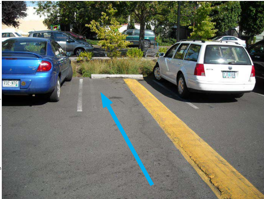
A speed bump intercepts and redirects runoff.
