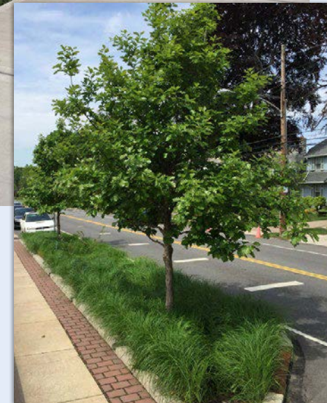
Bioretention facility with trees in Philadelphia, PA.
