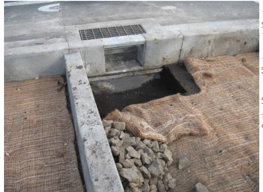
Shallow depressed drains include inlet openings to maintain runoff capacity into the cell if debris accumulates on the grate, Portland, OR.
