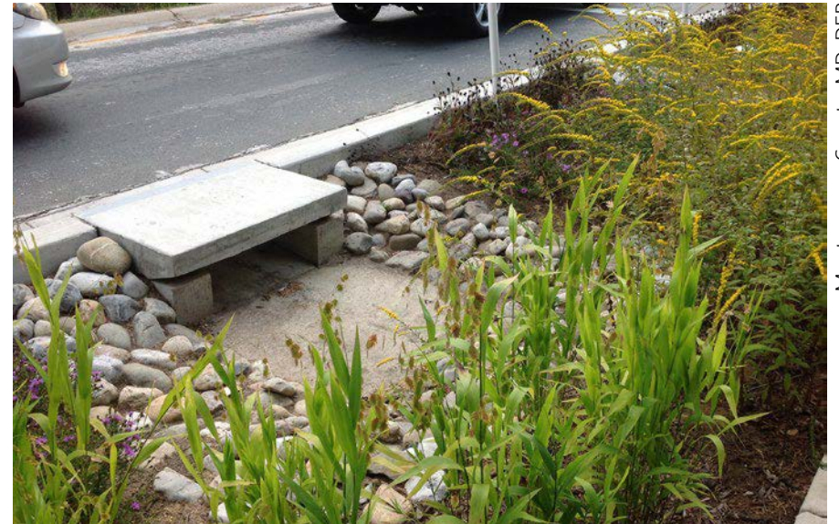
Retrofitted inlet in Montgomery County, MD.
