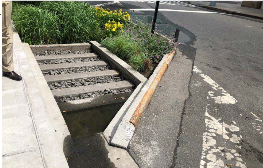
Concrete forebay in New York City, NY.
