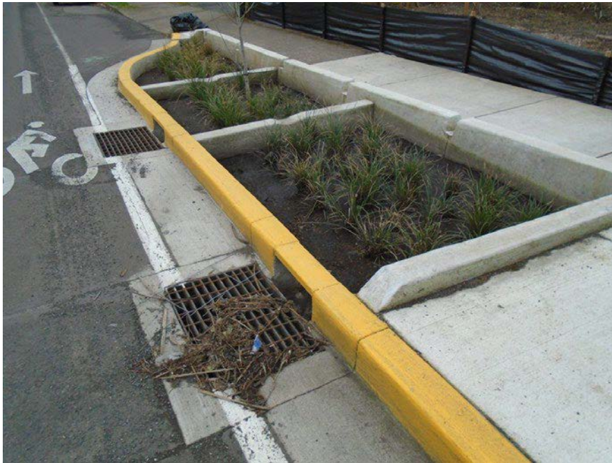
Shallow depressed drains include inlet openings to maintain runoff capacity into the cell if debris accumulates on the grate, Portland, OR.
