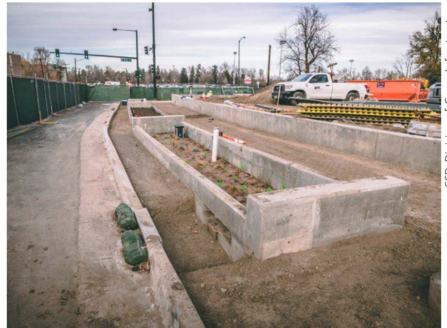
Grass plugs were planted in a newly constructed bioretention facility in Denver, CO.
