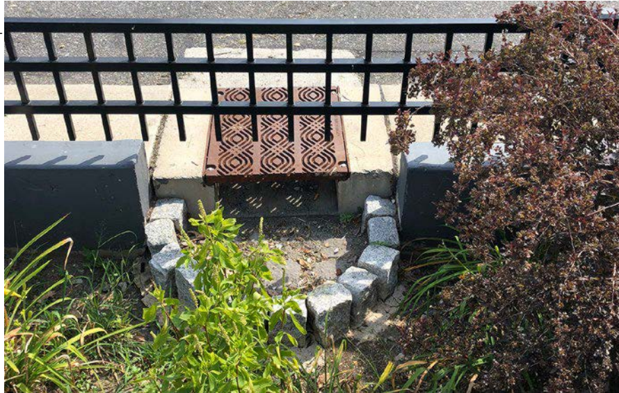
Concrete forebay in New York City, NY.
