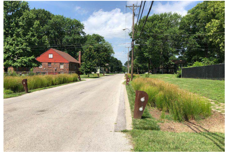
Curbless bioretention in Kansas City, MO.
