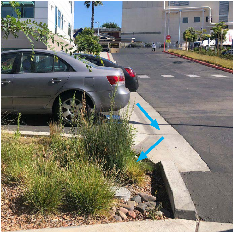
A runnel directs runoff to a bioretention practice in San Diego, CA.
