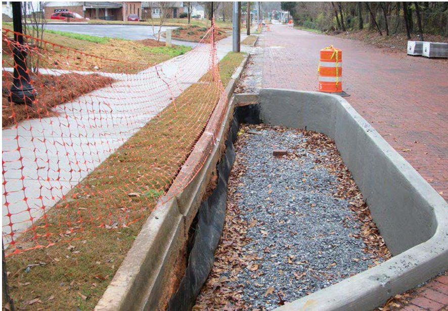
Bioretention under construction in Atlanta, GA.
