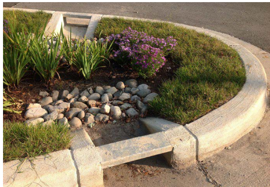
Wheel guards protect openings from vehicles on this stormwater curb extension in Montgomery County, MD.
