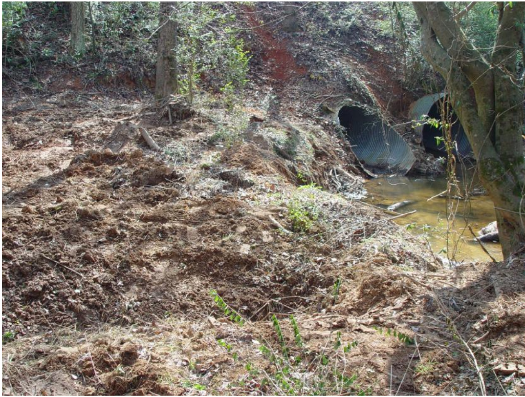
Figure 11. Shiloh Creek: Front loader disturbed soil while clearing culvert of debris - Looking D/S
