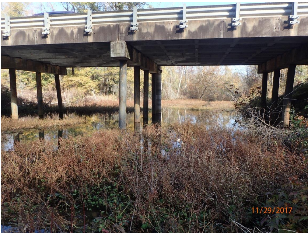
View downstream of Brushy Creek at Highway 80.
