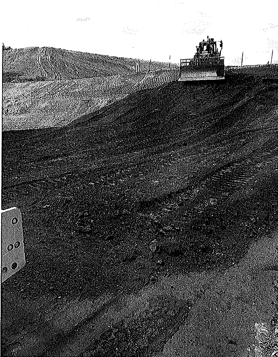
Test pad construction began with a bulldozer spreading a 12" lift of ash material. The test pad for each material was approximately 10' X 15'.
