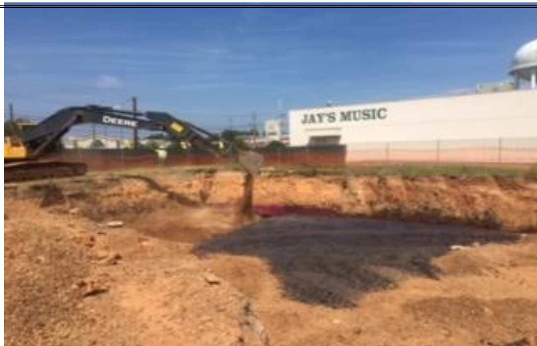
Placement of gravel mixture - Primary AOC Area
