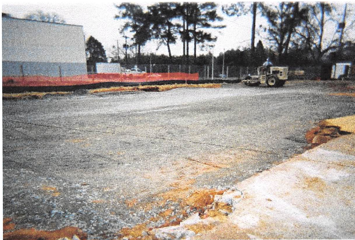
SITE LOCATION: Silverstien Cleaners, Augusta, GA. DESCRIPTION: First lift of backfill crusher run. DATE: 2-20-03 PHOTOGRAPHER: Philip Bodney
