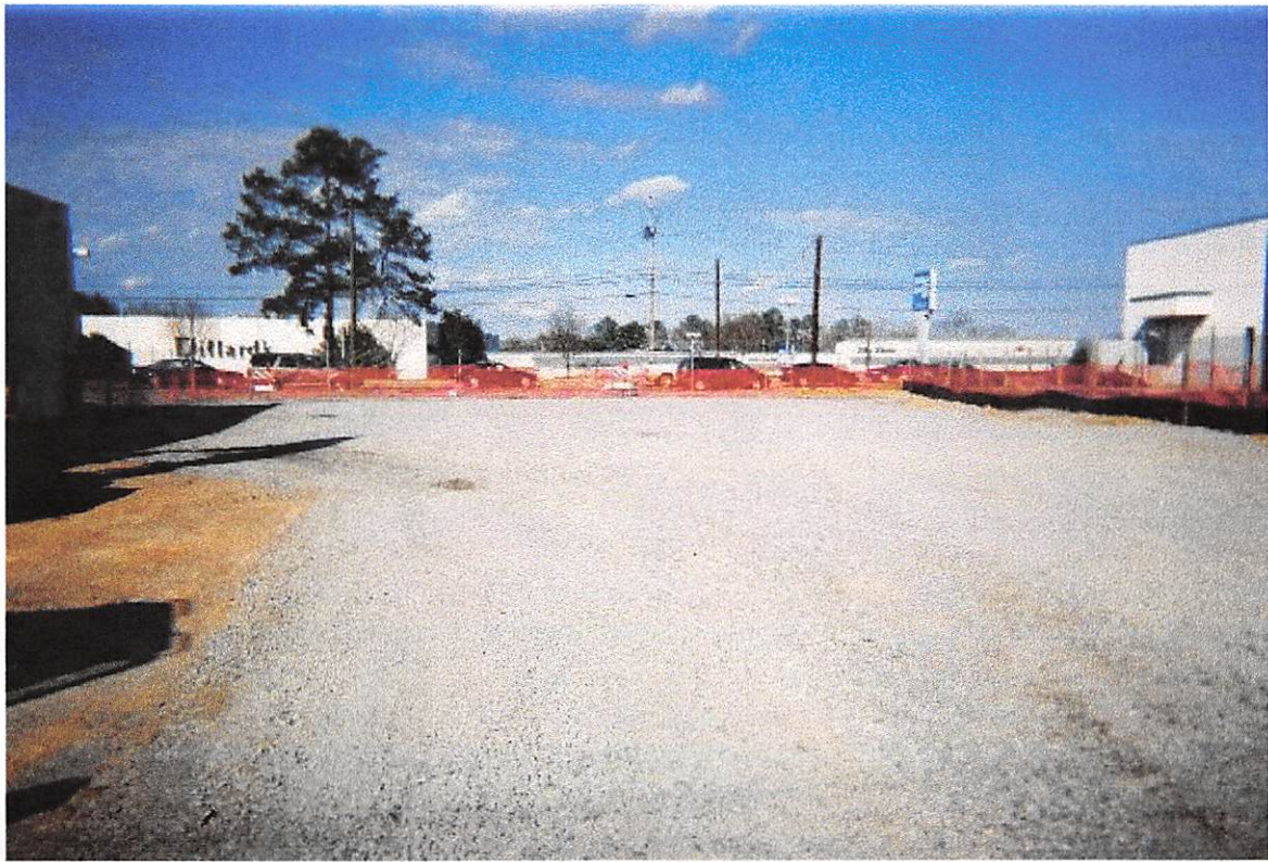
SITE LOCATION: Silverstien Cleaners, Augusta, GA. DESCRIPTION: Final lift of backfill crusher run. DATE: 2-24-03 PHOTOGRAPHER: Philip Bodney
