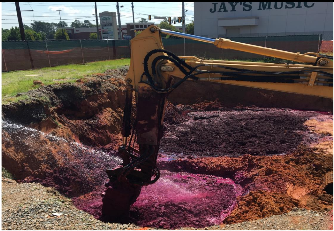
Deep soil mixing – Primary AOC
