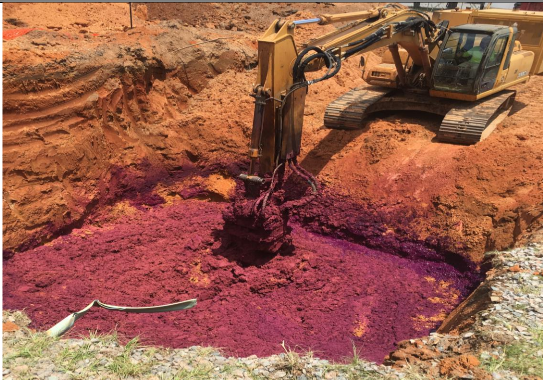
ISCO Soil blending – MW-27 Area
