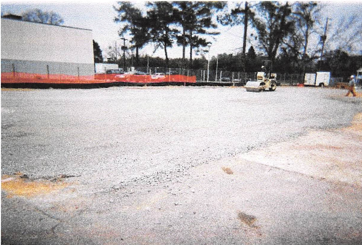
SITE LOCATION: Silverstien Cleaners, Augusta, GA. DESCRIPTION: Final lift of backfill crusher run. DATE: 2-20-03 PHOTOGRAPHER: Philip Bodney
