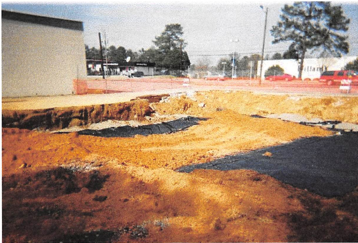
SITE LOCATION: Silverstien Cleaners, Augusta, GA. DESCRIPTION: First lift of backfill soil. DATE: 2-19-03 PHOTOGRAPHER: Philip Bodney
