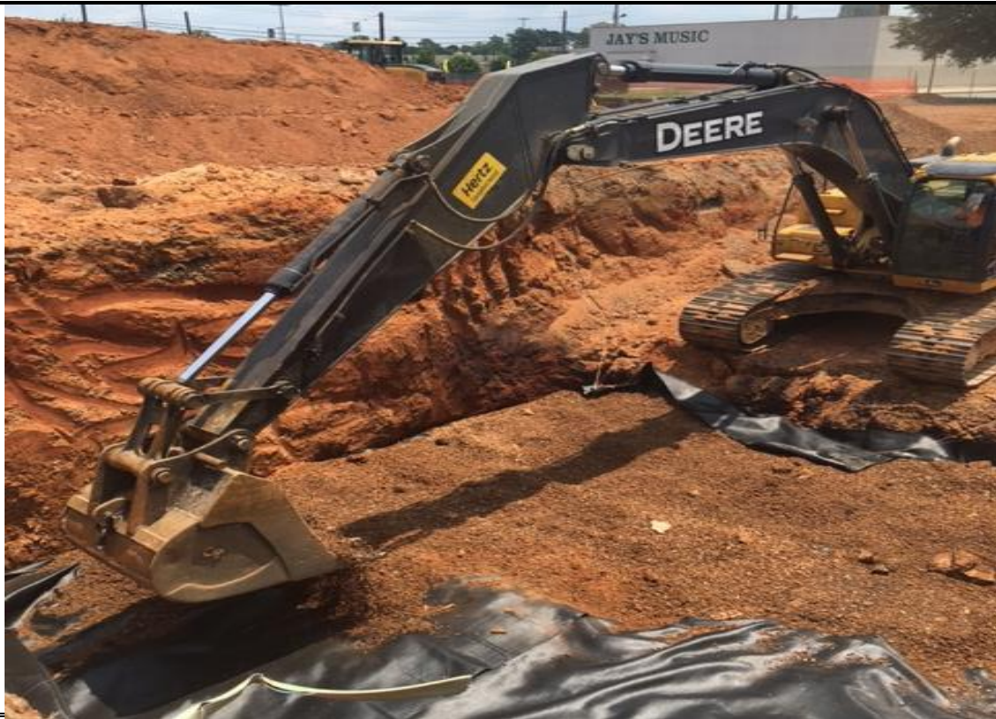
Placement gravel mixture over the geotextile liner – MW-27 Area
