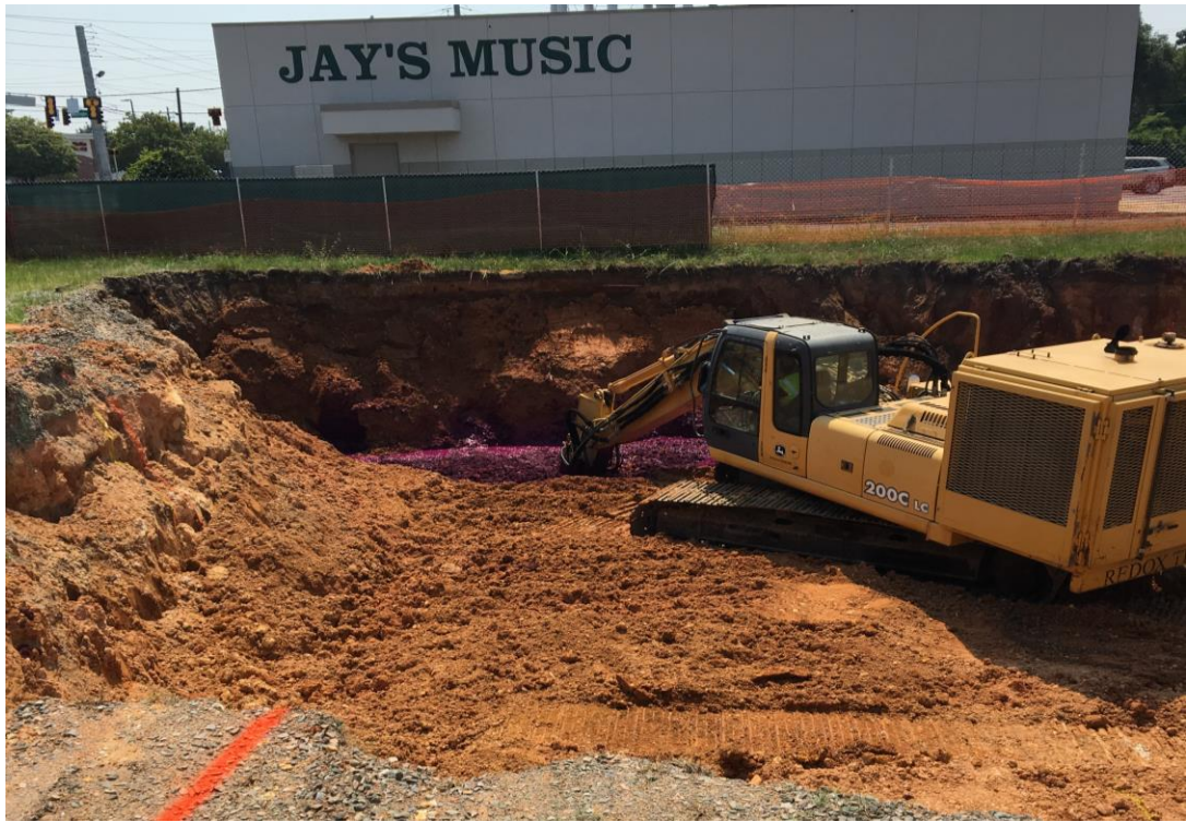
Deep soil mixing – Primary AOC
