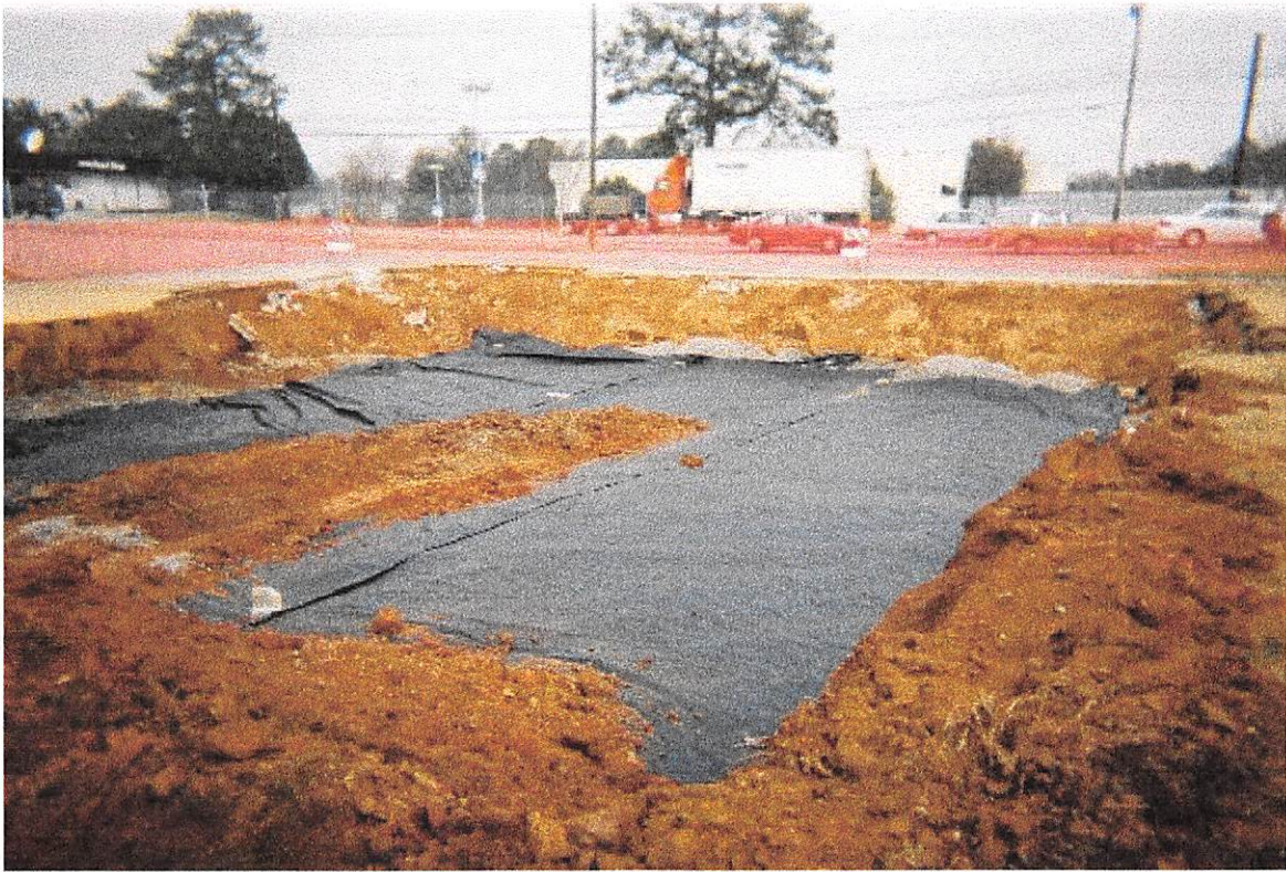
SITE LOCATION: Silverstien Cleaners, ,Augusta, GA. DESCRIPTION: Laying of fabric. DATE: 2-19-03 PHOTOGRAPHER: Philip Bodney
