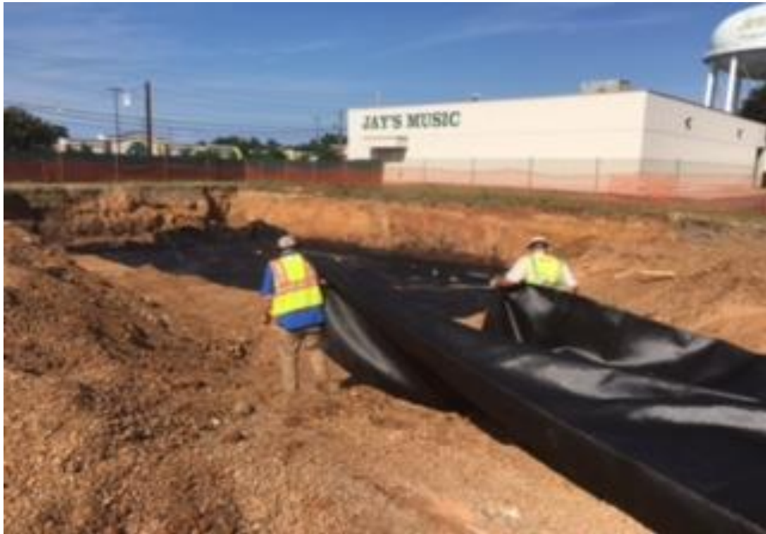
Placement of geotextile liner – Primary AOC
