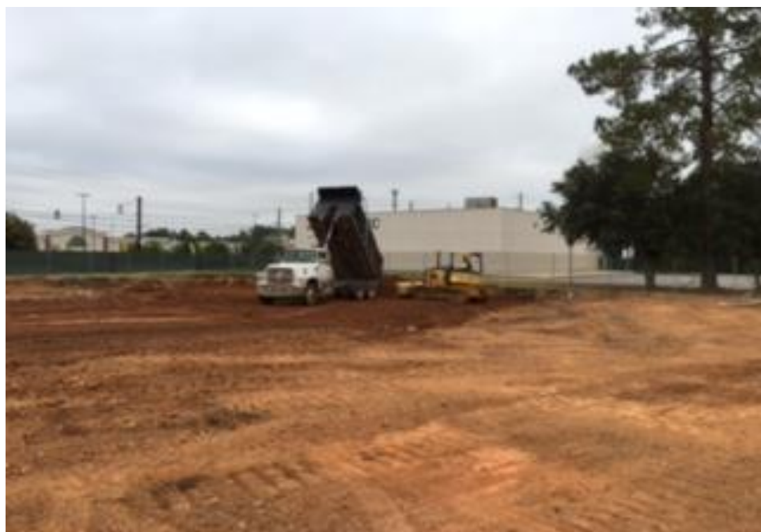
Placement of overburden – Primary AOC Area
