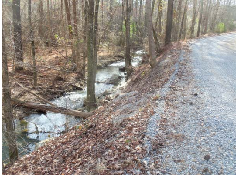
Figure 3.5. Photo showing unpaved section of Flowery Branch Road with gravel washing down the bank into Dykes Creek.
