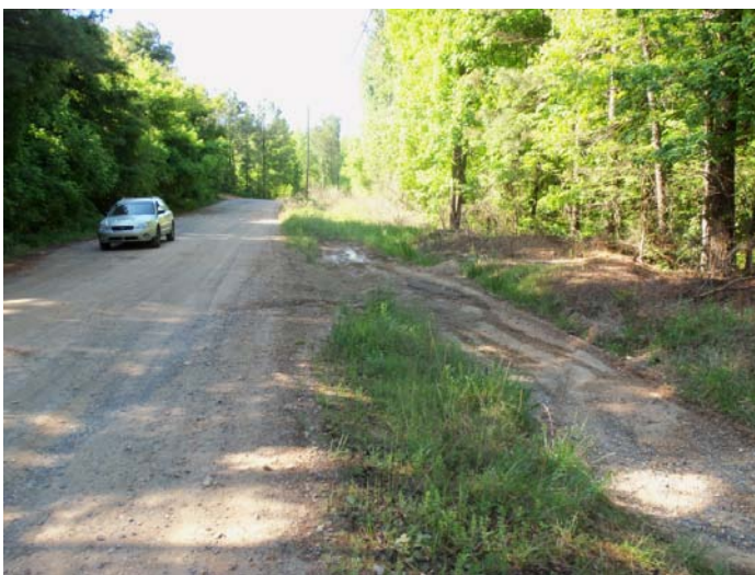
Figure 3.2. Road in Shannon Oaks Subdivision off of Firetower Road. Note large accumulation of sediment on right from road.
