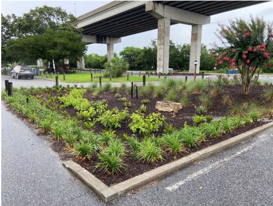
Figure 6: Liberty Ship Park Bioretention Cell (South) – FY2020 GI/LID Retrofits in Brunswick – From Planning to Implementation
