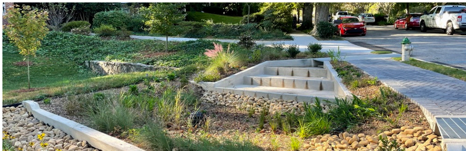
Figure 14: Bioretention system - FY2021 Huron & Champlain Streets Bioretention Basin Improvement Project
