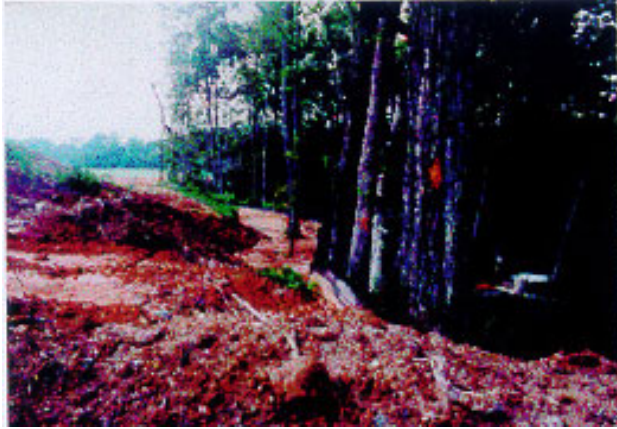
Figure 4-1. 7 Slope grade reduction from panning. Figure 4-1. 8 Soil encroachment toward silt fence.
