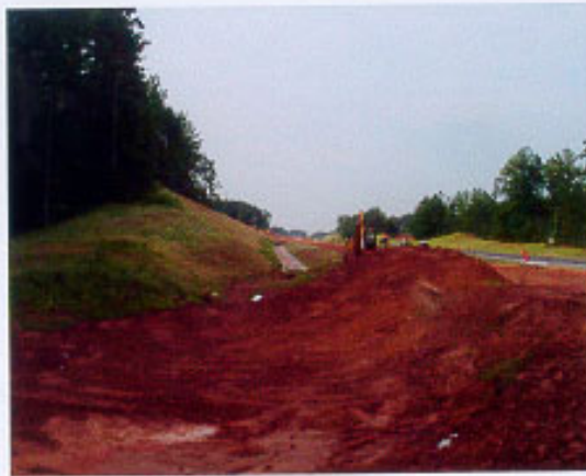
Figure 4-3. 1 Highway basin cleanout.
