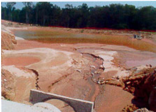
Figure 4-2. 9 Excessive deposition at inlet.
