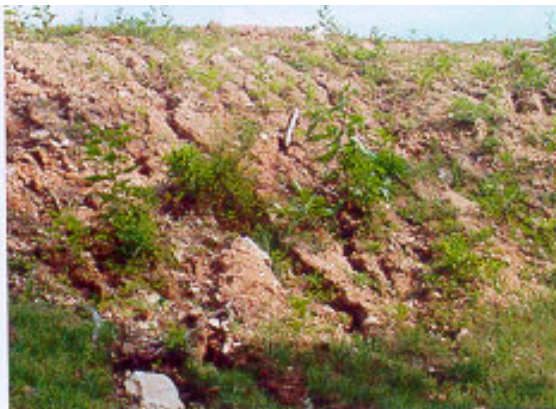
Figure 4-1. 4 Rills and gullies in steep slope.
