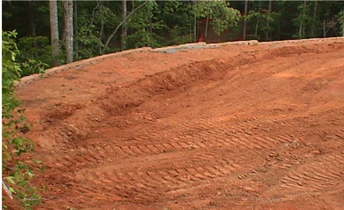
Figure 5- 20 Typical temporary earthen berm to protect a steep structural fill slope near basin B1.
