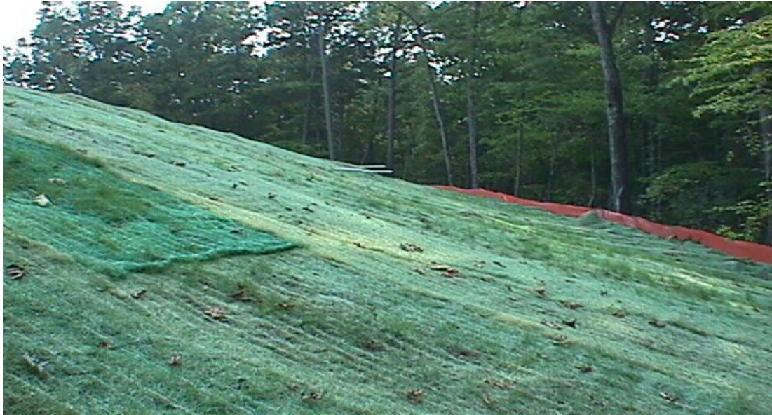
Figure 5- 26 Protection of basin B1 outslope by commercial erosion control product.
