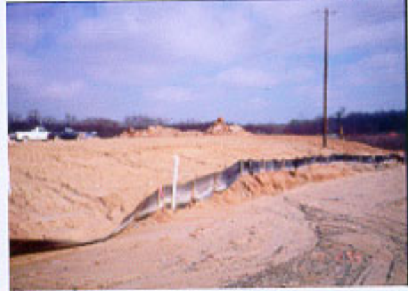
Figure 4-2. 18 Silt fence failure.
