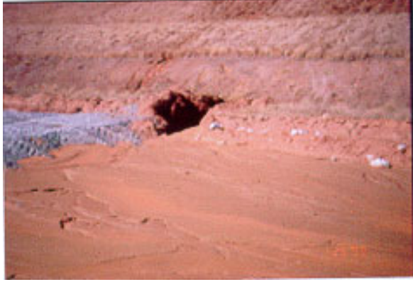
Figure 4-3. 17 Sediment bypass cut on roadbed.
