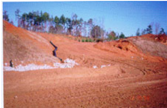
Figure 4-3. 21 Up-gradient new intersection w/ drain.
