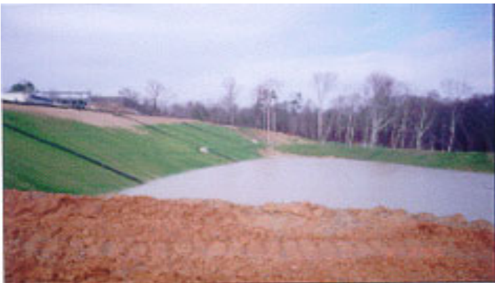
Figure 4-2. 19 Stabilized basin with vegetation and down-drains.
