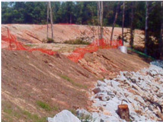
Figure 4-2. 7 Embankment erosion from dam breach.
