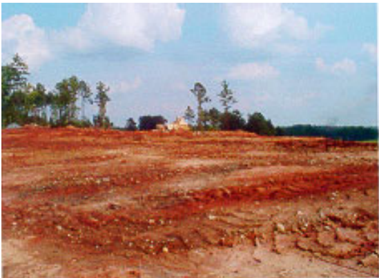
Figure 4-1. 5 Active grading area above steep slope.
