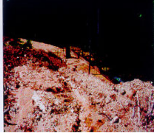
Figure 4-1. 7 Slope grade reduction from panning. Figure 4-1. 8 Soil encroachment toward silt fence.
