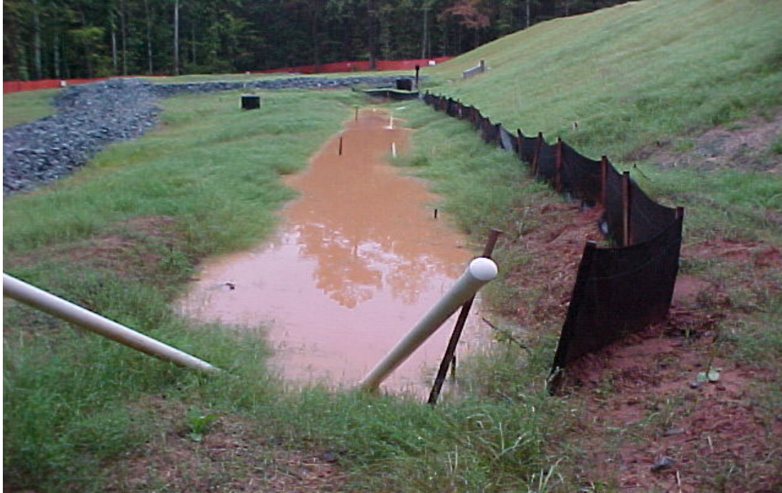
Figure 5- 18 Basin B2 sand filter in operation.
