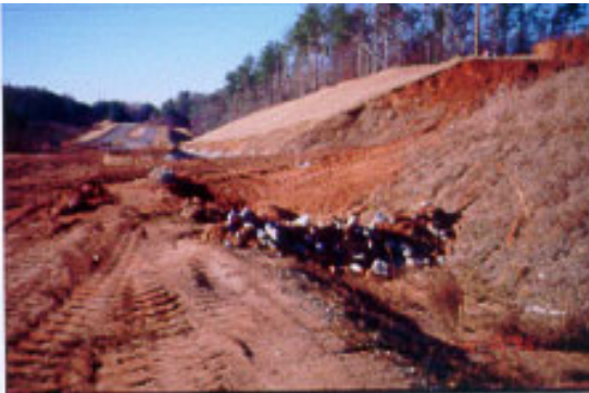
Figure 4-3. 22 Channel w/ rock check dam.
