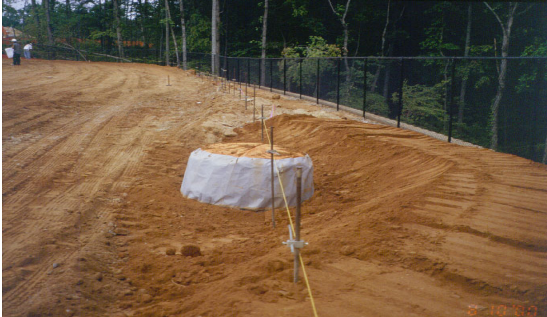
Figure 5- 21 Temporary earthen berm inlet protected by a silt stack covering.
