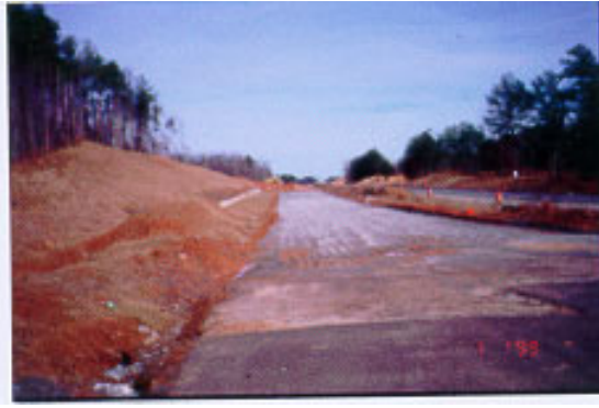
Figure 4-3. 12 Aggregate placed on roadbed.
