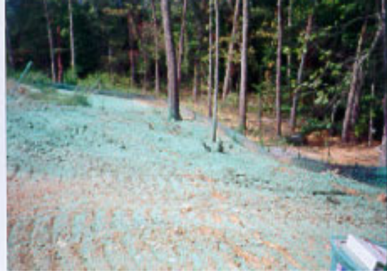
Figure 4-1. 14 Hydro-seeded slope.
