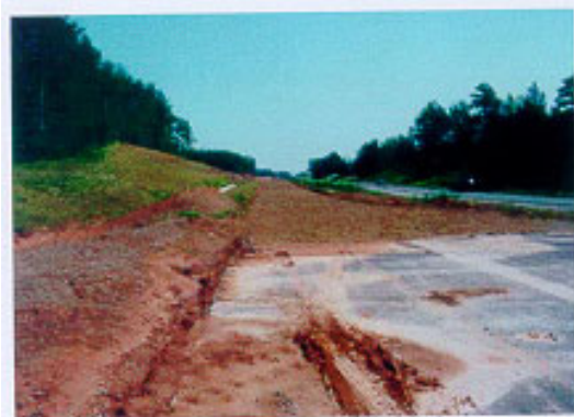
Figure 4-3. 7 Straw mulch on graded road base. Figure 4-3. 8 Deposition in basin and PSW location.
