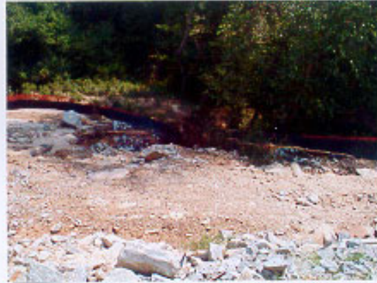
Figure 4-2. 8 Silt fence undercutting.
