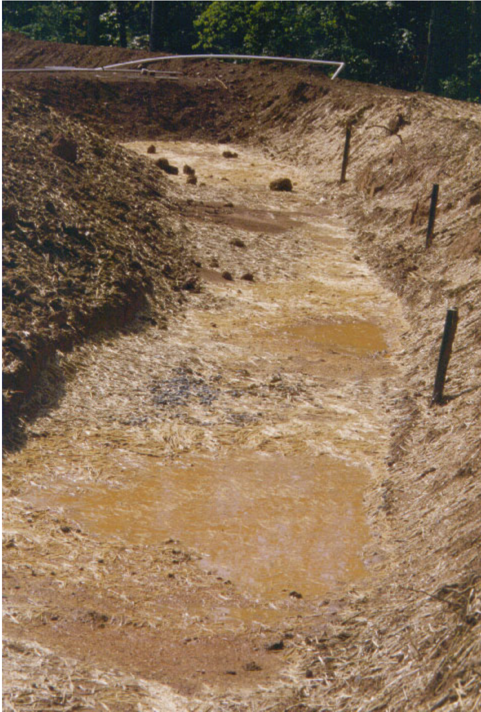
Figure 5- 5 Photograph of seep berm at the Big Creek site illustrating the berm, check dam, and perforated risers.
