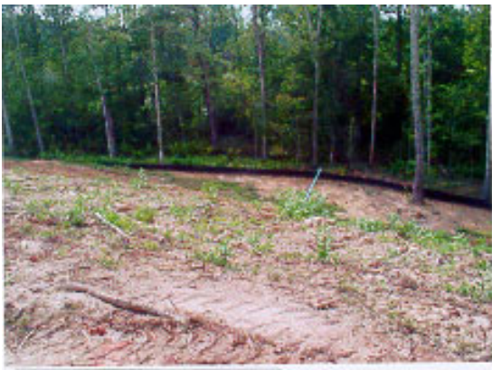
Figure 4-1. 3 Slope up-gradient from silt fence.
