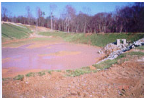
Figure 4-2. 14 Grass establishment on inslopes.
