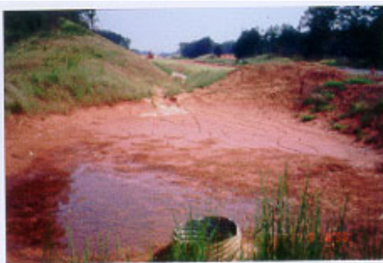
Figure 4-3. 7 Straw mulch on graded road base. Figure 4-3. 8 Deposition in basin and PSW location.
