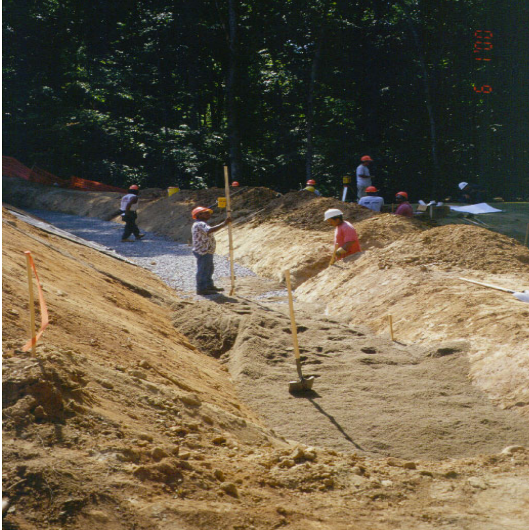
Figure 5- 17 Basin B1's sand filter under construction.
