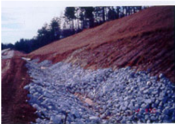
Figure 4-3. 13 Silt checks replaced with riprap.
