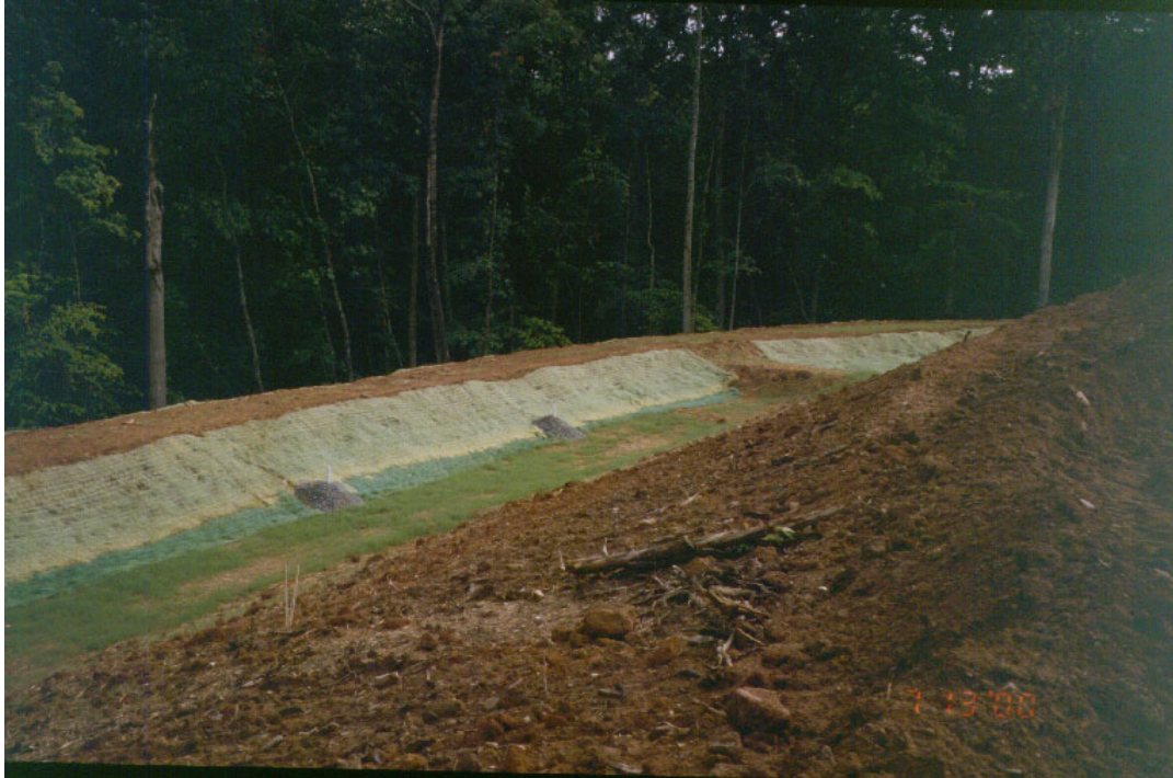
Figure 5- 6 Big Creek seep berm with stabilized berm and forested area.
