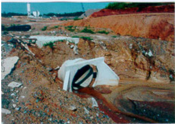
Figure 4-2. 11 Headwall dislodged, Aug 1998.
