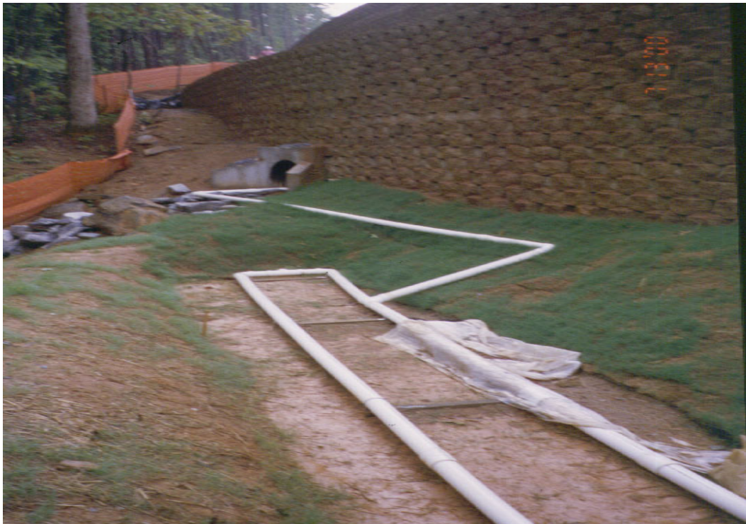
Figure 5- 19 Temporary basin B4's completely constructed sand filter showing the conveyance pipe from the basin to the sand filter and the surface distribution pipes.
