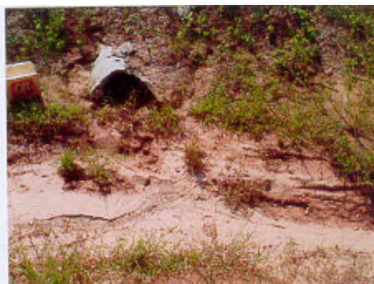
Figure 4-3. 9 Scour hole from down-drain. Figure 4-3. 10 Deposition in channel prior to basin.
