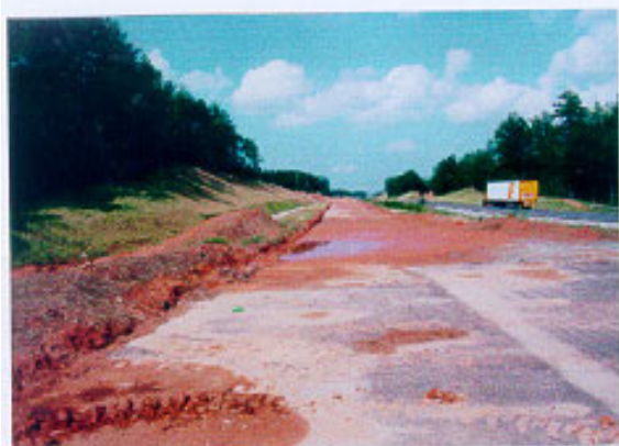
Figure 4-3. 5 Up-gradient view of road widening. Figure 4-3. 6 Erosion at end of concrete channel.
