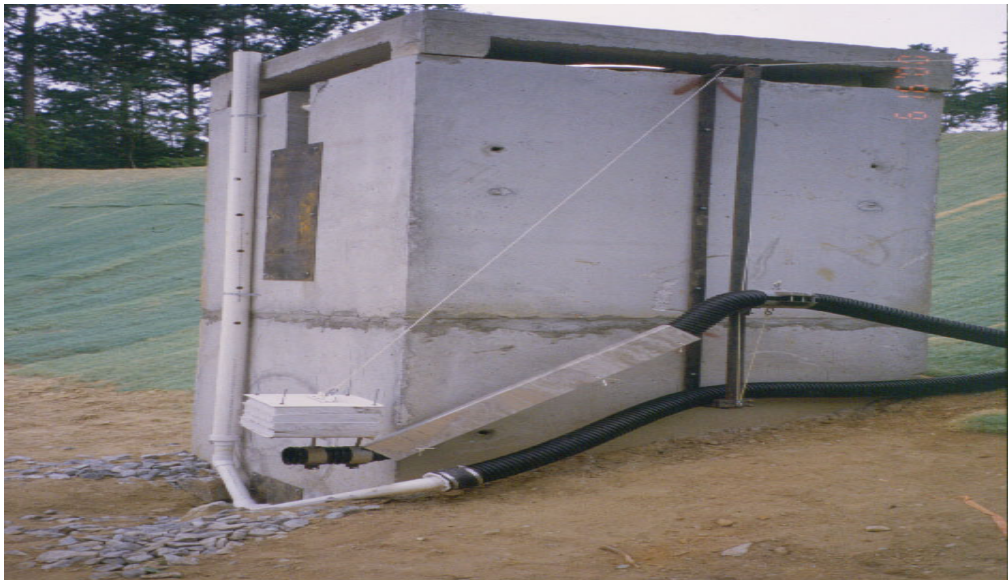
Figure 5- 13 Basin B2's drop inlet, small perforated riser, and floating siphon.
