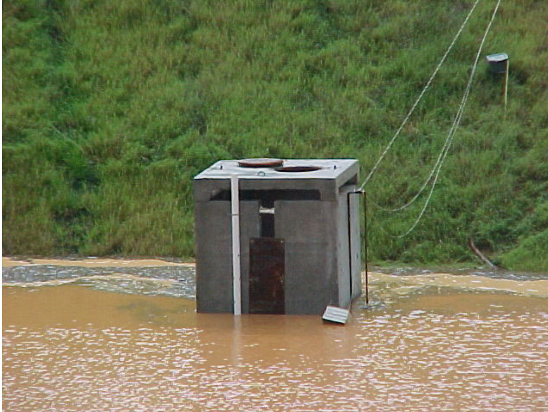
Figure 5- 14 Side view of basin B2's drop inlet, small perforated riser, and floating siphon.
