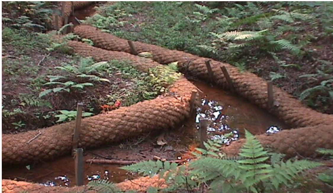
Figure 5- 23 Coir logs used for stream slope protection.
