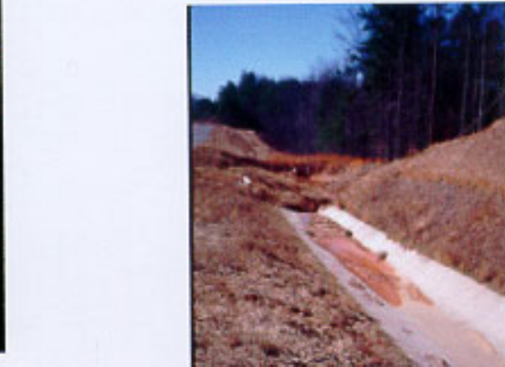
Figure 4-3. 24 Deposition in concrete channel.
