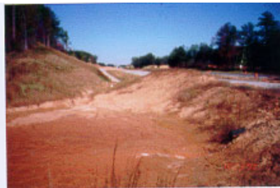
Figure 4-3. 16 Sediment build-up in basin.
