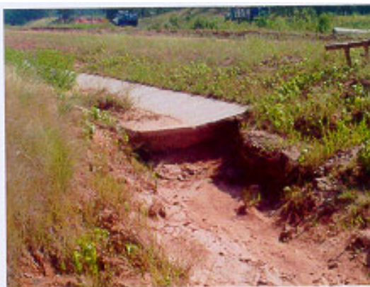
Figure 4-3. 5 Up-gradient view of road widening. Figure 4-3. 6 Erosion at end of concrete channel.
