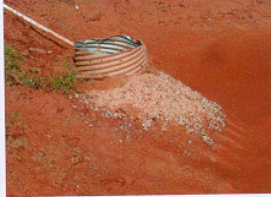
Figure 4-3. 18 Sediment caking on stone apron.
