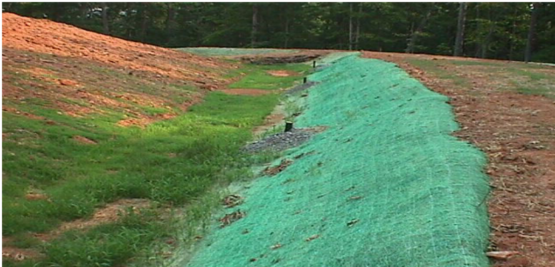
Figure 5- 27 Example of protecting the inslope of the seep berm by a commercial erosion control product.
