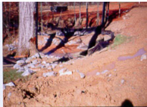
Figure 4-1. 11 Steep slope groomed and flattened. Figure 4-1. 12 New stream crossing.
