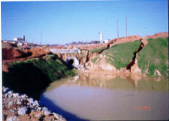
Figure 4-2. 17 Eroded gully on grassed slope.
