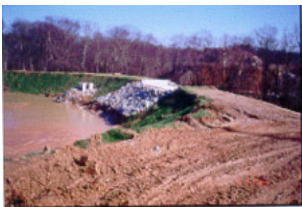
Figure 4-2. 15 Emergency spillway in place.
