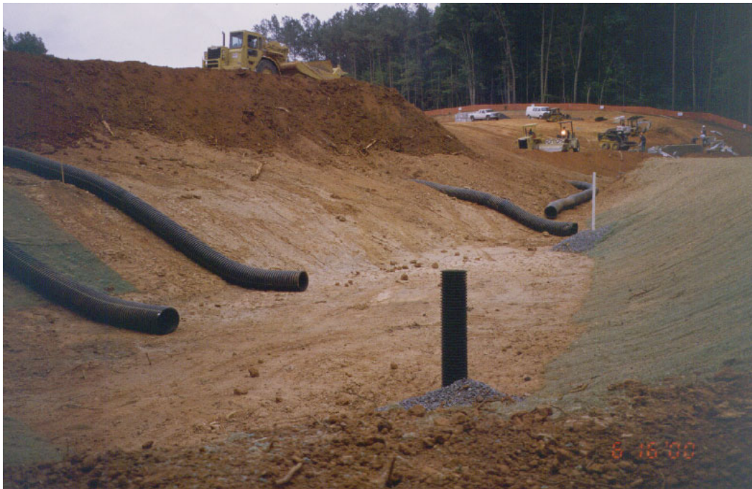
Figure 5- 22 Down-drain lines safely conveying runoff from the temporary earthen berm to basin B1.
