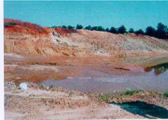
Figure 4-2. 10 Slope erosion from large rainfall event.
