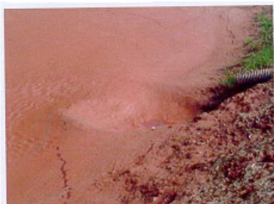
Figure 4-3. 9 Scour hole from down-drain. Figure 4-3. 10 Deposition in channel prior to basin.
