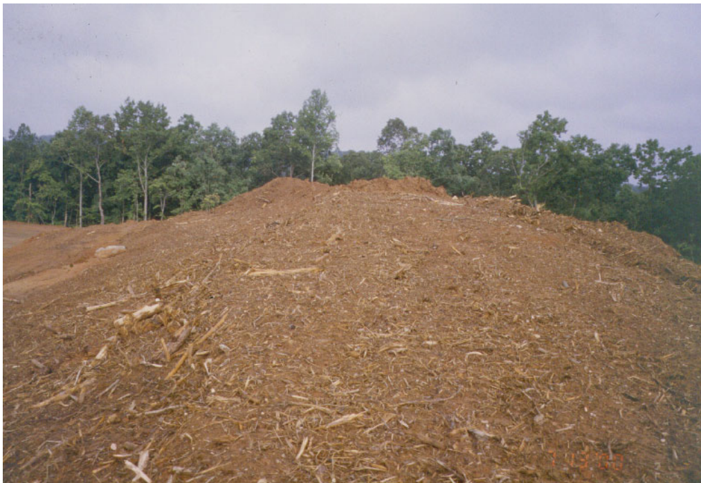
Figure 5- 25 Example of using on-site produced rough-grade mulch for erosion prevention.
