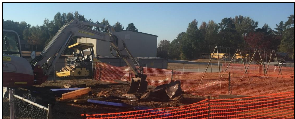
Soil excavation in school yard.
