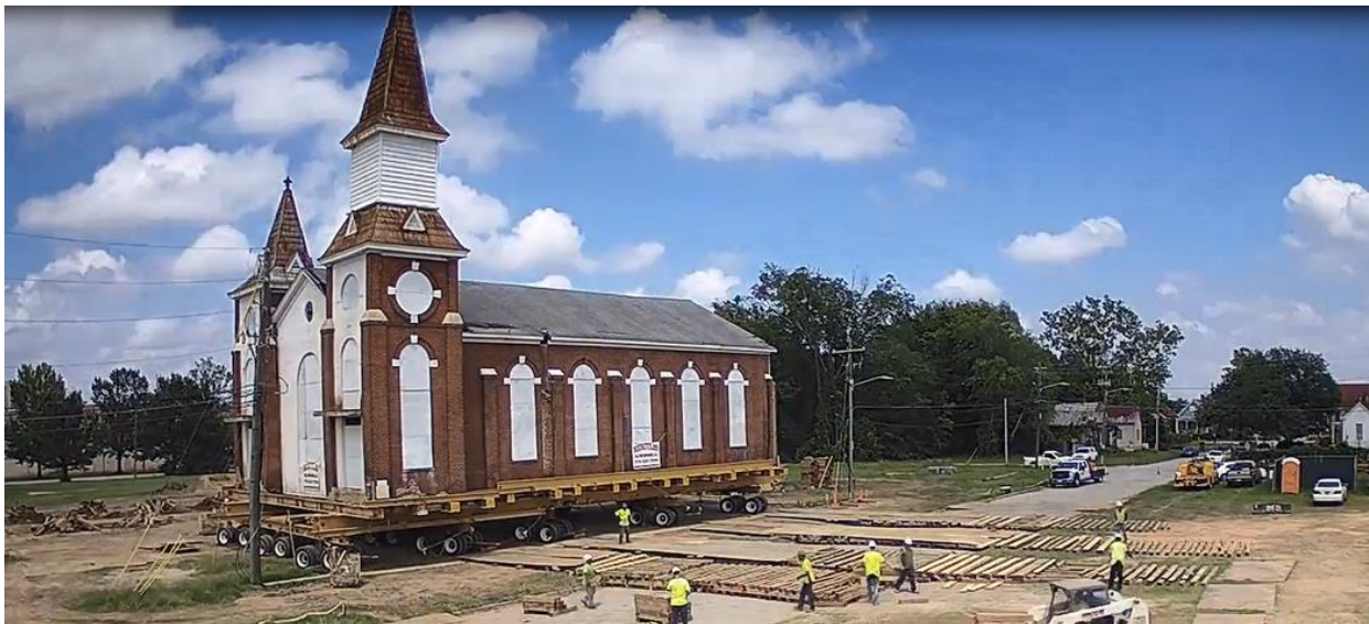
Augusta MGP Site, HSI 10132, Richmond County. As part of a lengthy historic Manufactured Gas Plant cleanup, Atlanta Gas Light worked with the community to relocate the former Trinity CME church, allowing extensive remediation to occur in FY20.
