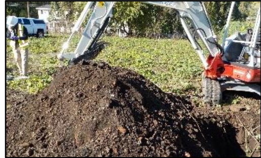
Excavation of soil contaminated by lead. Westside Atl.
