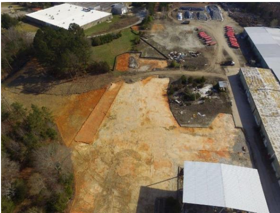
Excavated area of contaminated soil by facility building
