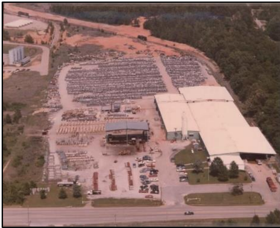
Martin Fireproofing during operations, Elbert County
