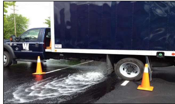
Figure 2 Meter testing via truck mounted apparatus
