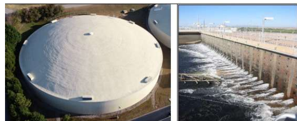
Figure 4 Reservoir or clearwell adjacent to a water treatment plant
