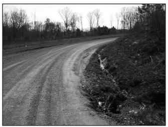
Problem: culvert is blocked with debris; ditch grade too steep. Fixes: clean culvert; line culvert inlet with stone; use rock check dams for grade control. *Photo: Courtesy of Limestone Valley RC&D Council*
