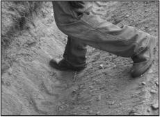
Final shape of roll ditch is a rounded U-shape. This is a better design shape to distribute and reduce water's erosive energy. Ditch needs to be revegetated.
