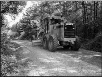
Blading to move surface materials; note slight tilt of front wheels. *Photo: Courtesy of Two Rivers RC&D Council*
