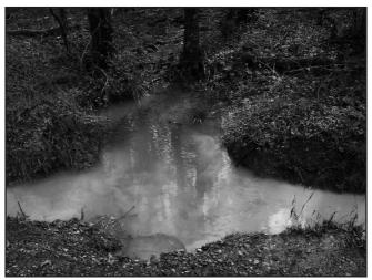
Problem: ditch grade too flat. Fix: re-grade ditch (during dry weather). Photo: Courtesy of Limestone Valley RC&D Council
