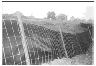
Example of type "C" sediment barrier silt fence (Sd1-C). Note that the fence is slightly angled into the direction of runoff. *Source: Field Manual for Erosion and Sediment Control in Georgia, GSWCC*
