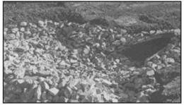
Example of outlet protection rock apron. Source: Manual for Erosion and Sediment Control in Georgia, GSWCC
