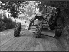
Using wheel for "shaping and tamping" ditch; creates a "roll" or "rounded U" shape ditch. Meriwether County, Georgia *Photo: Courtesy of Two Rivers RC&D Council*
