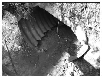
Problem: corroded metal pipe. Fix: replace with corrosive-resistant pipe. Photo: Courtesy of Two Rivers RC&D Council
