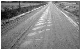
This distortion was cut into the road surface by operating motor grader too fast. The angle of depressions matches the angle of the moldboard.
