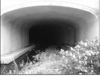
Example of bottomless culvert; note natural bottom material remains exposed. Cherokee County, Georgia *Photo: Courtesy of GDOT*
