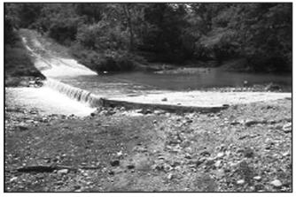
Example of concrete low-water crossing; note downstream edge is protected from scouring with riprap or gabions. *Source: USDA Forest Service*
