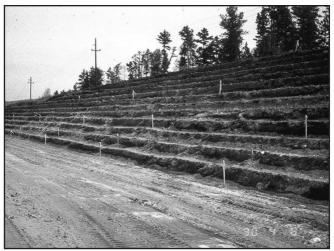
Example of terraced slope. Photo: Courtesy of GDOT
