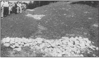
Example of check dams (Cd) in concentrated ditch flow. Source: Manual for Erosion and Sediment Control in Georgia, GSWCC
