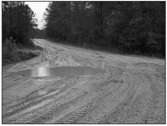
Poor drainage causing weak sub-grade and road surface from vehicle weights during "dry" periods. *Photo: Courtesy of Two Rivers RC&D Council*
