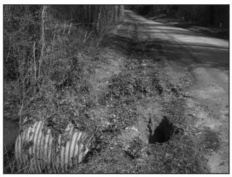
Problem: water erosion around pipe; poor installation with fill. Fix: reset pipe with proper bedding material and compaction. *Photo: Courtesy of Two Rivers RC&D Council*
