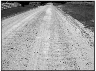
Road surface ravelling; coarse aggregates worn away by traffic. *Photo: Courtesy of Two Rivers RC&D Council*
