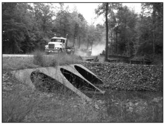
Example of rock filter dam (Rd) installed at drainage ditch outlet to live stream. Harris County, Georgia *Photo: Courtesy of Two Rivers RC&D Council*
