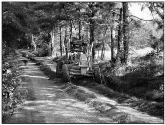
Example of "pulling" ditch and re-establishing crown. Monroe County, Georgia Photo: Courtesy of Two Rivers RC&D Council **Description:** An area of maintenance concern where roads meet
