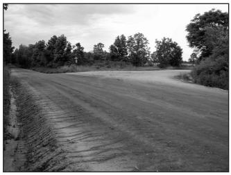
Lignin sulfate application; treated area "darker" than side road.
