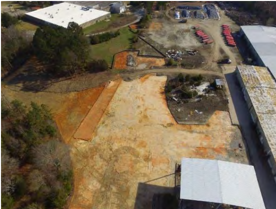
Excavated area of contaminated soil by facility building
