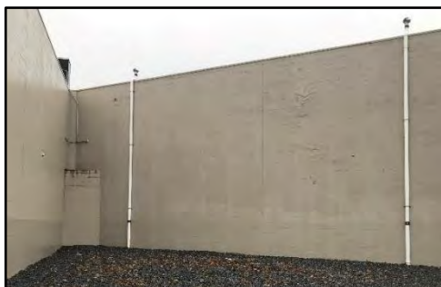
Vapor intrusion remediation system installation, Fulton County
