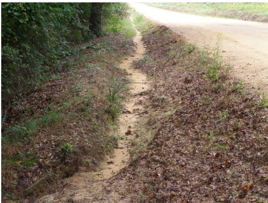
Water travelling down long slopes erodes the ditch bank and carries sediment to the outlet.
