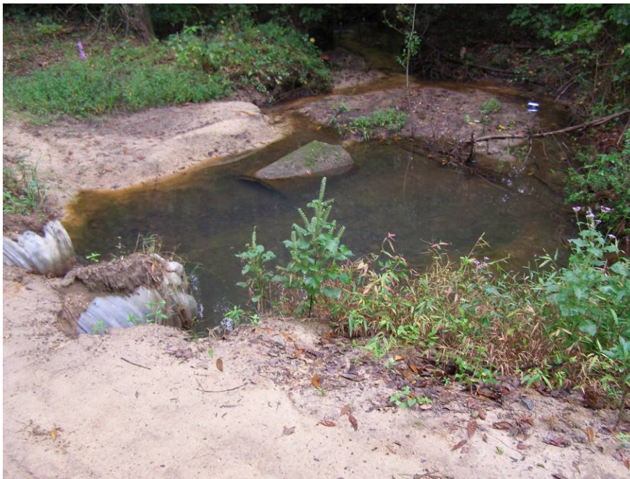
Poor outlet protection causing erosion, sedimentation and pipe failure.
