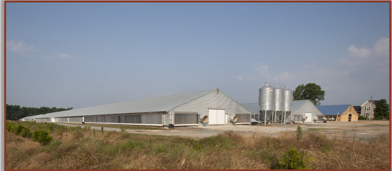
Figure 4.2.a. There are many poultry operations within the Holly Creek Watershed. None, however, exceed the capacity threshold that requires NPDES permits.
