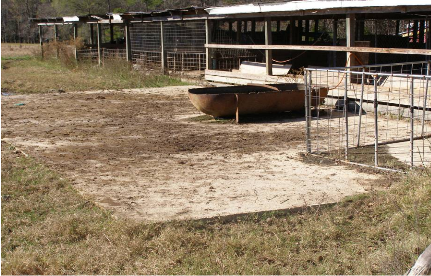
Livestock watering facility to meet water requirements and get livestock out of the stream.
