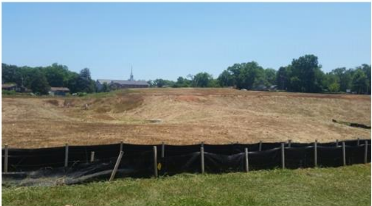
Best management practices implemented at construction site on E 10th Street in West Point 5/28/19
