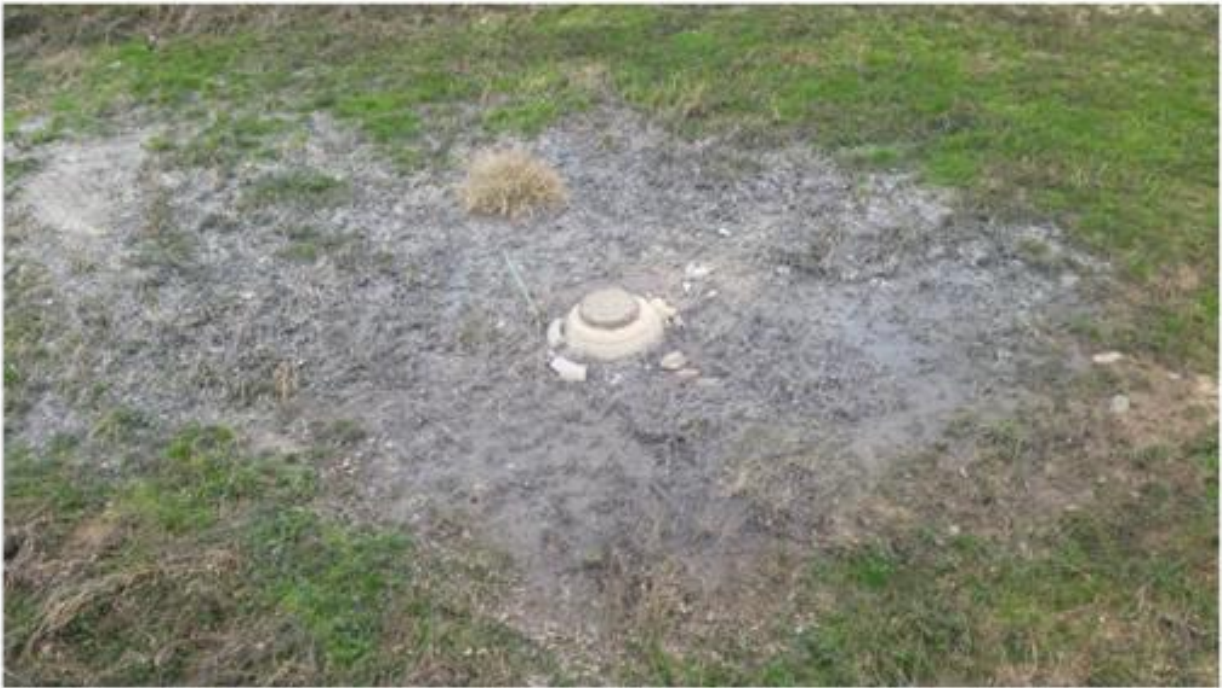
Sewage spill on Old West Point Road at Long Cane Creek resulting from pump failure at lift station and damaged manhole (Site 10) 2/27/19
