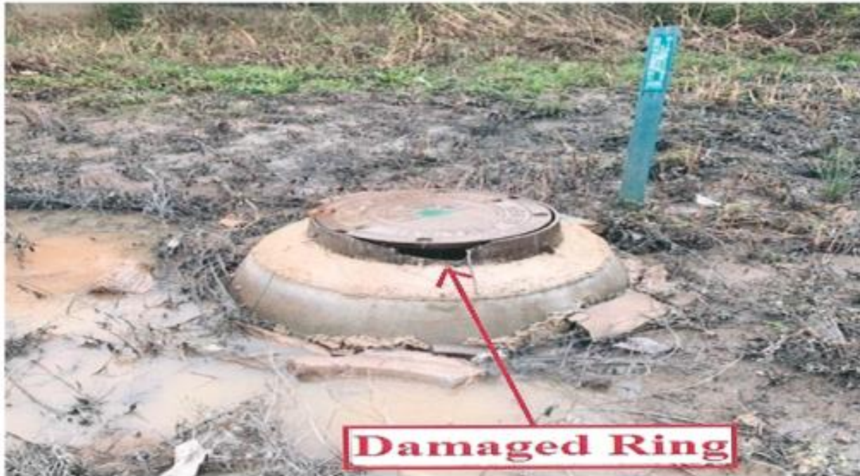
Damaged manhole at sewage spill location on Old West Point Road at Long Cane Creek (Site 10)
