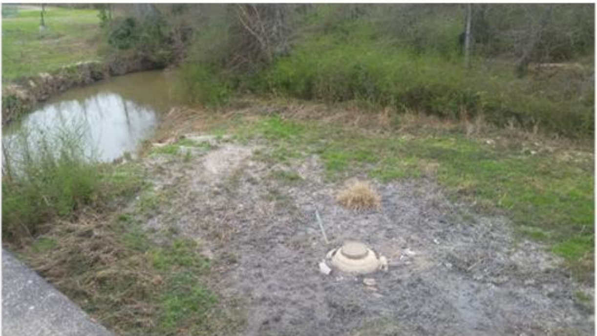
Sewage spill on Old West Point Road at Long Cane Creek resulting from pump failure at lift station and damaged manhole (Site 10) 2/27/19
