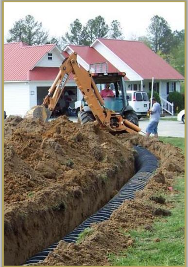
Figure 6.2.b. A septic system repair can reduce the fecal coliform load in streams. A cost-share program can help incentivize costly repairs.
