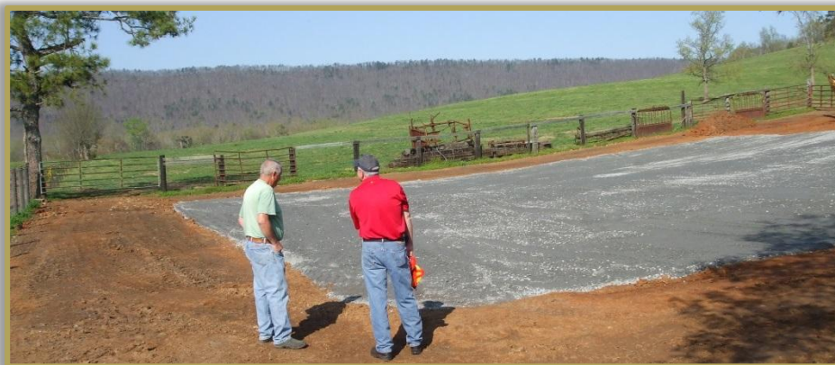
Figure 6.2.a. Constructing heavy use area pads for cattle feeding or watering areas can reduce erosion and sediment loads in the watershed.
