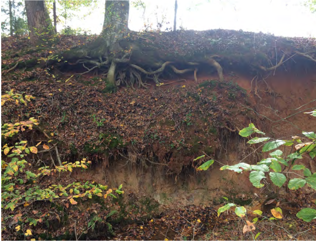
Bank erosion due to stormwater runoff. Eroded bank is 15' - 20' high.
