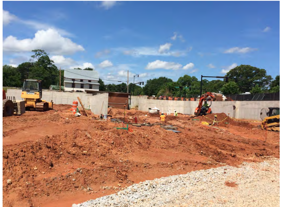
Construction activity at Indian Creek headwaters.
