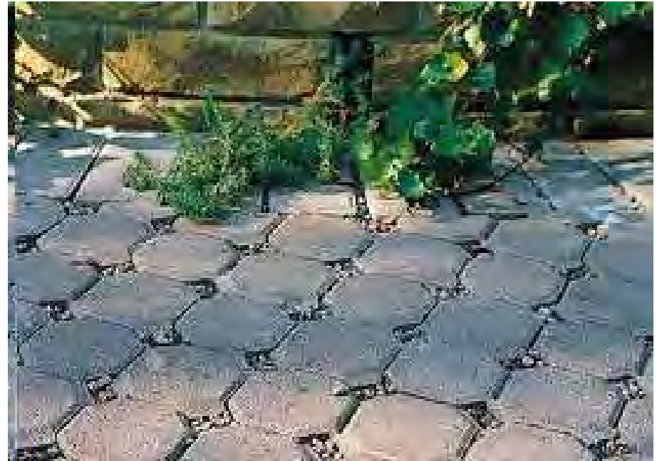
Permeable Pavement System (sidewalk)
