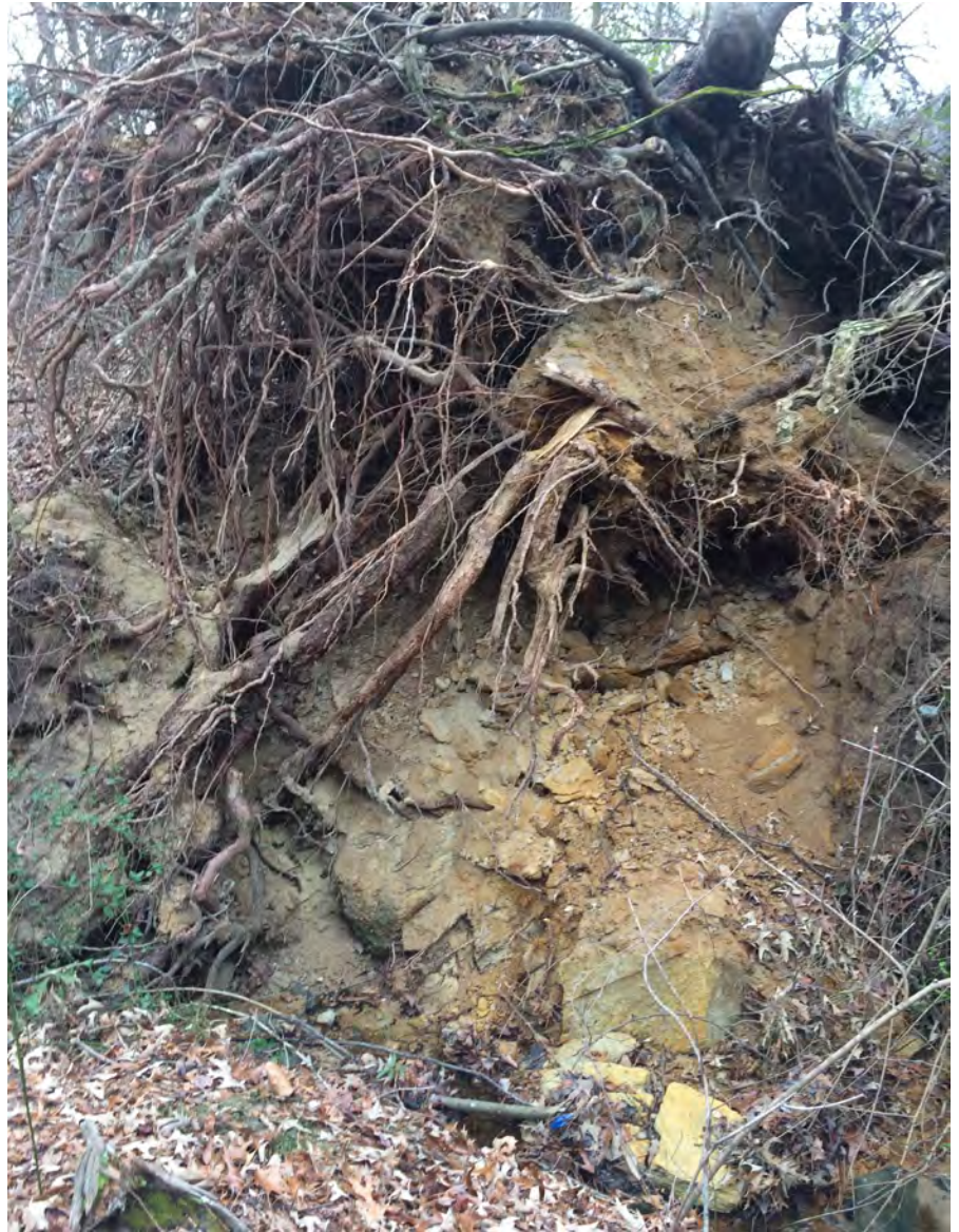
Stream bank "blow out" from stormwater. Eroded bank is about 10' high.
