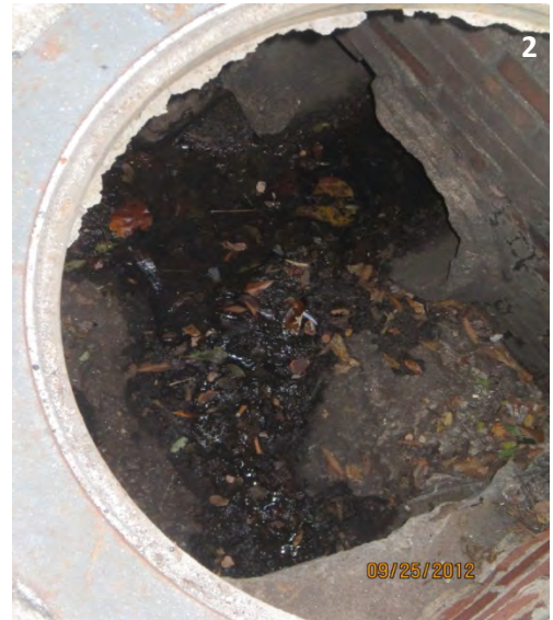
Figure 8b. Flow in dry weather in a stormwater pipe suggests sewage leak
