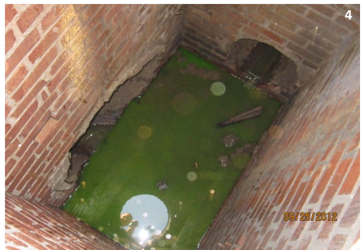
Figure 8d. Green dye is flushed down the toilet of a nearby business, helping hone exact location of leak
