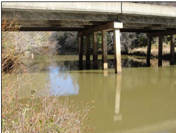
Pataula Creek under Hwy 82 bridge.
