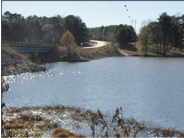
Pataula Creek and Hwy 39.
