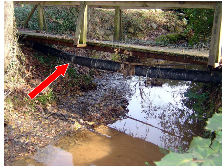
Damaged Sanitary Sewer Pipe on Springer Drive
