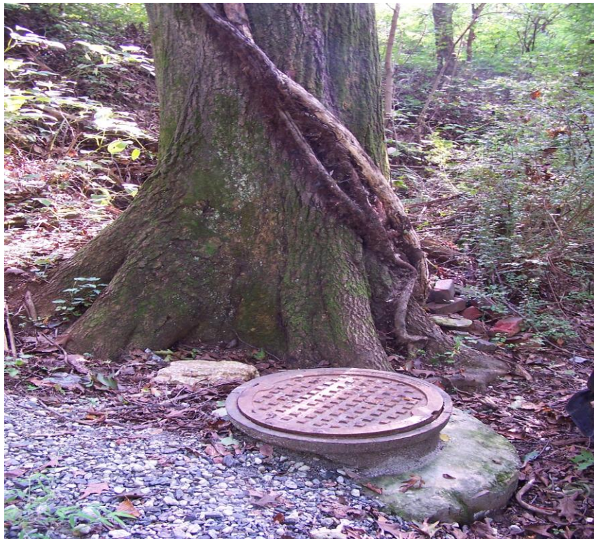
Figure 53. Tree growing immediately next to sanitary sewer manhole and rights-of-way
