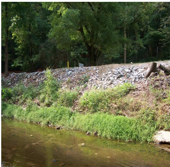
Figure 33. View of rip-rap and access road next to Proctor Creek
