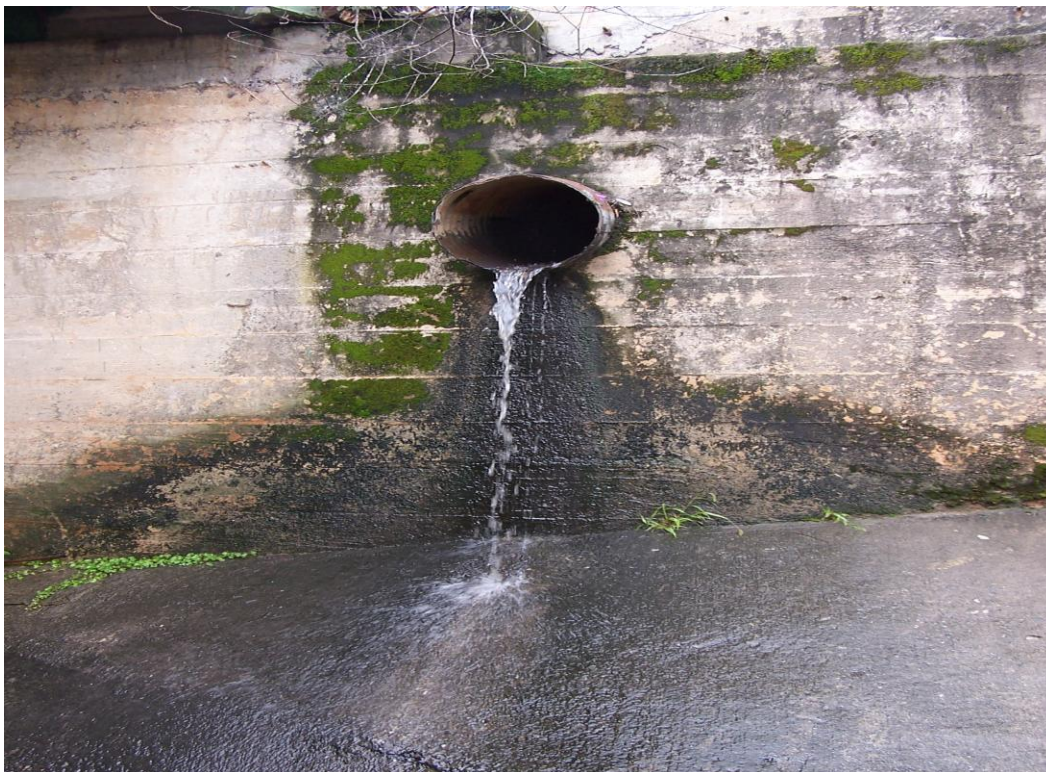
Figure 50. Flowing pipe with soapy smell below Simpson Rd.
