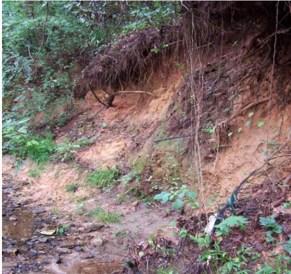
Figure 11. Bank failure
