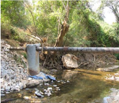
Replaced sanitary sewer crossing downstream of Johnson Rd.
