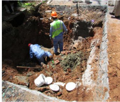
City of Atlanta Crew repairing broken sewer and storm lines
