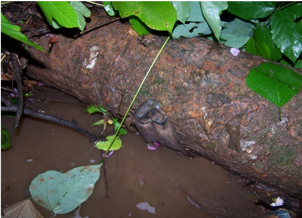
Figure 51. Ductile iron pipe with rubber plug crossing Proctor Creek in headwaters above Interstate 20
