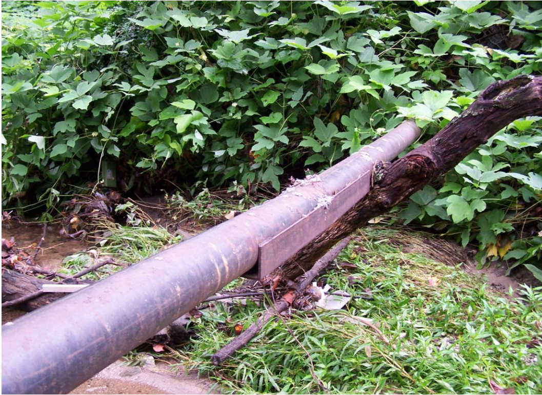
Figure 52. Repaired and braced sanitary sewer line crossing Proctor Creek
