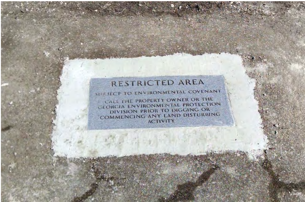
Photograph 5-2: AOC-2 monument installation
