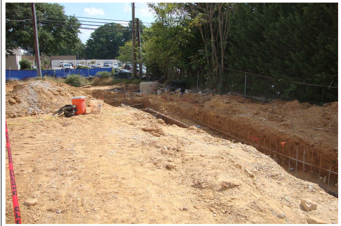
Photo 5. View east along excavation for retaining wall footings along southern property boundary.
