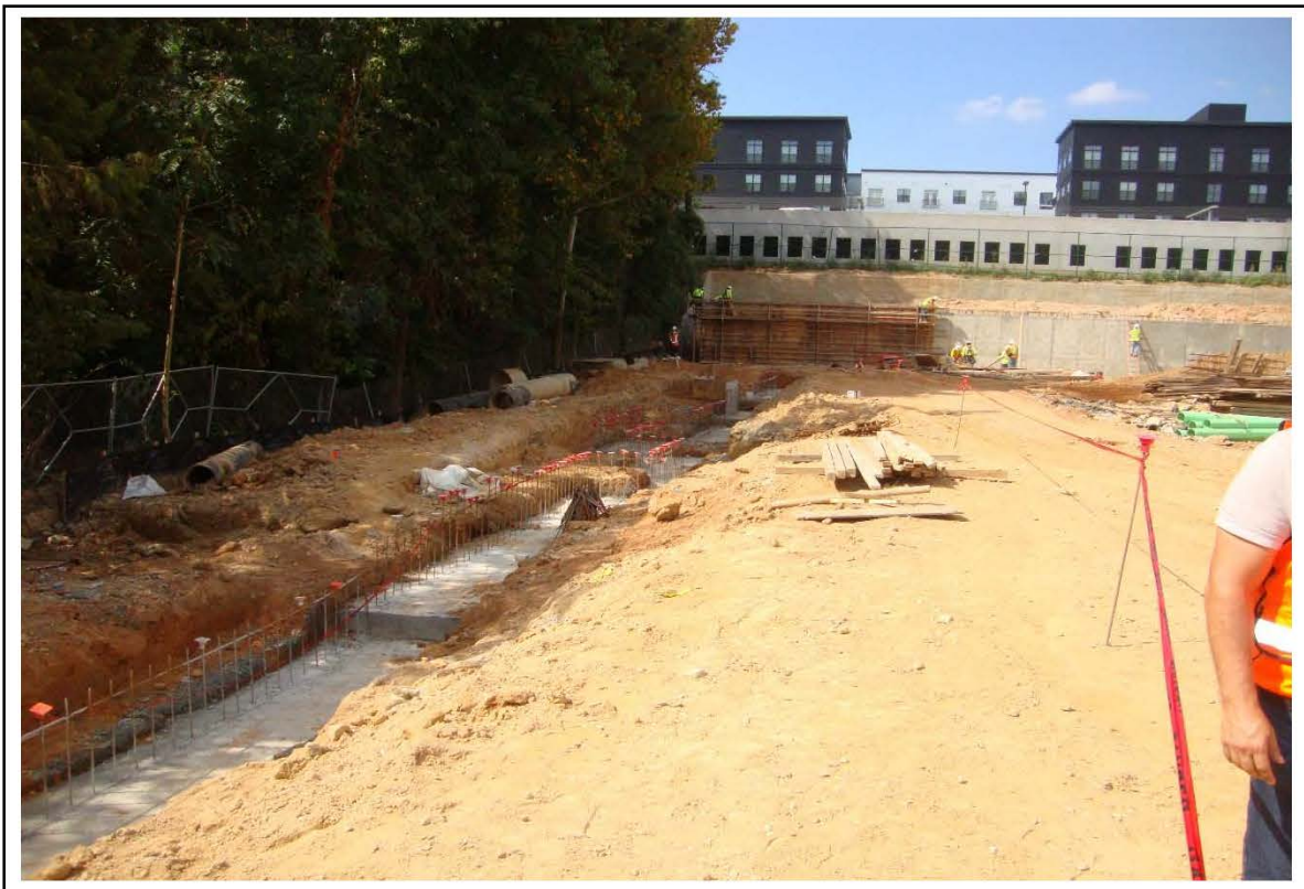
Photo 4. View west along excavation for retaining wall footings along southern property boundary.
