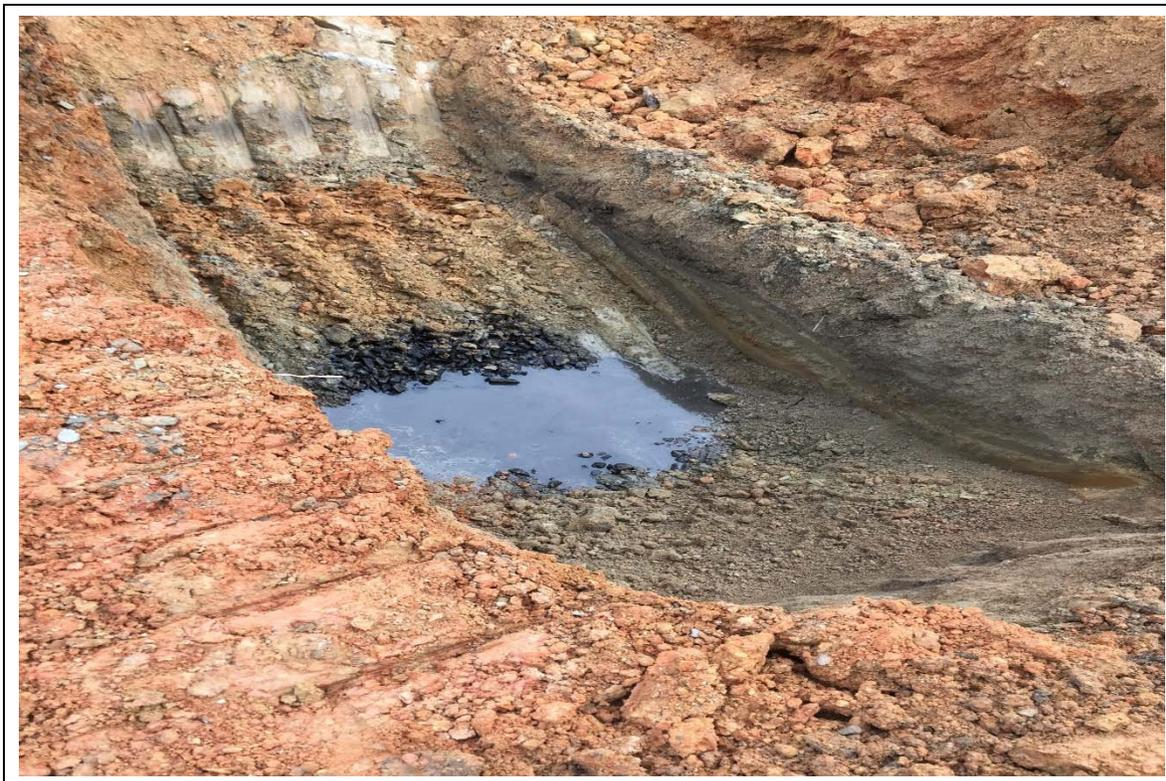
Photo 3. Groundwater in bottom of suspect mechanic's pit excavation following removal (12/19/17).
