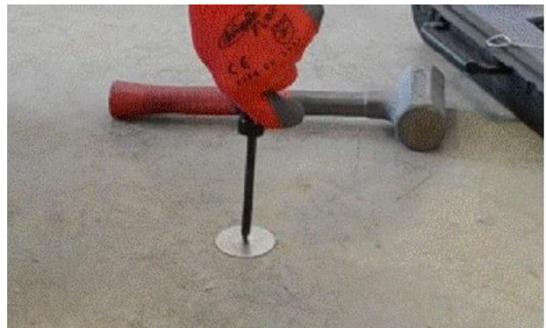
Figure 5. Tightening the Secured Cover
