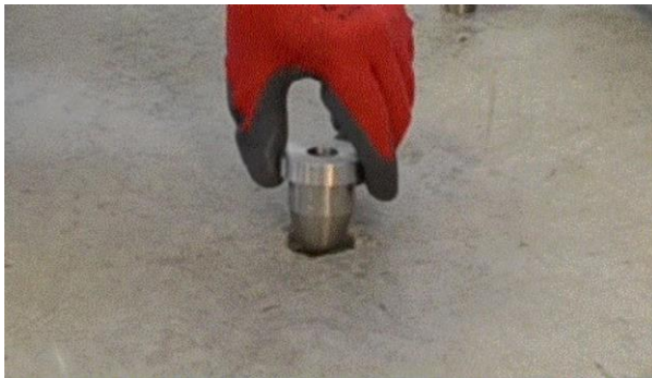
Figure 3. Testing Depth with the Drilling Guide
