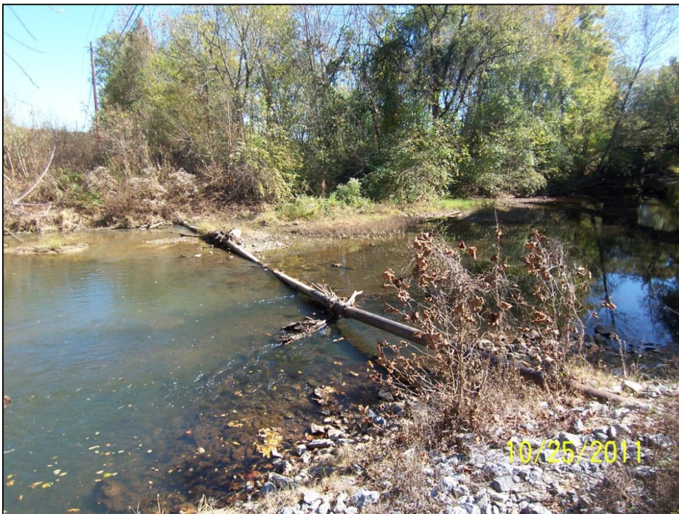
Figure 16. Old Sanitary Sewer Line in Pumpkinvine Creek
