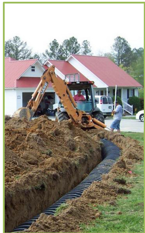
Figure 6.1.b. Septic system repairs can reduce fecal coliform loads.
