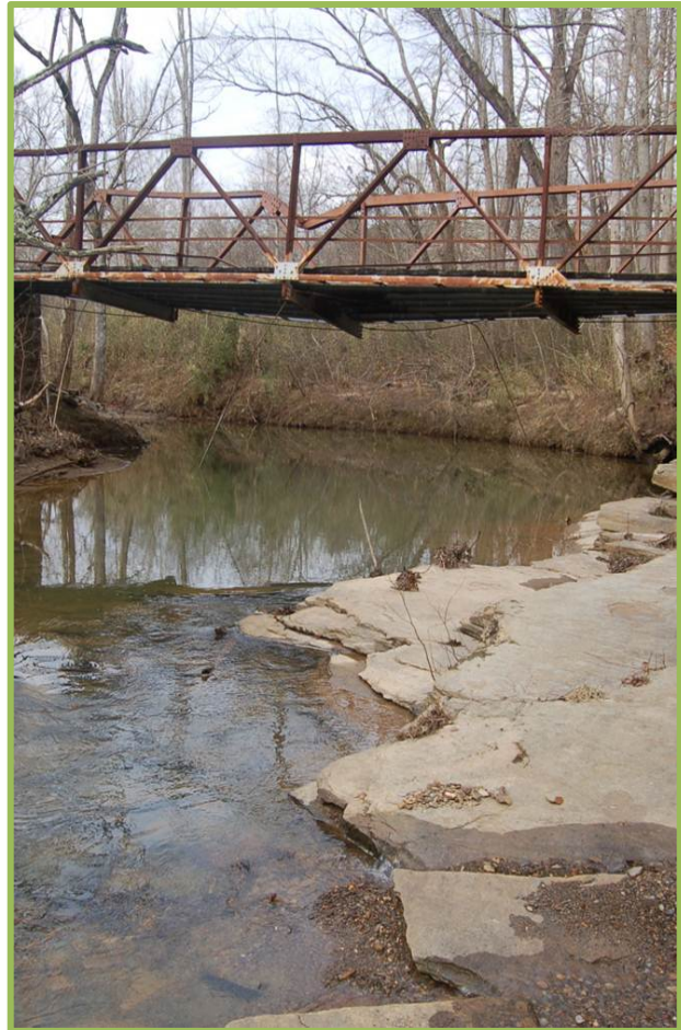
Figure 1.1.a. A historical bridge spanning Salacoa Creek in Cherokee County.
