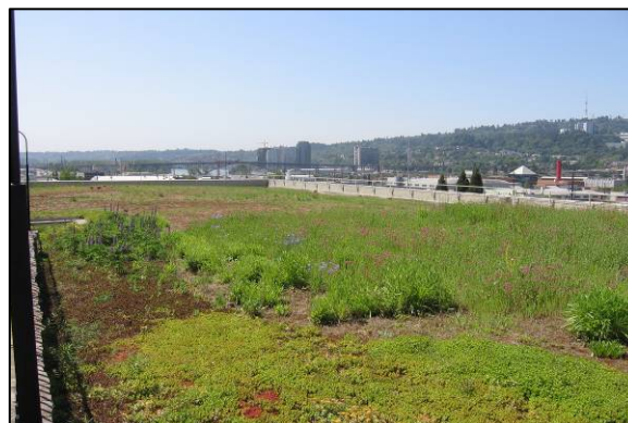
Figure 6.12: Green Roof Used in Place of a Traditional Impervious Rooftop (Source: Center for Watershed Protection)
