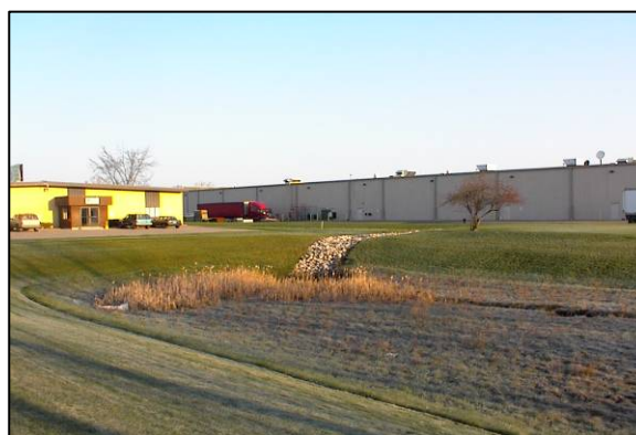
Figure 6.20: Dry Detention Basin Used to Provide Water Quantity Management (Source: Center for Watershed Protection)
