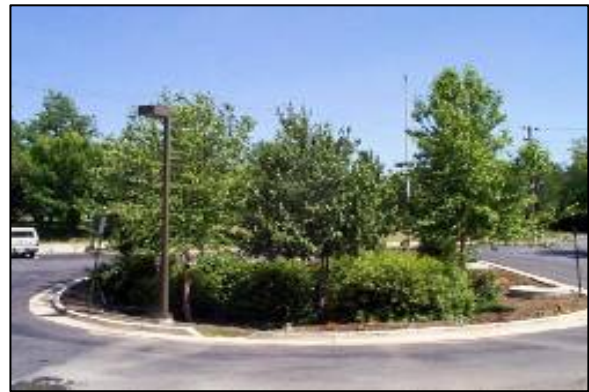
Figure 6.17: Bioretention Area (Source: Center for Watershed Protection)
