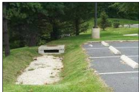
Figure 6.18: Infiltration Trench (Source: Center for Watershed Protection)
