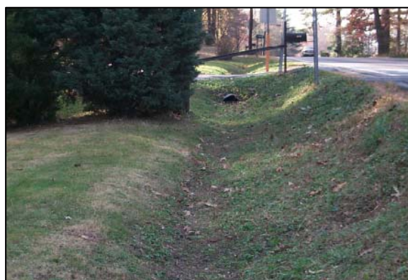
Figure 7.33: Grass Channel Along a Local Roadway (Source: Atlanta Regional Commission, 2001)
