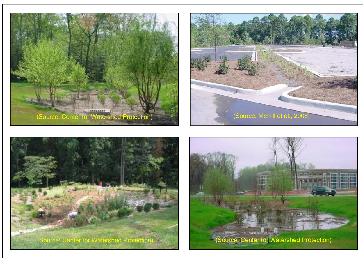
Figure 8.19: Various Bioretention Areas
