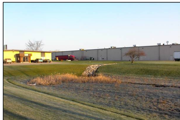
Figure 8.6: Dry Detention Basin Used to Provide Water Quantity Management (Source: Center for Watershed Protection)
