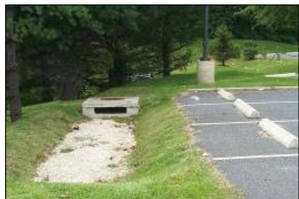
Figure 8.4: Infiltration Trench (Source: Center for Watershed Protection)
