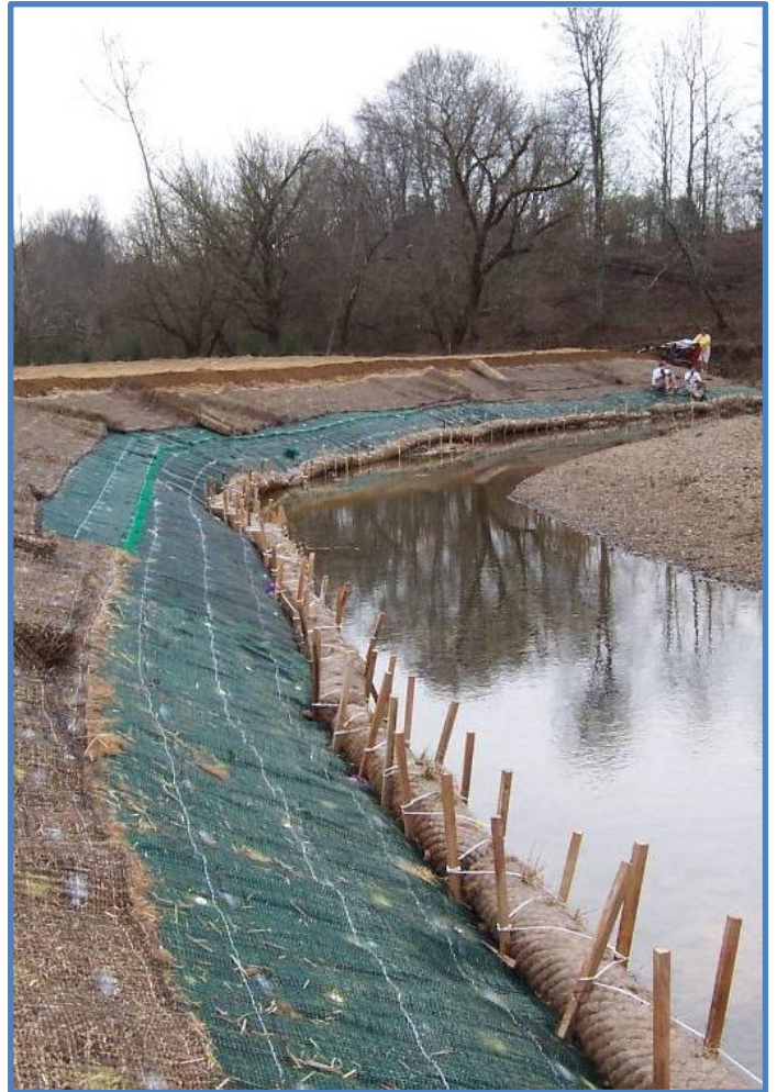
Figure 5.1.a. Streambank stabilization is an important restoration technique where eroding banks contribute to the stream's sediment load.
