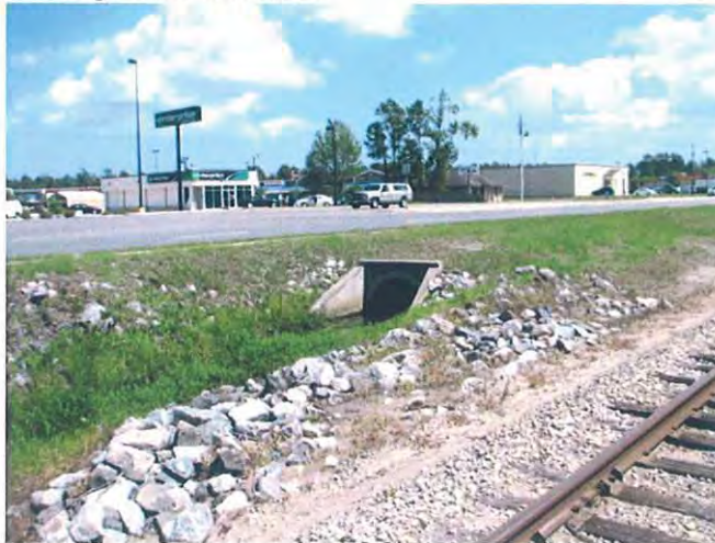
Drainage Southside GA 40 Across from Wal-Mart
