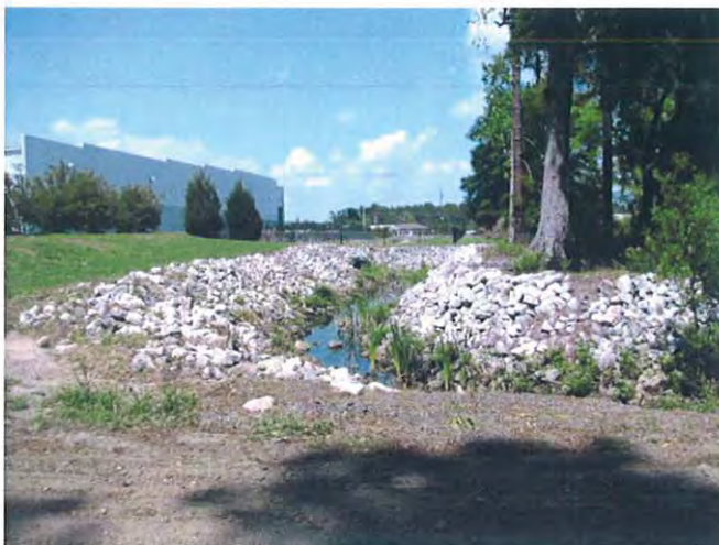
Upper Miller's Branch – Lowes Store Drainage
