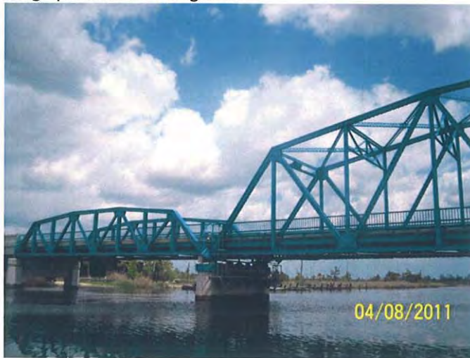
US Highway 17 Bridge and Boat Launch
