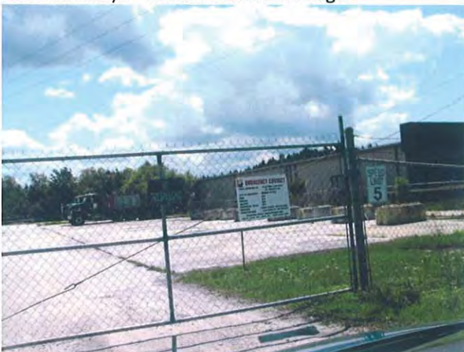
Looking West Cement Plant in St. Marys – Miller's Branch Drainage
