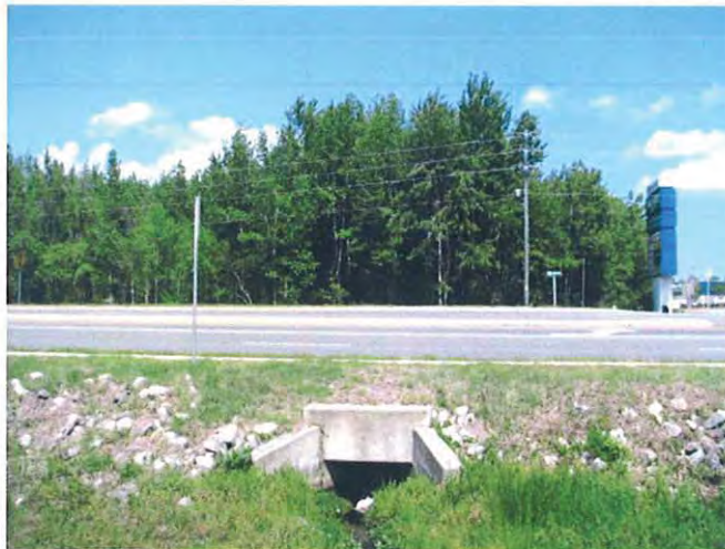
Drainage under GA 40 from Wal-Mart
