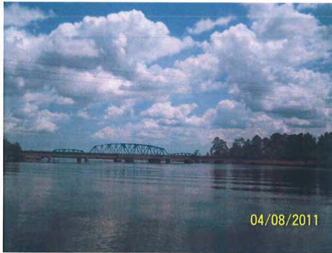
Highway 17 and Rail Road Bridge up river from segment
