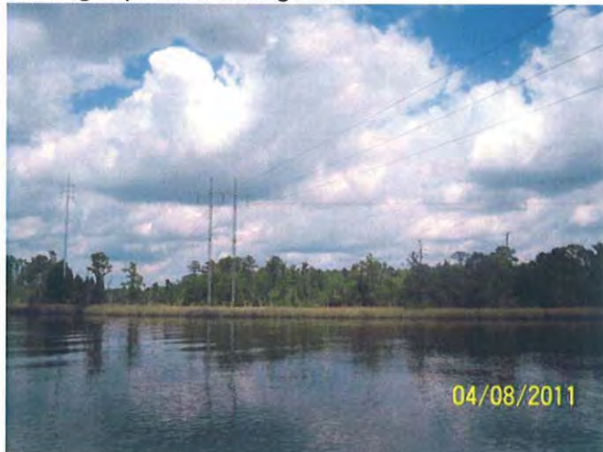
Transmission Lines crossing upstream from segment
