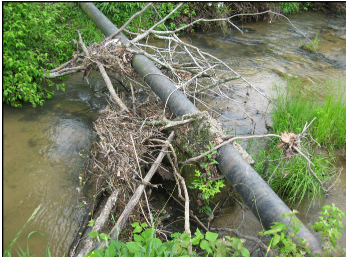
Problematic sewage lines cross Scott Creek, oftentimes leading to flotsam and debris jams on the infrastructure.
