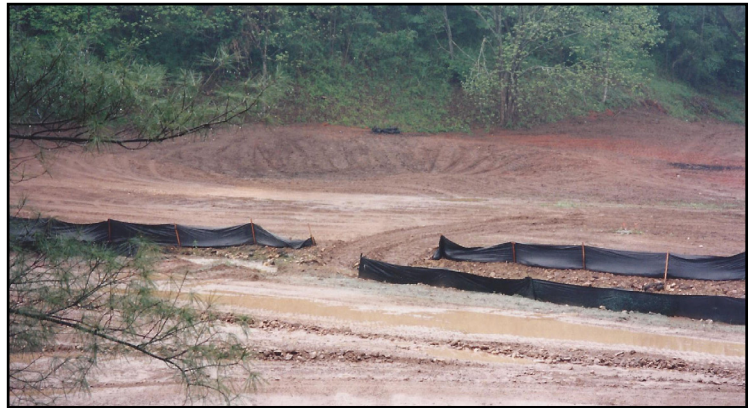
The absence or improper design of BMPs during reconstruction of the Kingwood golf course caused a massive amount of dirt to wash into Chechero Creek, and evidence of this remains today.
