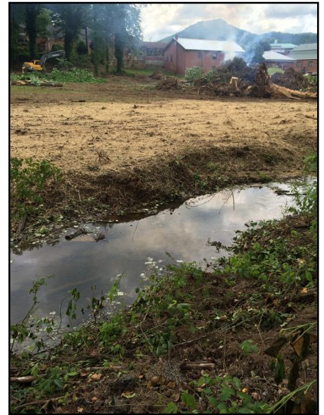
Ginger Creek, tributary to Scott Creek, shows a lack of BMPs in its stream buffer zone as illustrated by this recent clearing operation.
