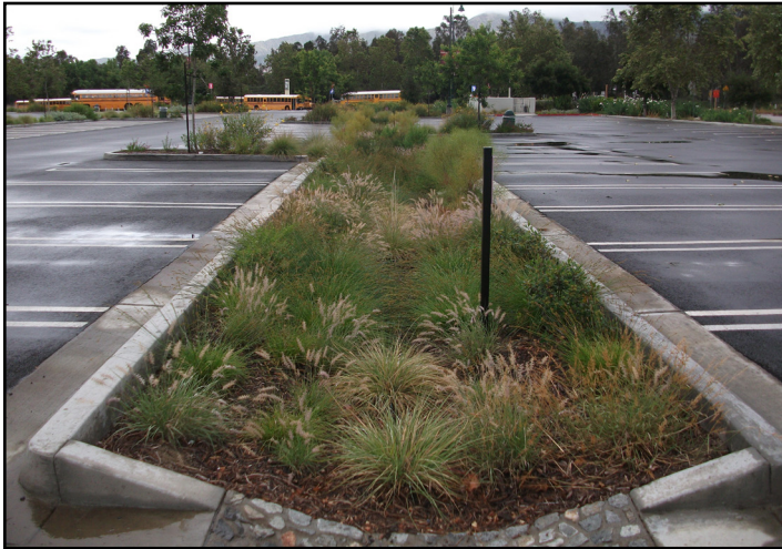
A parking lot bioswale can control and naturally filter parking lot stormwater runoff.
