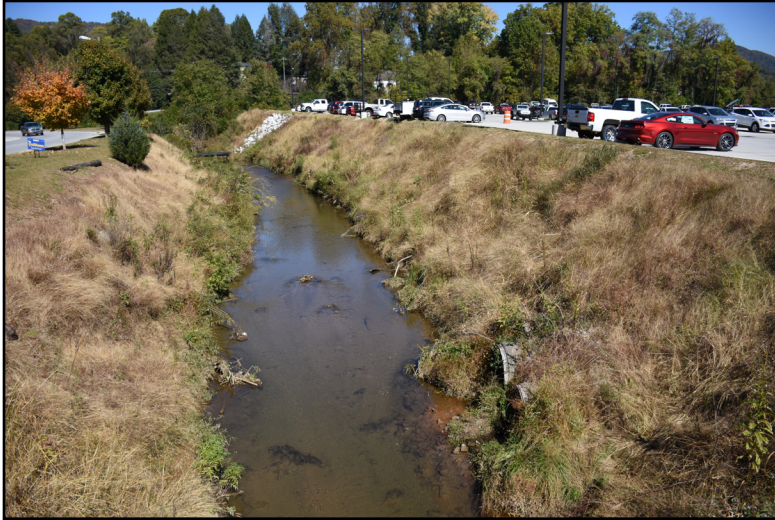
In Clayton, sections of Stekoa Creek have undergone hydromodification that includes channelizing and confining the stream within rip-rap embankments.
