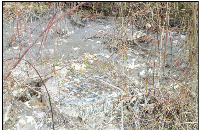
A sewer manhole overflow into Coffee Branch, a tributary to Stekoa Creek, contributes to the bacteria load in Stekoa Creek.
