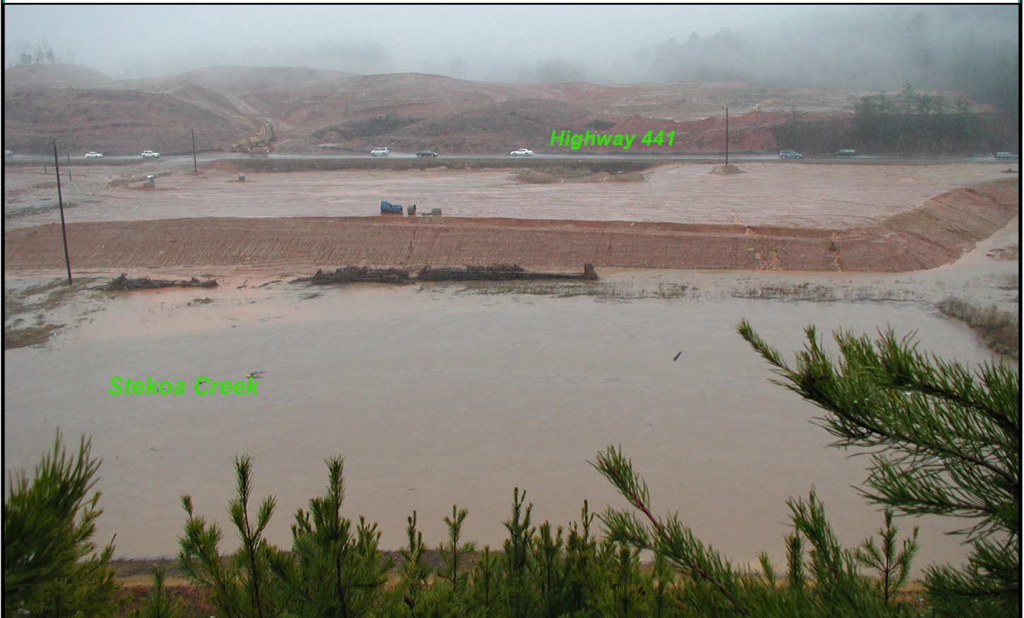
In 2004, the steep topography on the east side of Highway 441 was leveled to make a flat spot for development, and the dirt was used for filling a portion of Stekoa Creek’s floodplain, putting a massive amount of dirt into the creek.
