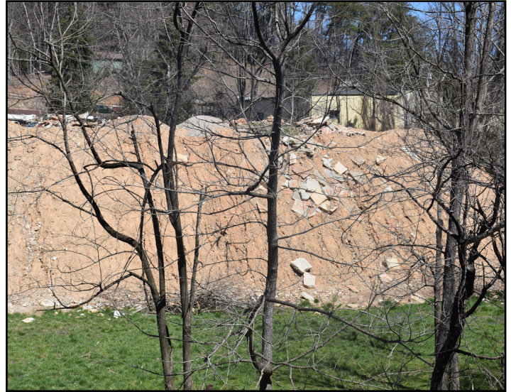
Filling at this site next to Coffee Branch, a tributary to Stekoa Creek, lacks BMPs for stopping erosion into the stream.
