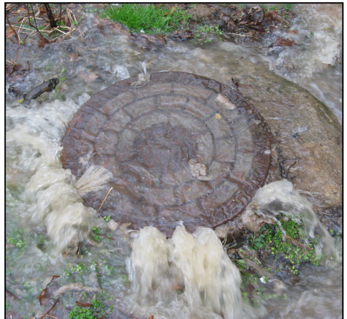
Stormwater infiltration has caused numerous sewage spills into Scott Creek, a tributary to Stekoa Creek.
