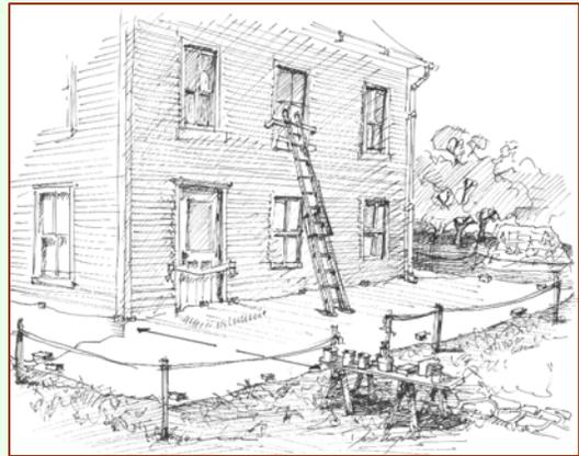
In situations, such as where work areas are in close proximity to other buildings, or under windy conditions, the renovation firm must take extra precautions in containing the dust and paint debris. Vertical containment may be necessary to containing the dust and paint debris in the work area.
