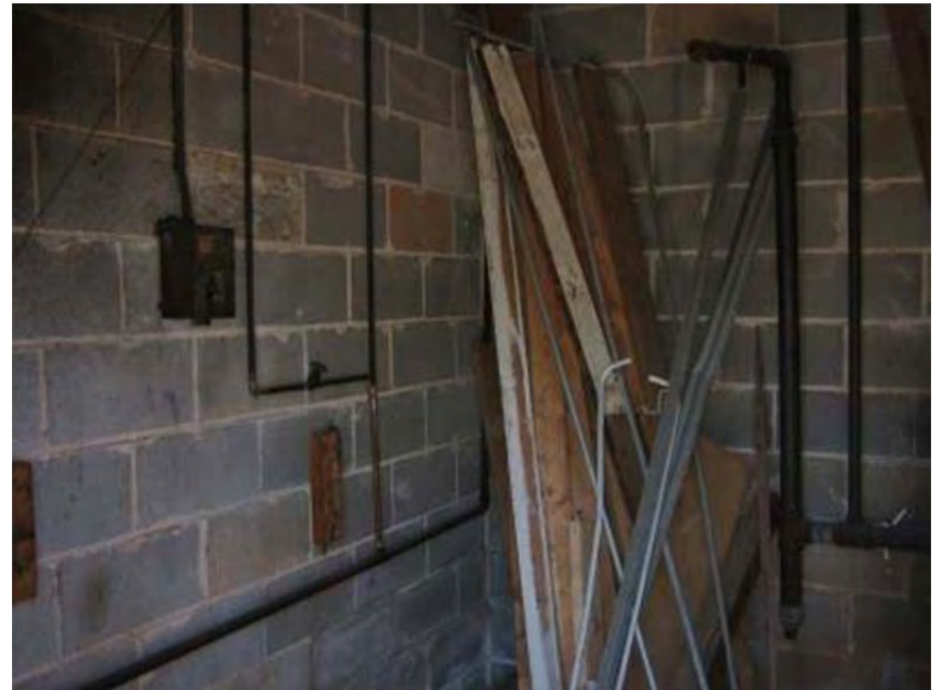
Photo 8: Exterior room attached to drycleaner.
