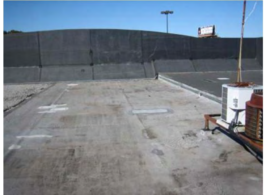
Photo 2: Non-ACM roof of the nail salon.
