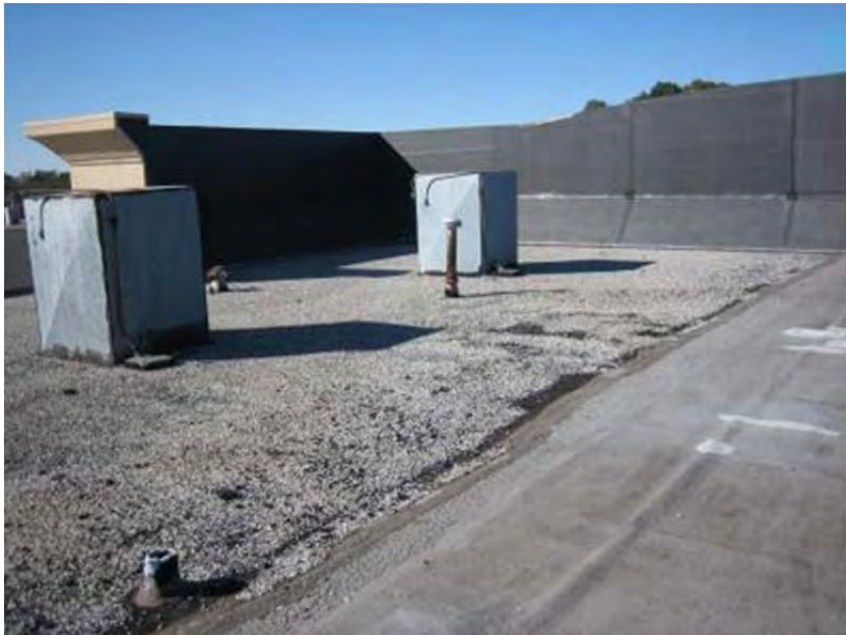
Photo 3: Non-ACM roof of the drycleaner.
