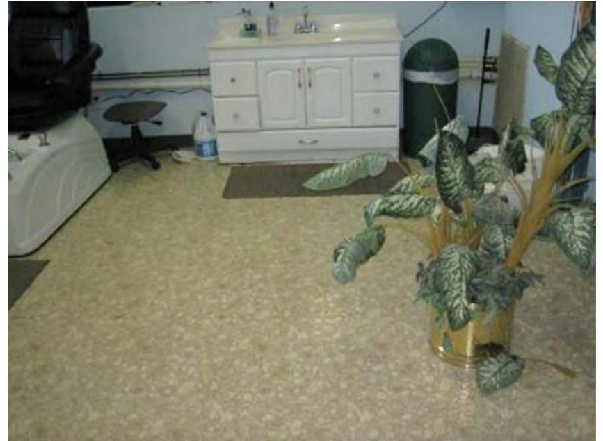
Photo 10: Yellow and white sheet flooring in nail salon, black mastic associated with sheet flooring is ACM.
