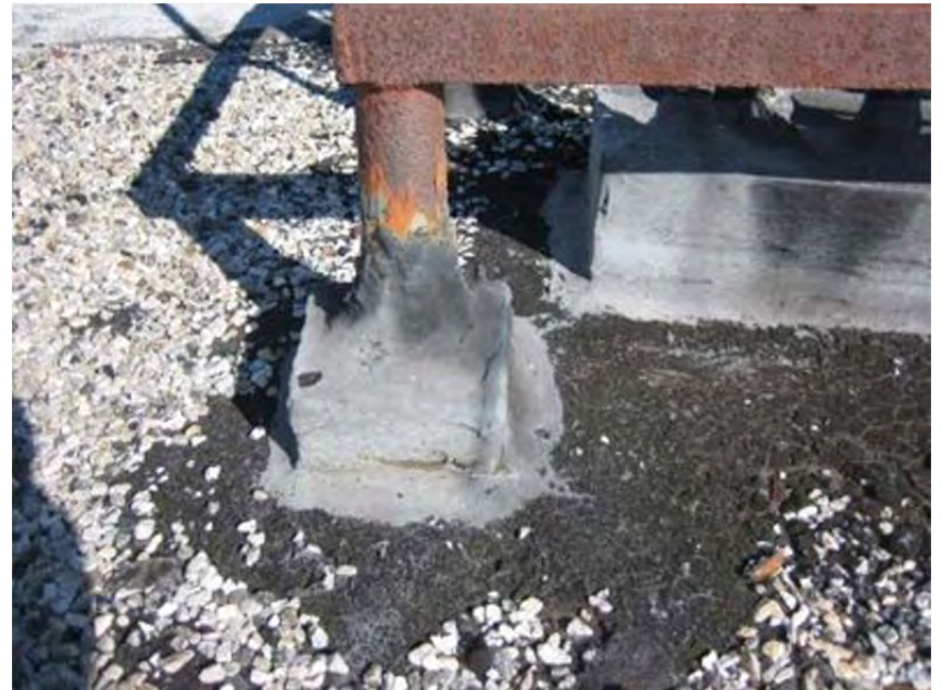
Photo 4: Non-ACM roof tar.
