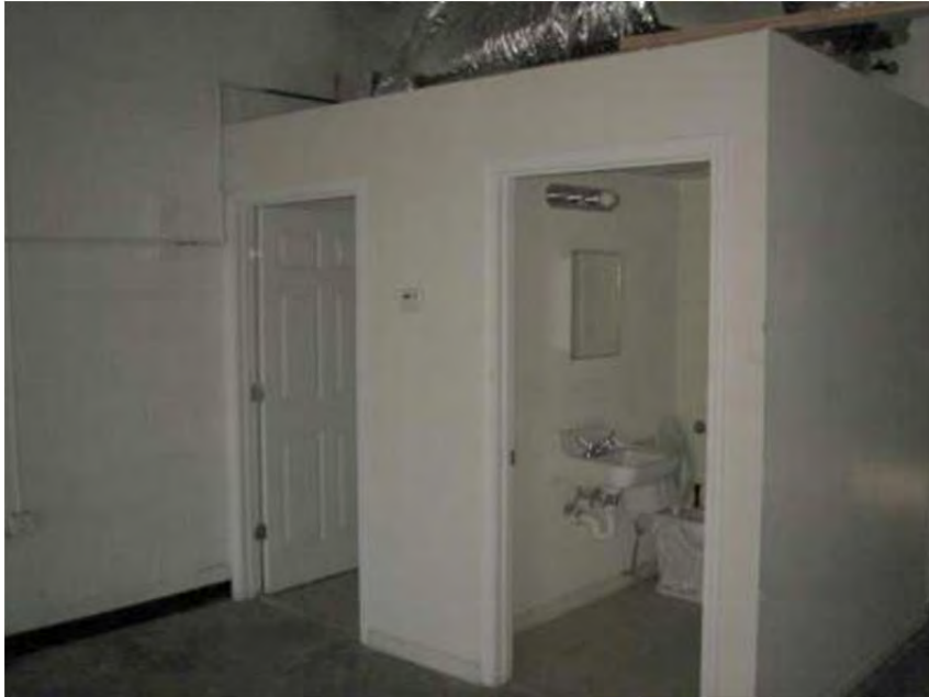
Photo 5: Interior of the drycleaners, drywall walls are non-ACM.
