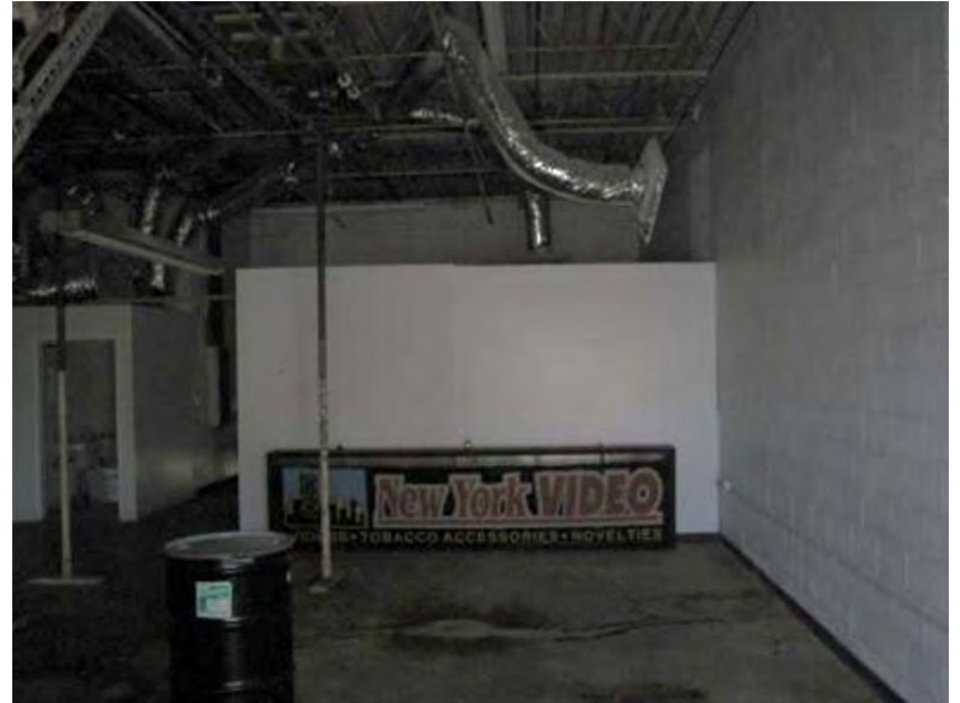
Photo 6: Interior of the drycleaners, drywall walls are non-ACM.
