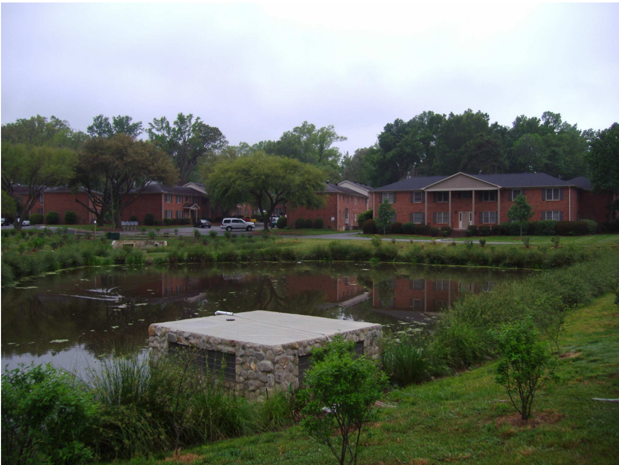
Figure 18. Detention pond retrofit with new forebay and vegetated shelf
