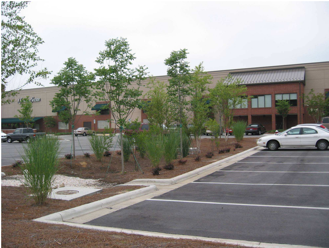
Figure 16. Bioretention cell located in a shopping center
