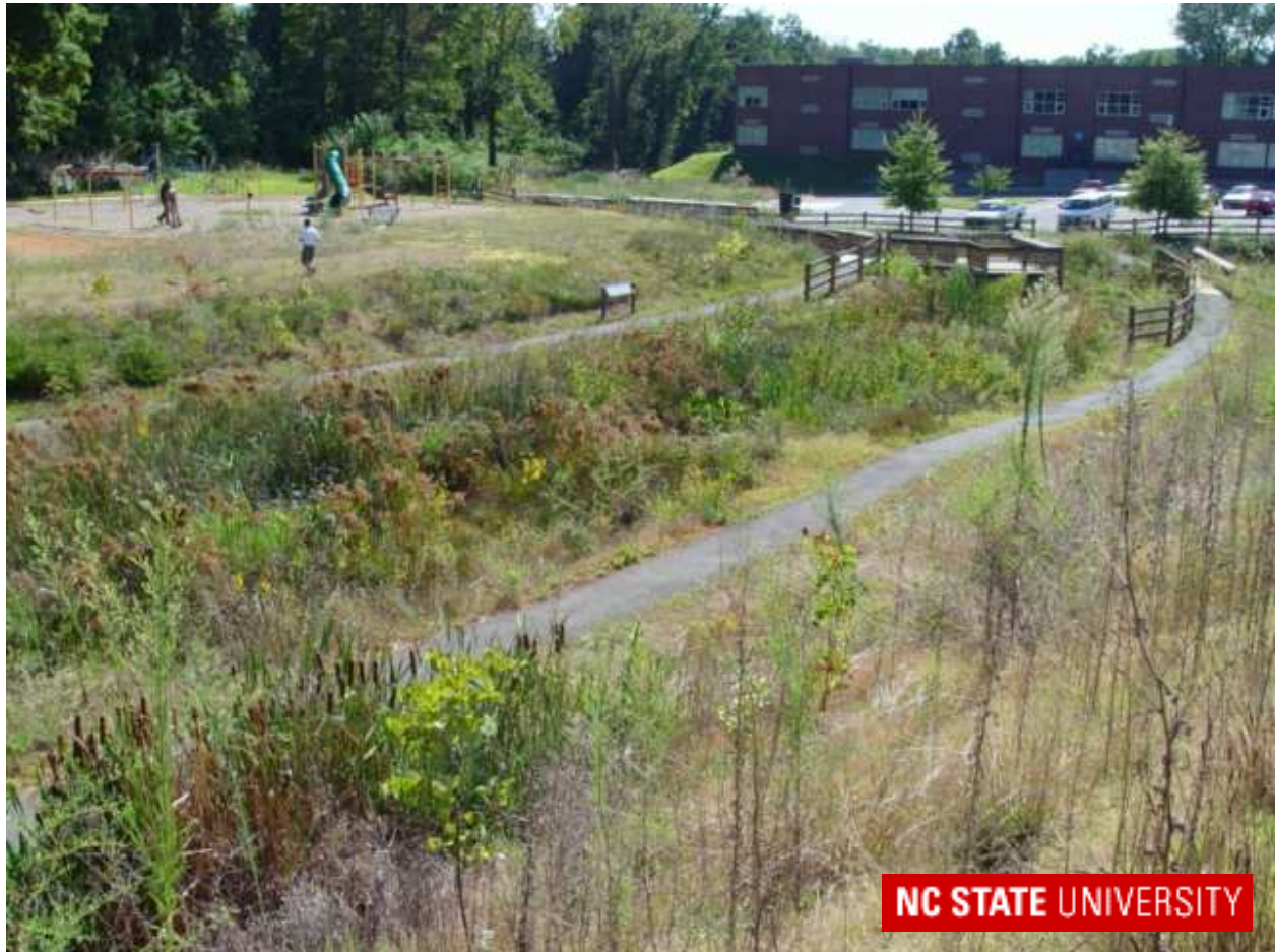
Figure 17. Stormwater wetland at an elementary school
