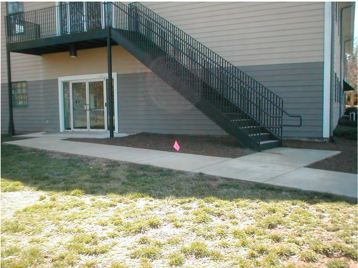
Plate 6: View – South. Shallow soil sample HA5 (1-2) (pink flag) was located near the northwest corner of the former Bibb Mill “Dye House”. March 6, 2008.
