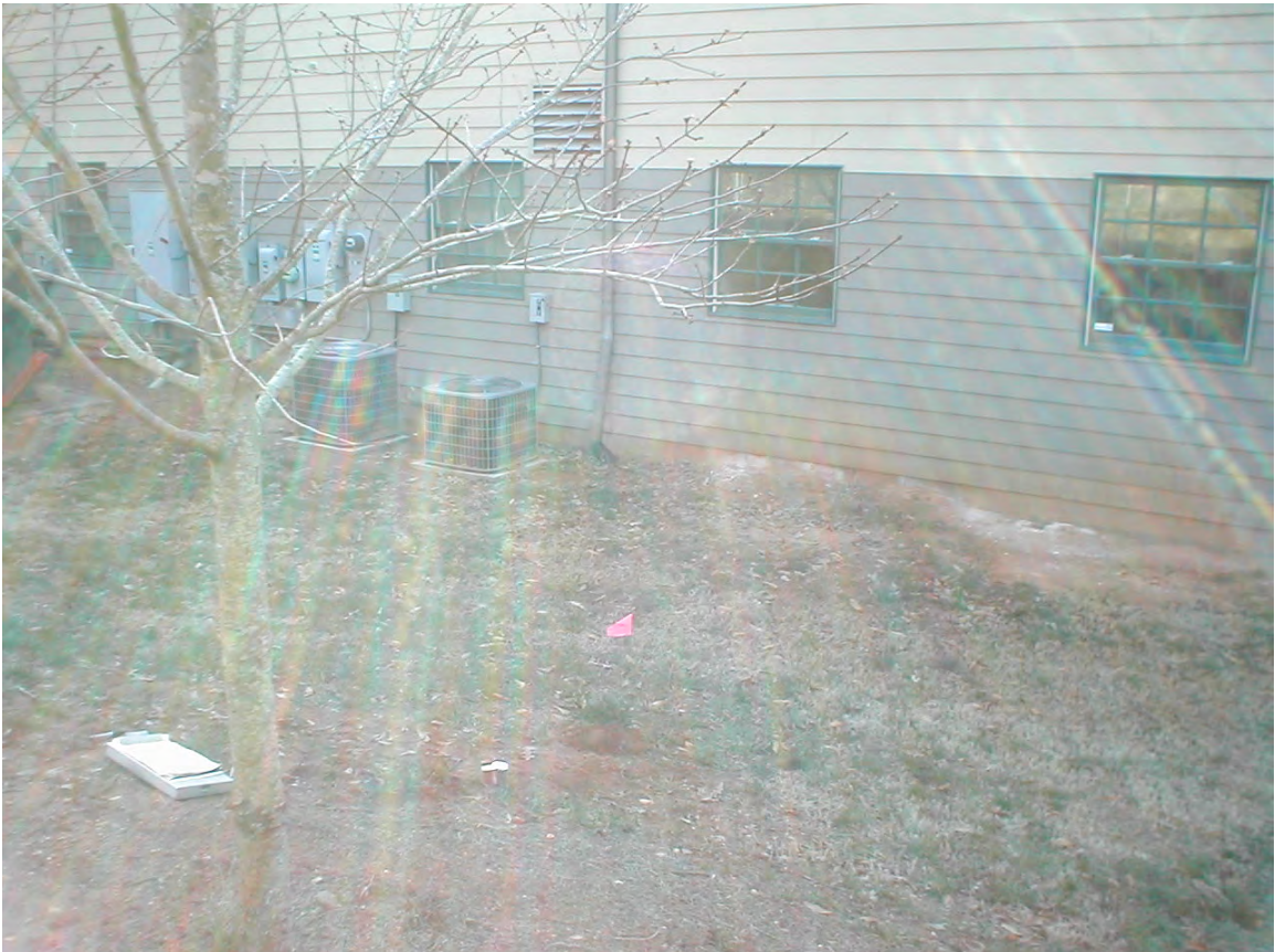
Plate 14: View – Southwest. Shallow soil sample HA14 (1-2) (pink flag) was located along the east side of the former Bibb Mill “Dye House”. March 6, 2008.
