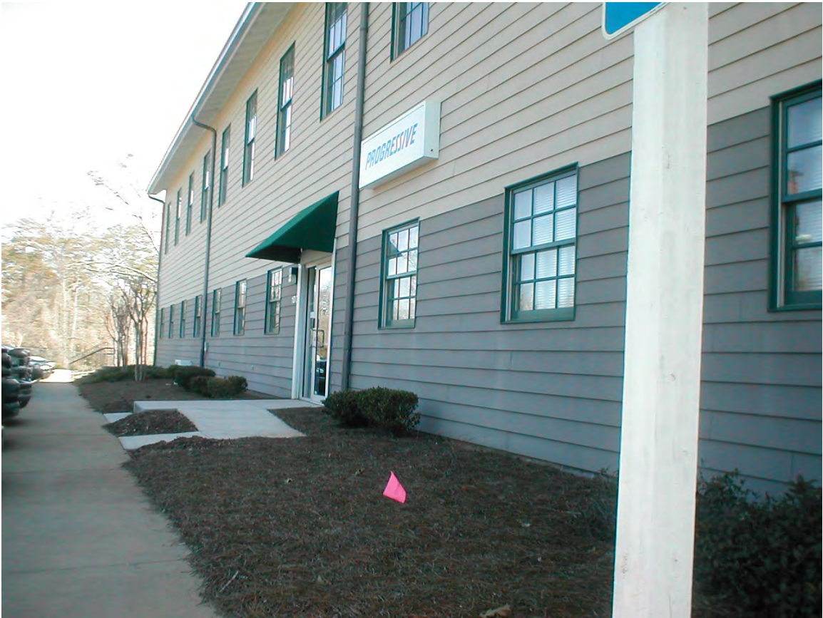
Plate 5: View – East. Shallow soil sample HA4 (1-2) (pink flag) was located near the southwest corner of the former Bibb Mill “Dye House”. March 6, 2008.
