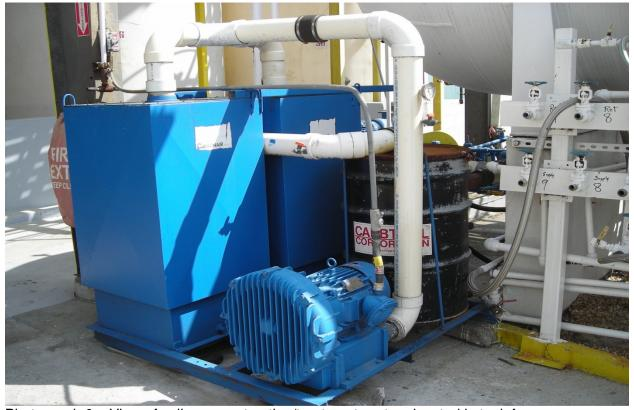
Photograph 6 – View of soil vapor extraction/treatment system located in tank farm area.
