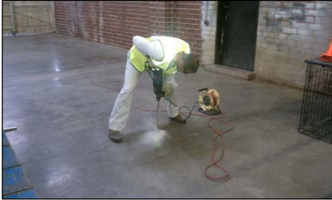
Photo 1 - Drilling through floor slab at BV051211-001; May 12, 2011
