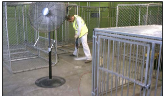
Photo 6 - Drilling through floor slab at BV051211-004; May 12, 2011
